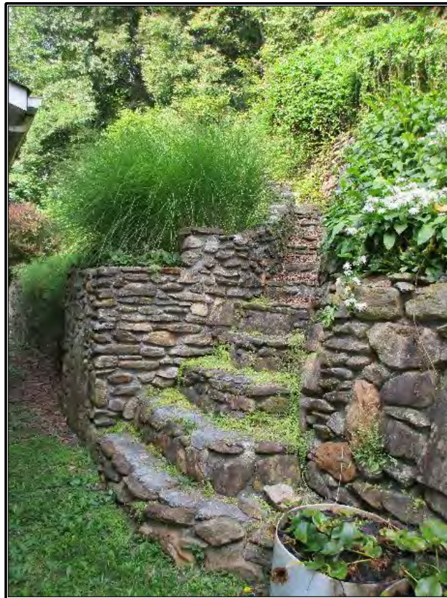
Figure 176. Stone stairs in the rear yard leading to a secondary terrace.
