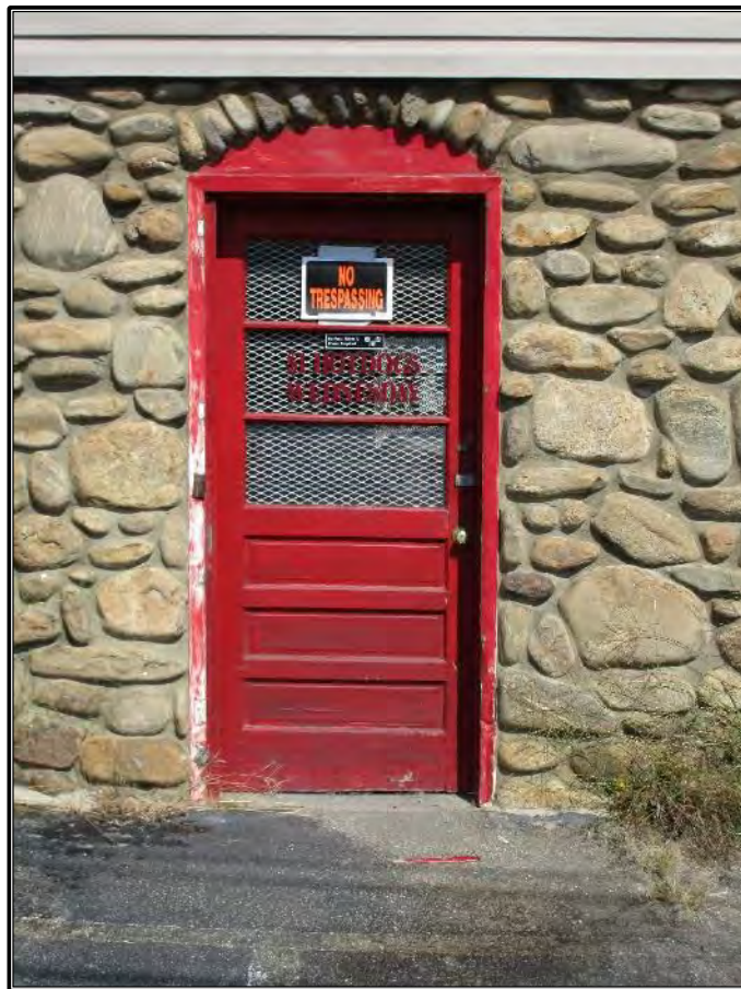
Figure 20. Detail of façade entry.
