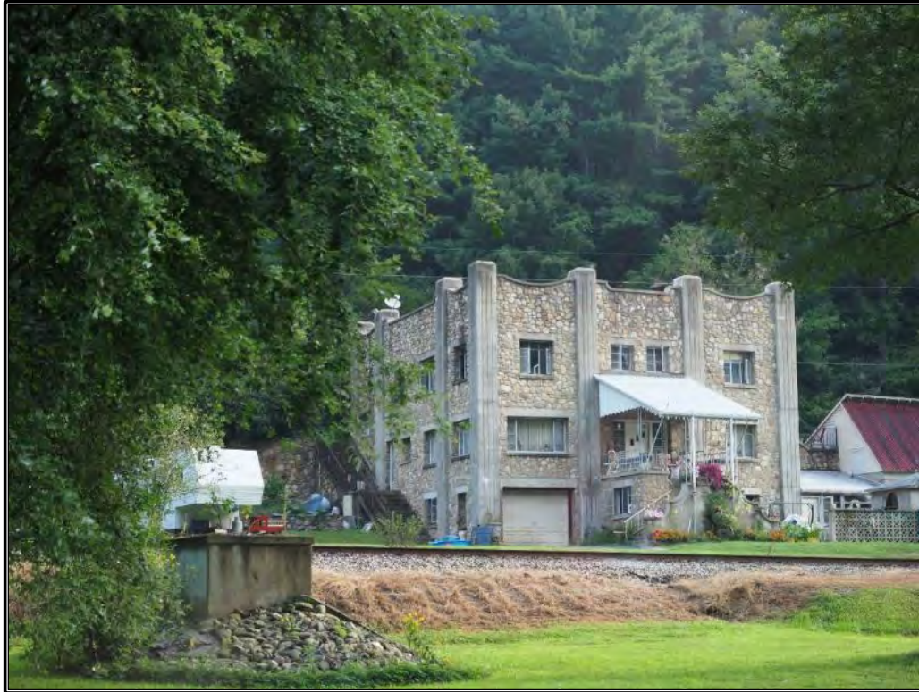
Figure 26. Rubble-rock masonry and cast-concrete commercial building along Asheville Highway east of Canton. This circa 1930–1950 building is among the largest and most intact examples encountered during the survey.
