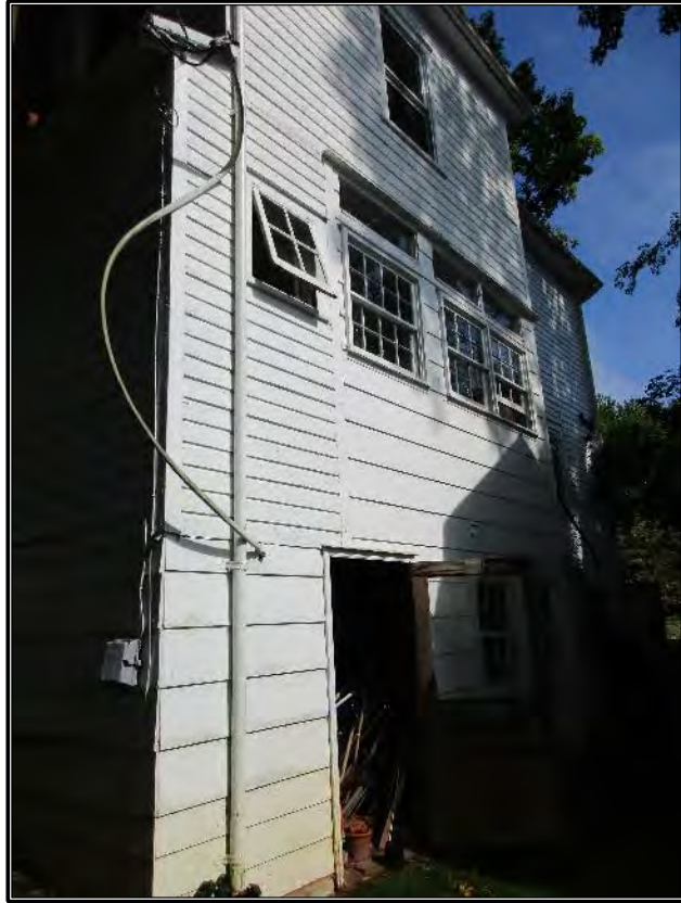
Figure 285. View of rear elevation.
