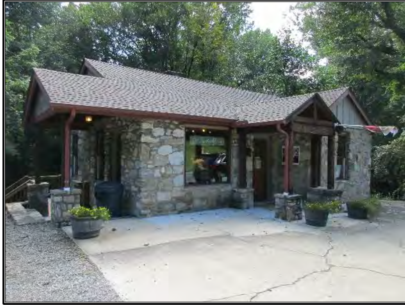
Figure 253. Façade of the Former House, 809 S. Main Street, now an artist studio.
