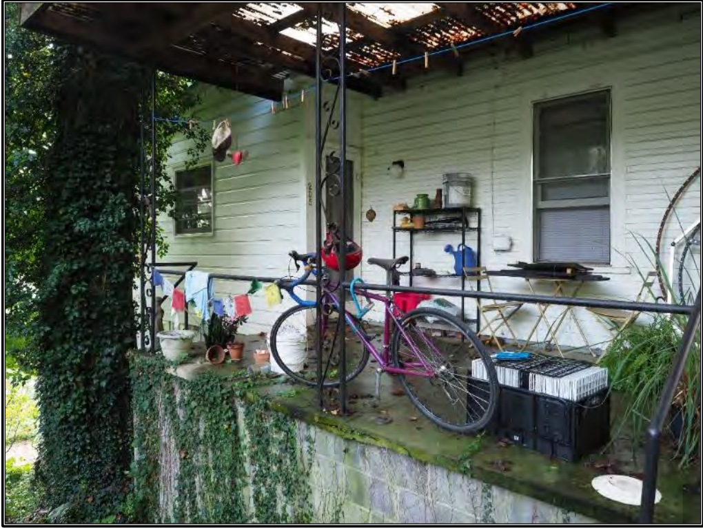
Figure 297. View of laundry building entrance and porch.
