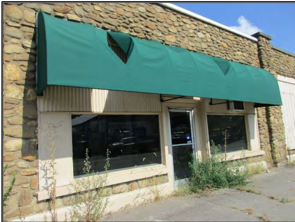
Figure 29. Detail of southwest façade storefront.
