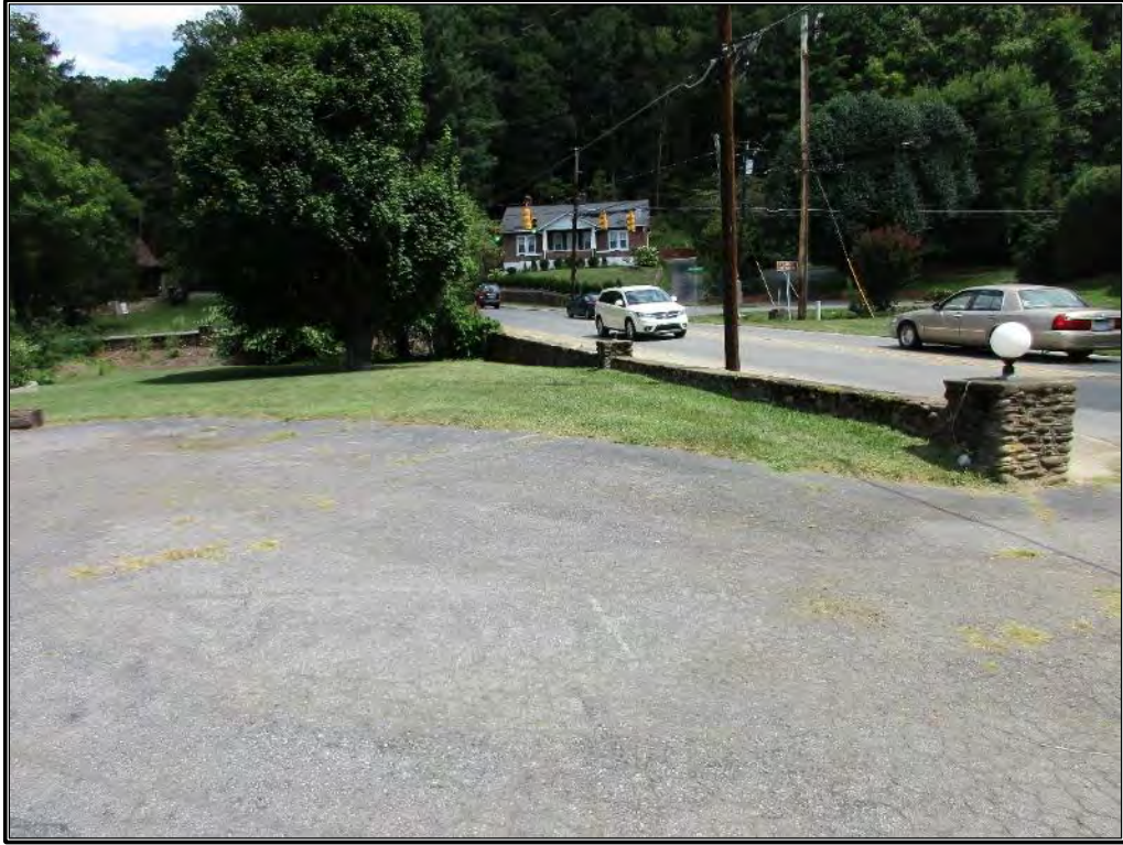
Figure 78. Overview of stone wall, looking west-southwest.
