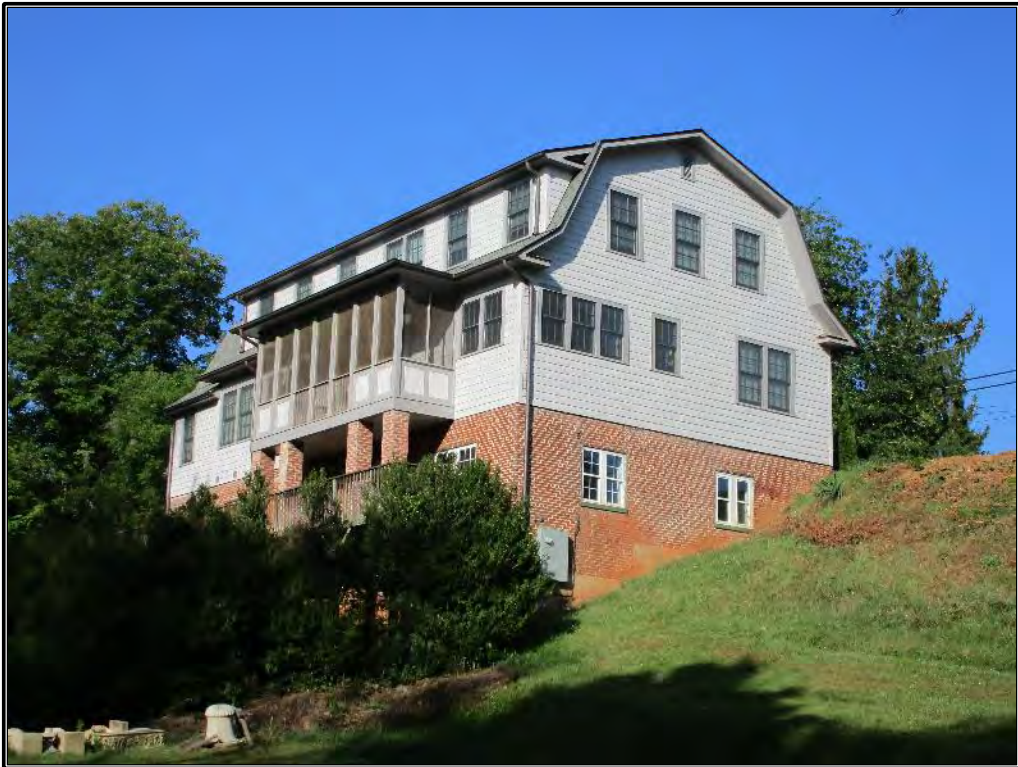
Figure 373. View of the northern corner with rear elevation and northeastern (side) elevation.
