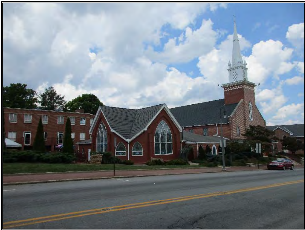
Figure 405. Overview of the First Baptist Church of Waynesville (HW0755) looking northwest.
