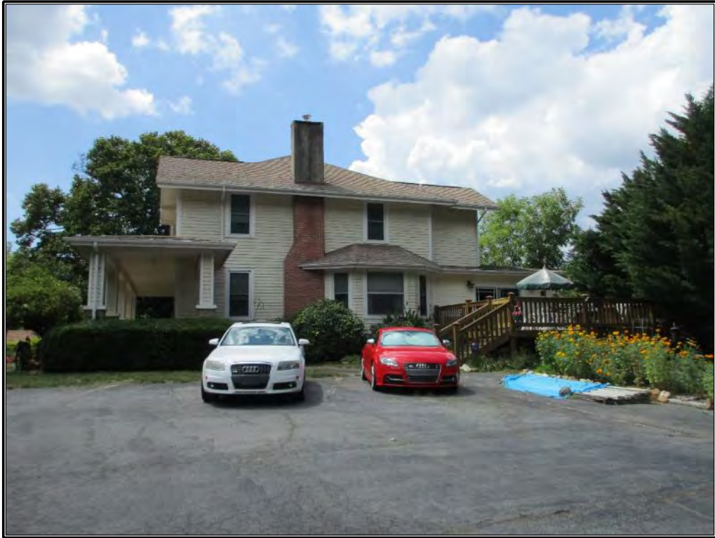
Figure 85. Northeast elevation of residence, looking west-southwest.
