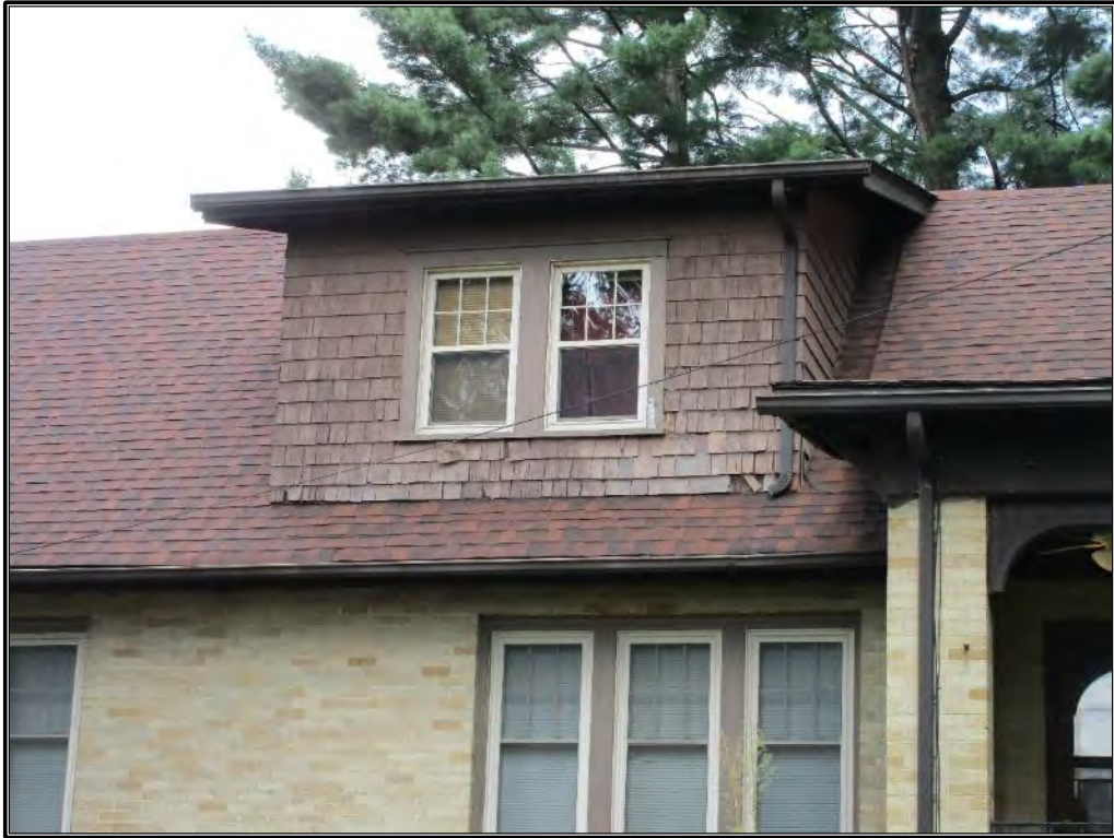
Figure 137. Detail of shed-roof dormer.
