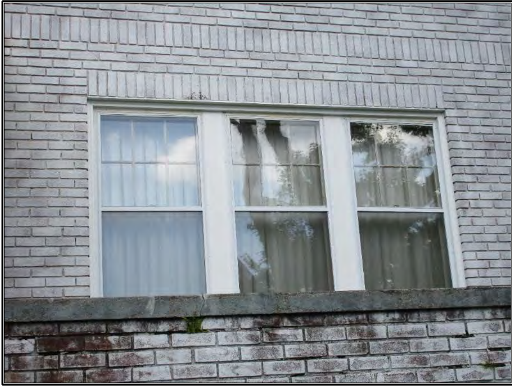
Figure 110. Detail of historic windows.
