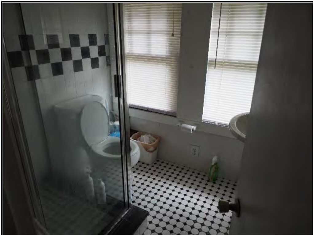
Figure 272. View of second floor bathroom.
