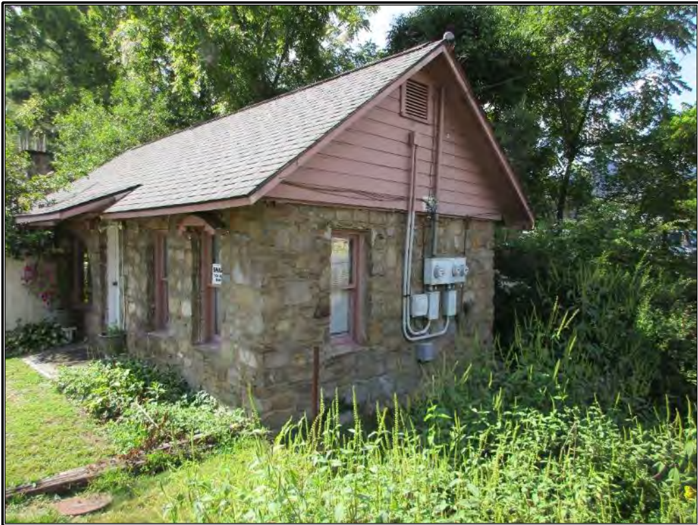
Figure 59. Northeast elevation of linear building, looking south.
