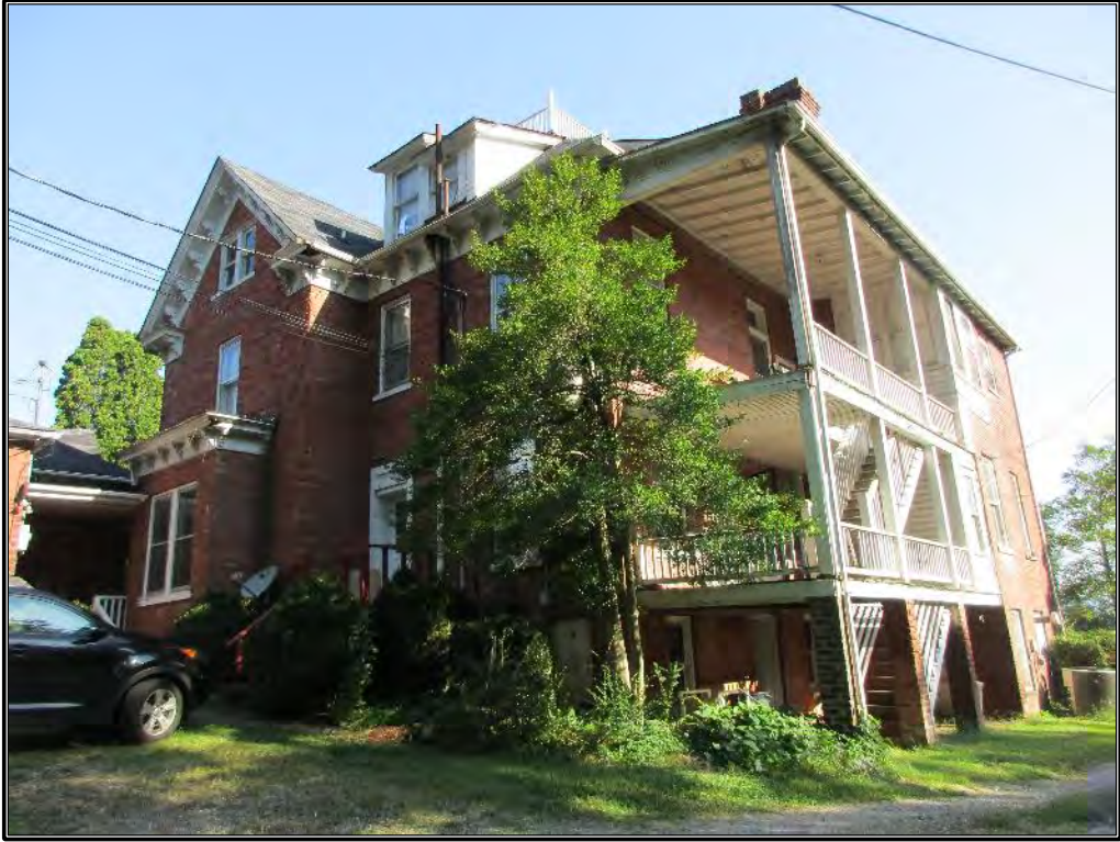
Figure 386. View of the southern corner with rear elevation.
