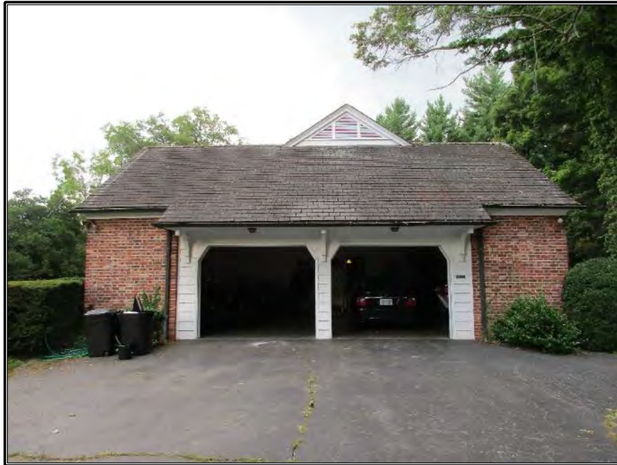
Figure 214. View of the north elevation showing the two-bay attached garage.
