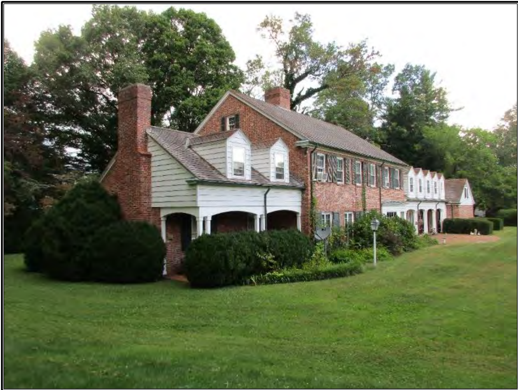
Figure 211. View of the east elevation of the southern wing.
