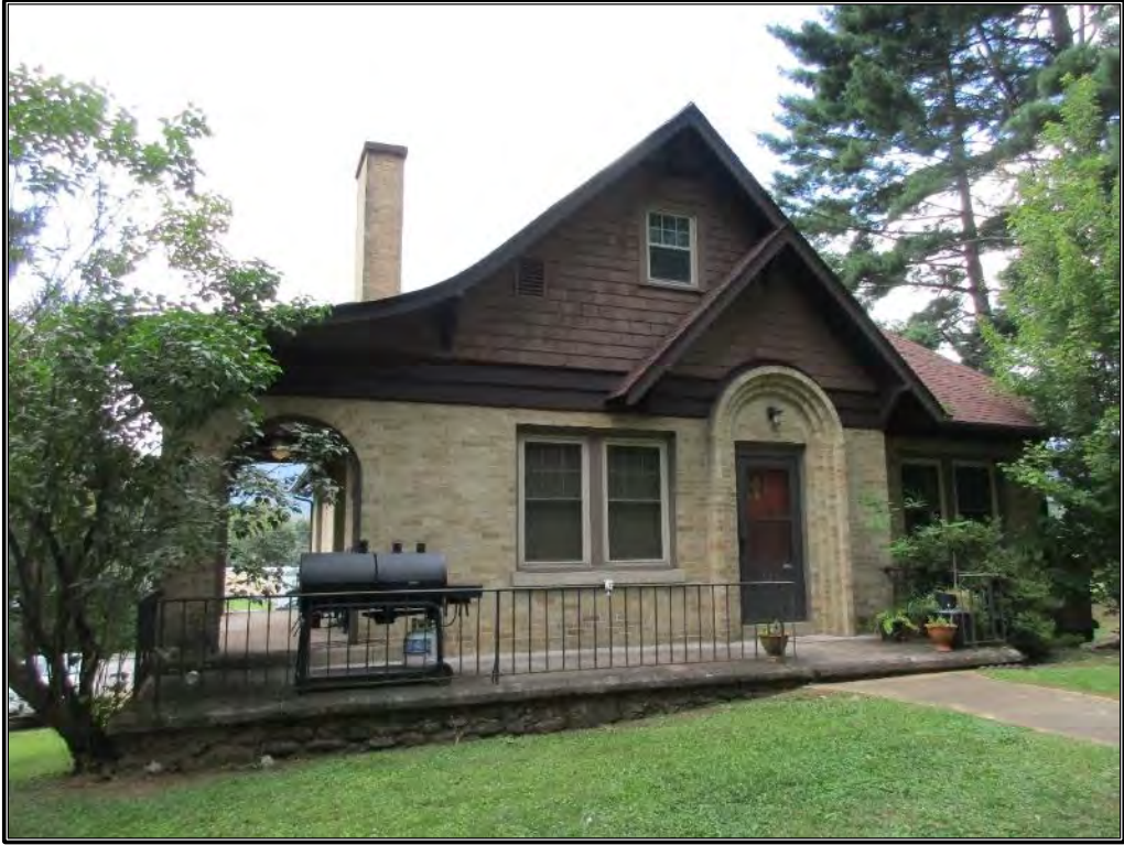
Figure 133. Façade of residence, looking west-northwest.
