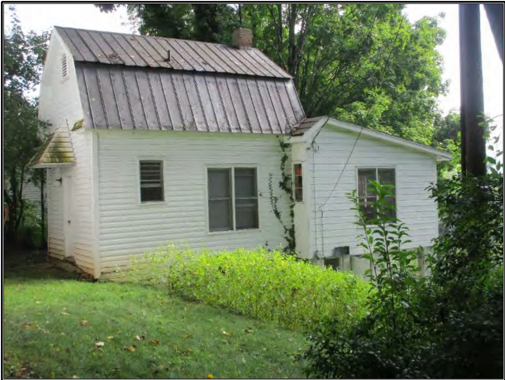
Figure 298. View of laundry looking northeast.
