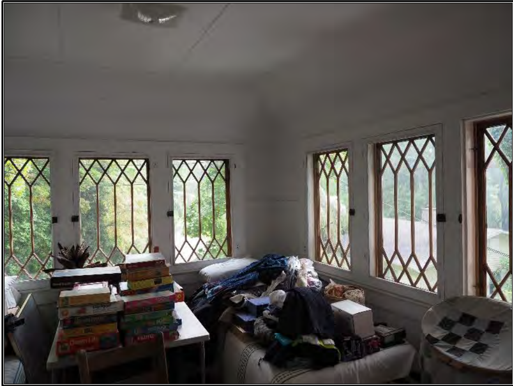
Figure 293. Interior view of porte cochere sleeping porch.
