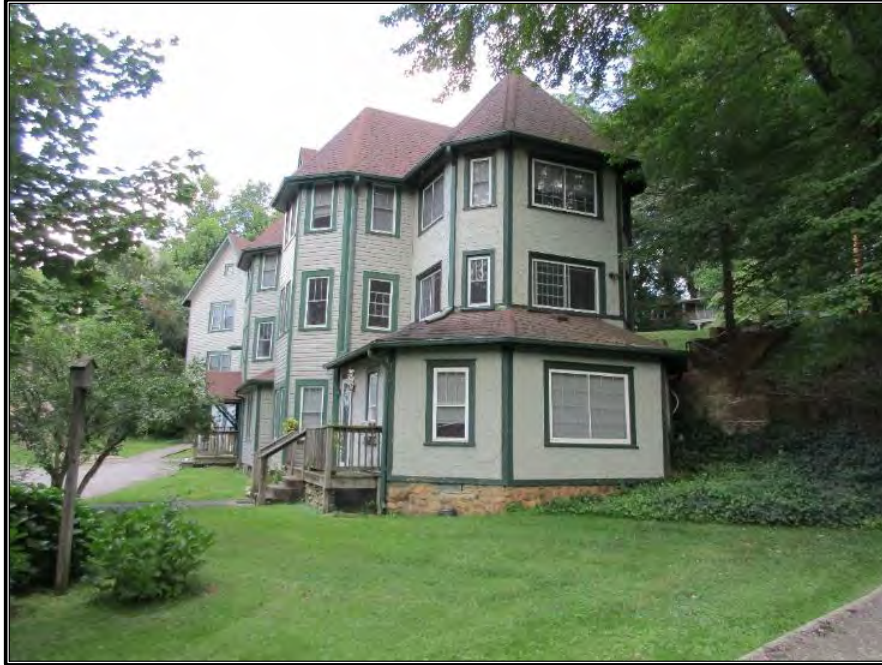
Figure 199. Southwest elevation showing the sloping lot.
