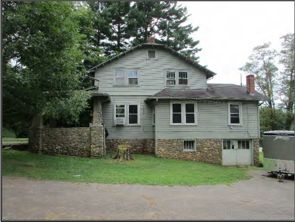
Figure 148. Northeast elevation of residence, looking south-southwest.
