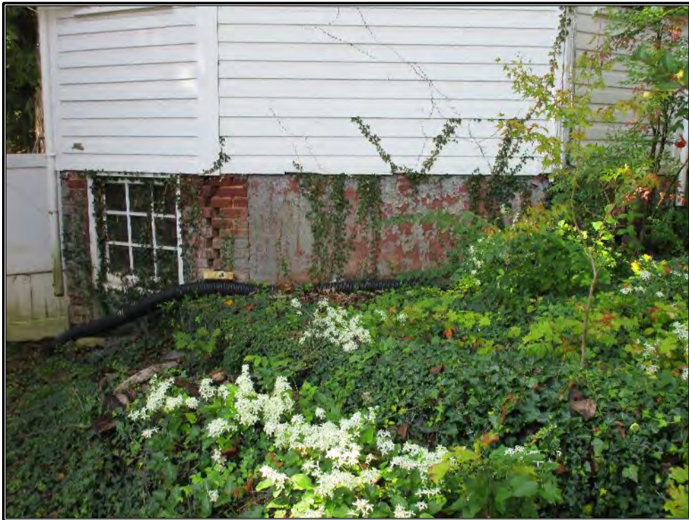
Figure 286. View of basement foundation and window.
