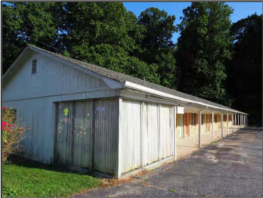
Figure 367. View of now-abandoned motel on Soco Road in Maggie Valley with corner office enclosed with plate glass.
