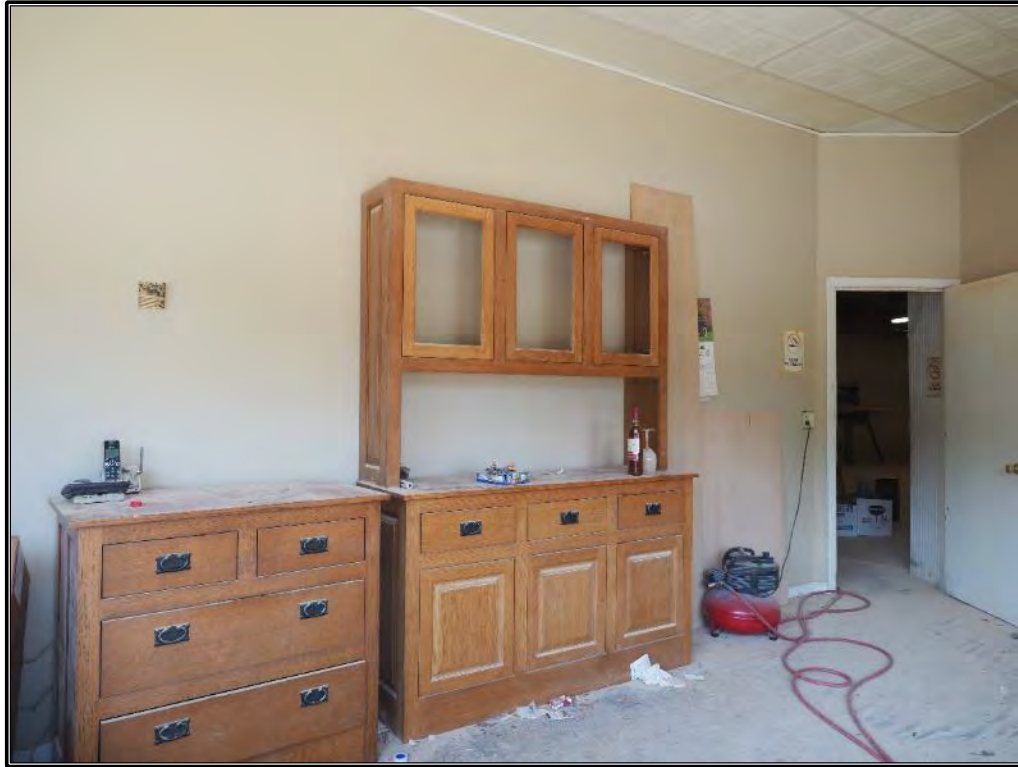
Figure 38. Interior view of storefront along the northeast elevation.
