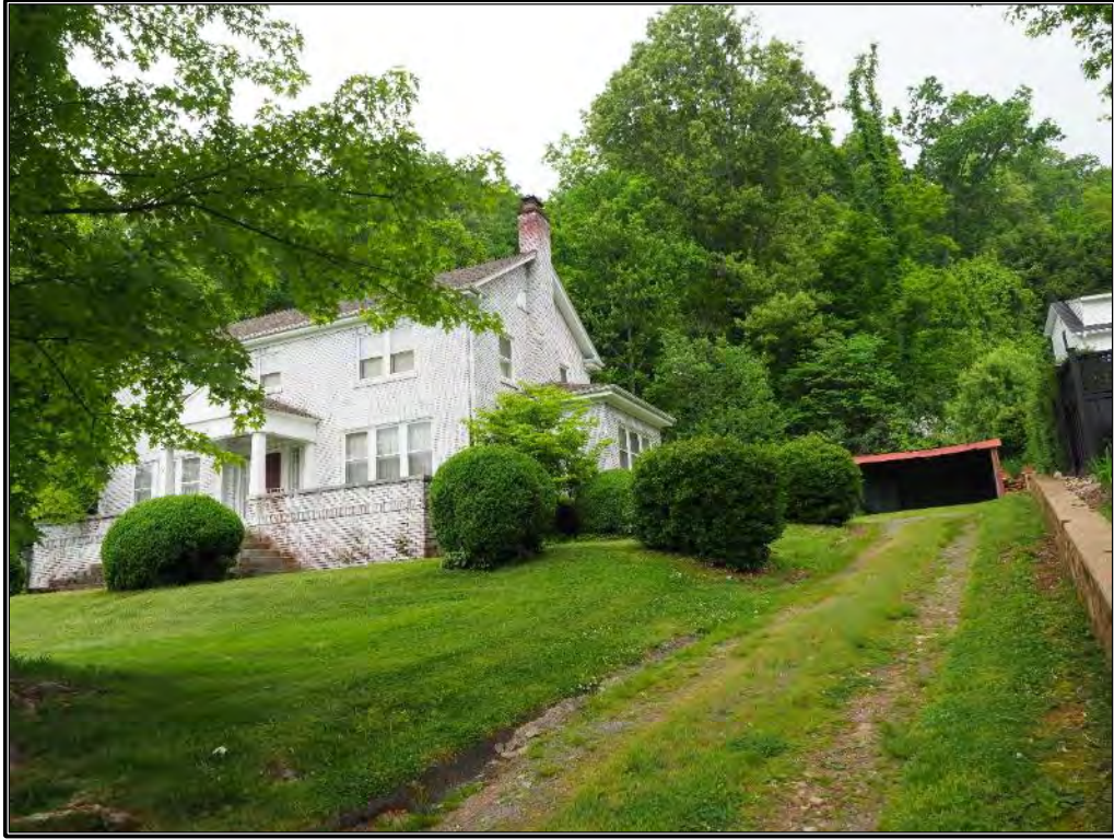
Figure 106. View of driveway from Virginia Avenue, looking east.
