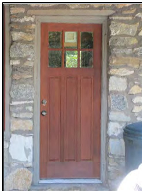
Figure 255. Detail of front entry door.
