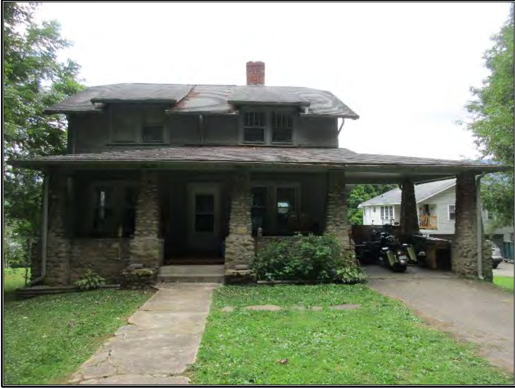
Figure 144. Façade of residence, looking west-northwest.
