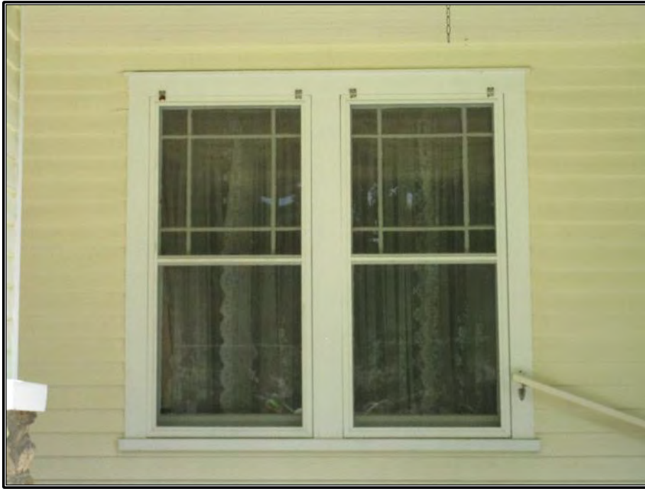
Figure 82. Detail of historic windows.
