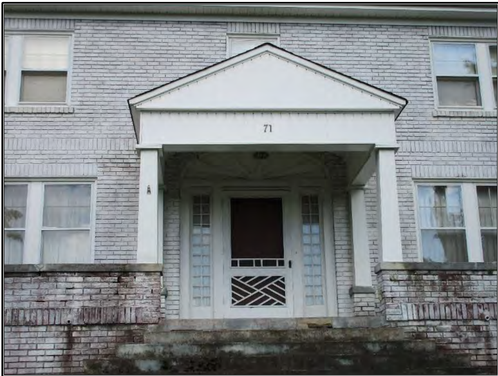
Figure 111. Detail of façade entry.
