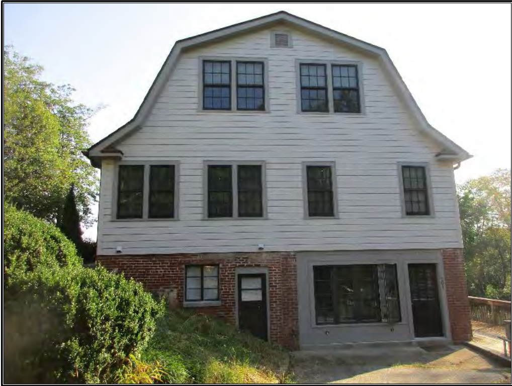
Figure 372. View of southwestern elevation with enclosed garage entry.
