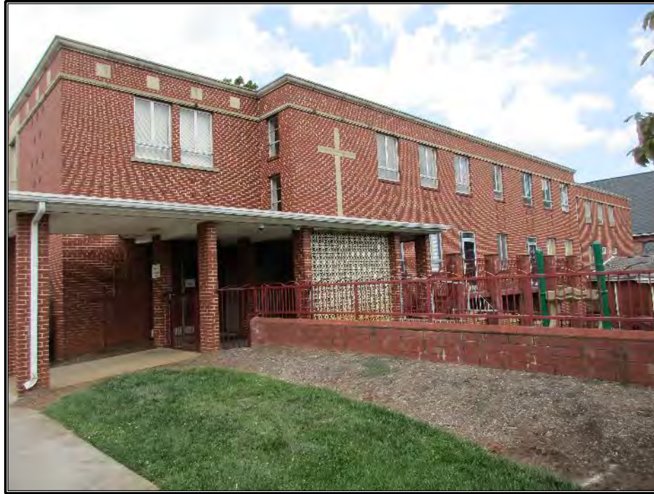
Figure 418. Façade view of the Child Development Center.
