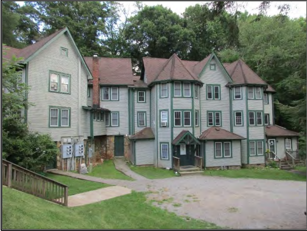
Figure 195. Northwest elevation with entrances and parking area.
