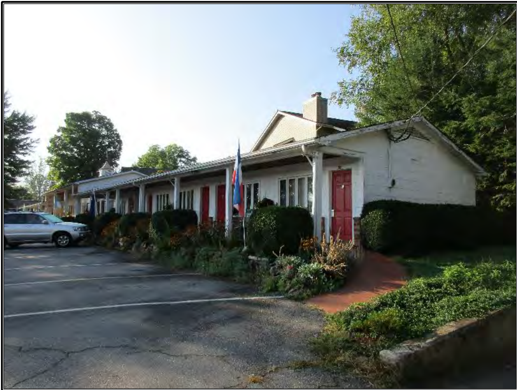
Figure 350. Northwestern corner view of Building A with asbestos shingle siding.
