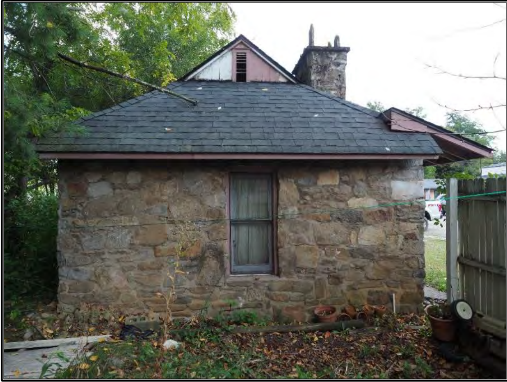
Figure 60. Southwest elevation of linear building, looking northwest.
