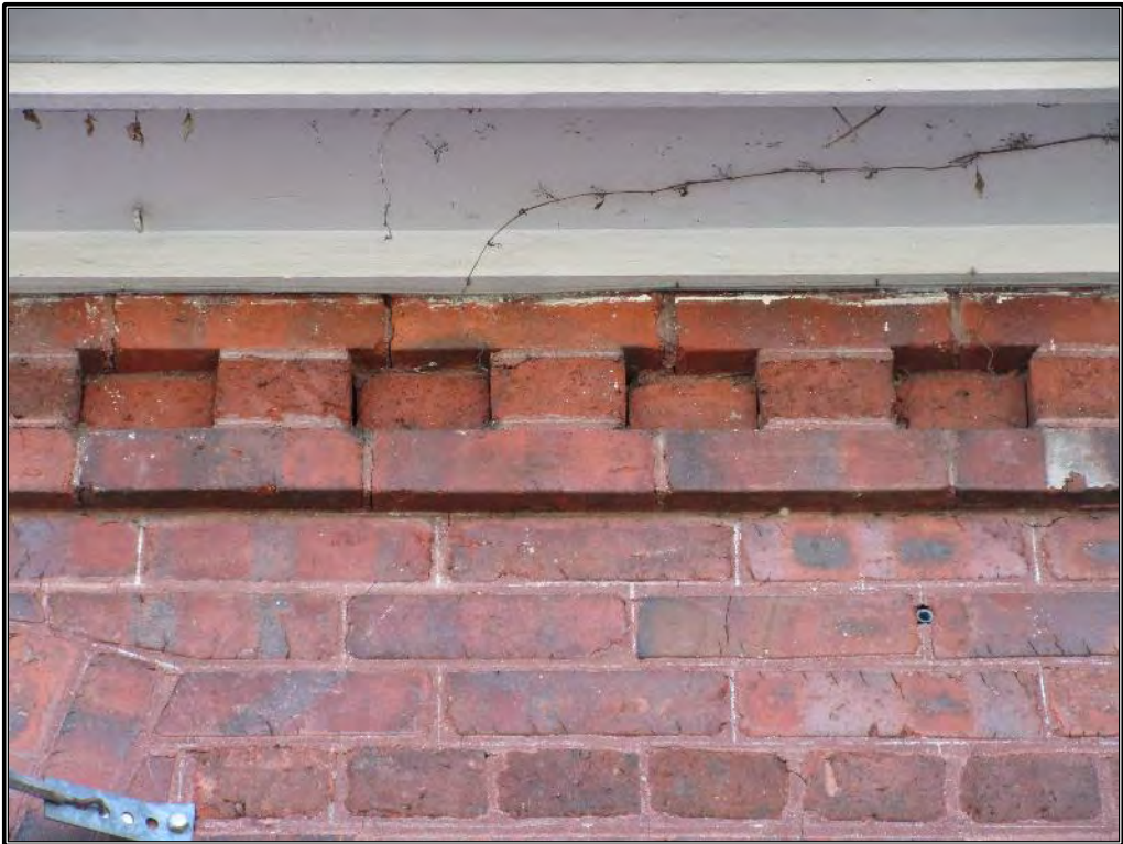
Figure 393. Detail of the brick cornice.
