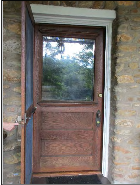
Figure 246. Detail of historic door and screen door.
