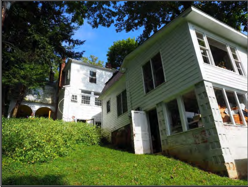
Figure 299. View of southeastern corner of the laundry building.
