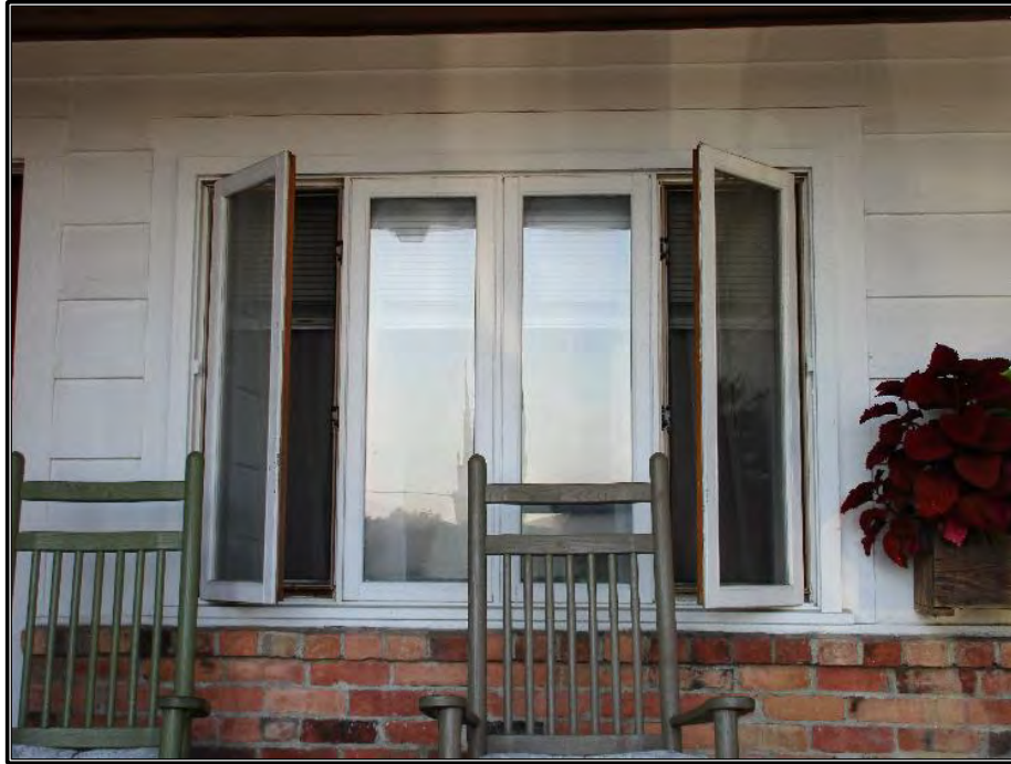
Figure 351. Detail of unit window.
