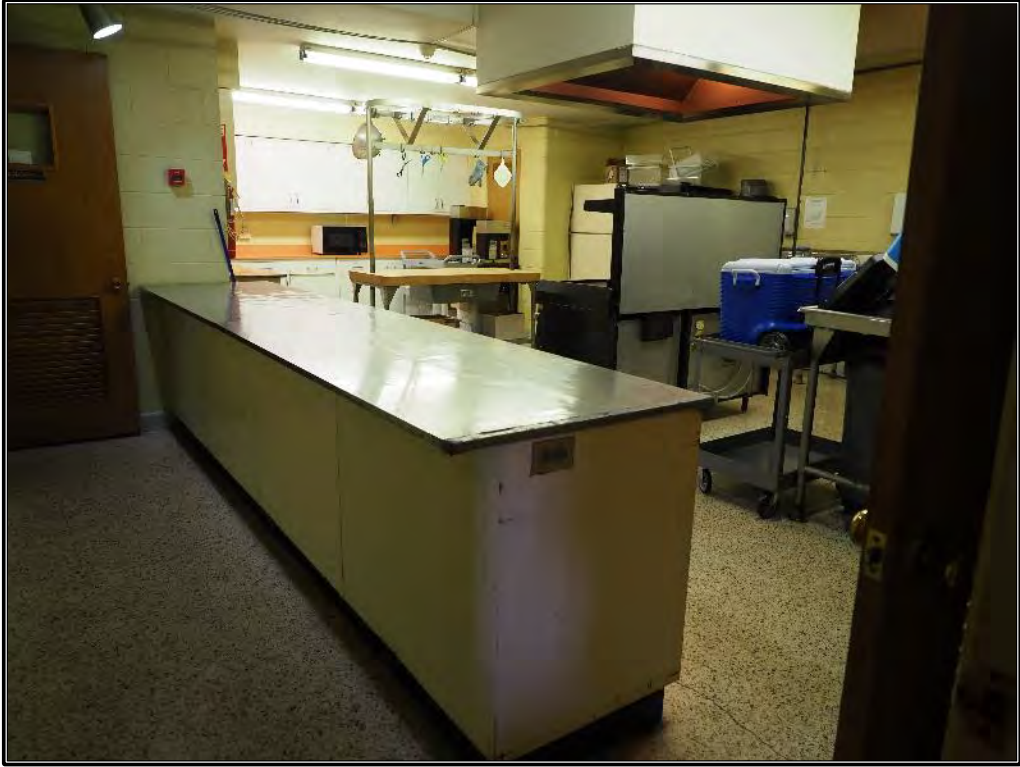
Figure 416. Commercial kitchen in the office annex.
