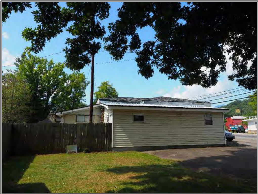
Figure 70. Northeast elevation of commercial building, looking west-southwest.
