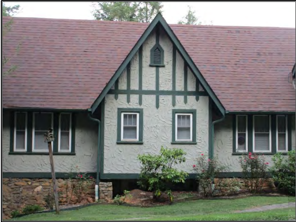
Figure 197. Detail of gable with faux half timbering.
