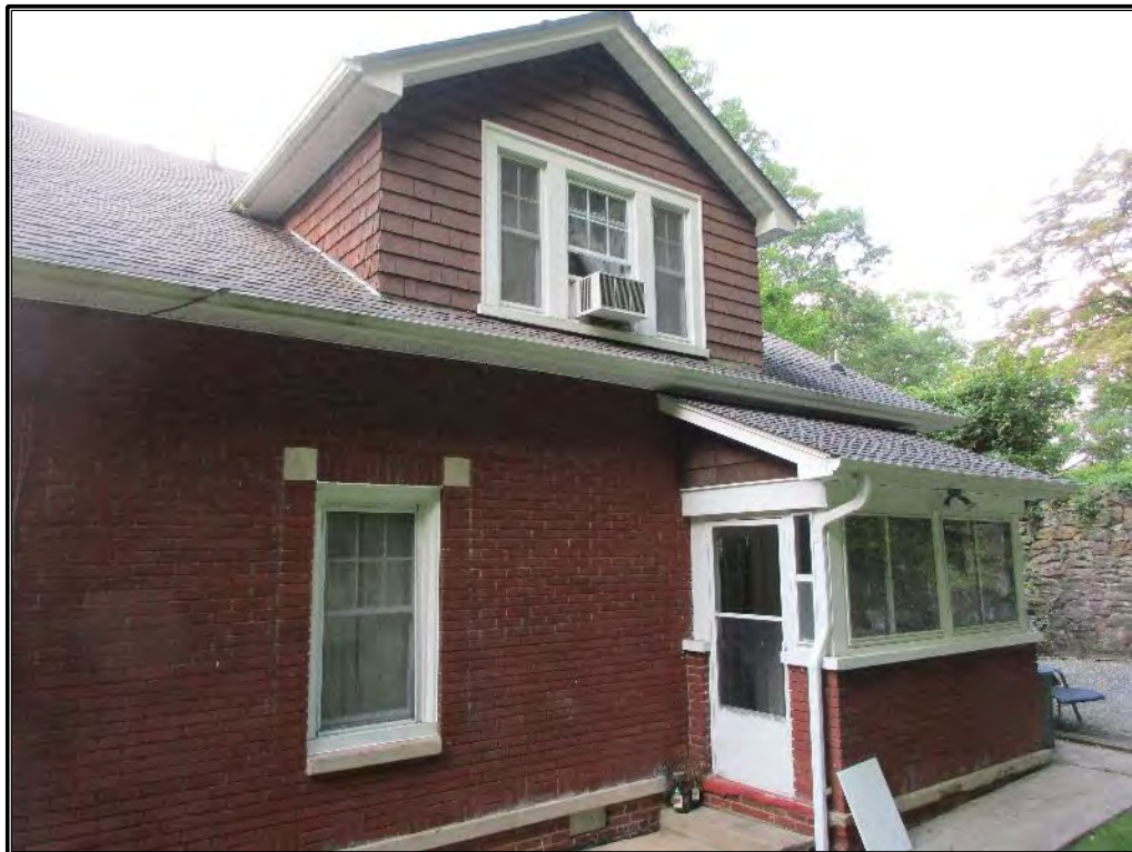
Figure 167. Rear elevation with dormer and porch.
