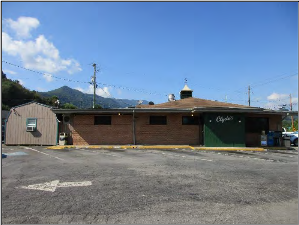
Figure 6. Northeast elevation of restaurant, looking southwest.
