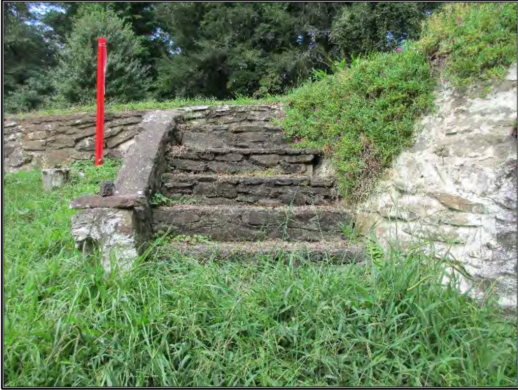
Figure 264. Stairs leading from South Main Street to side and rear yards.
