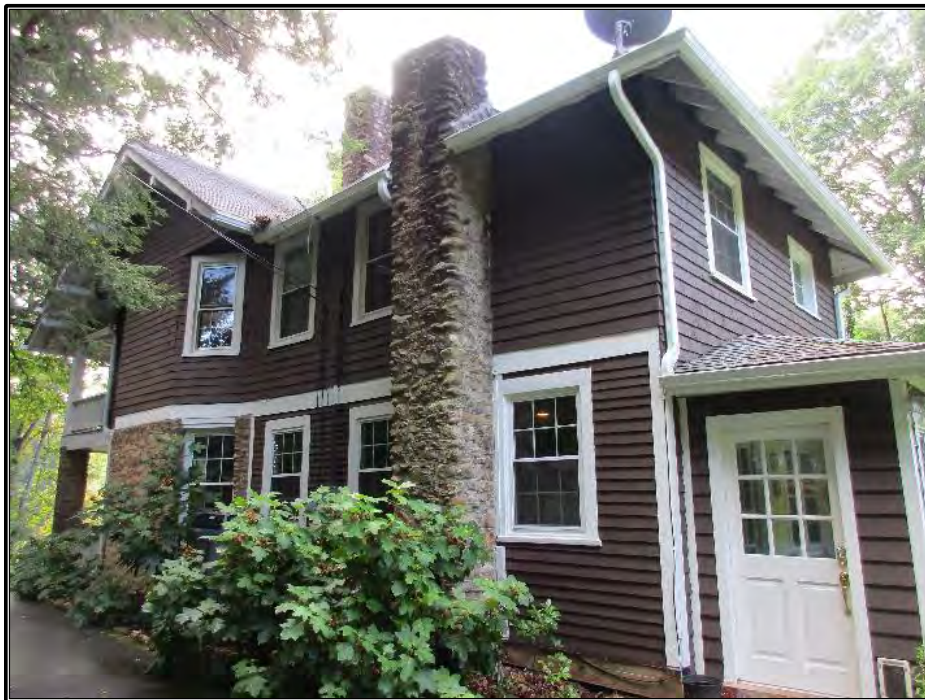
Figure 245. View of northeast (side) elevation.
