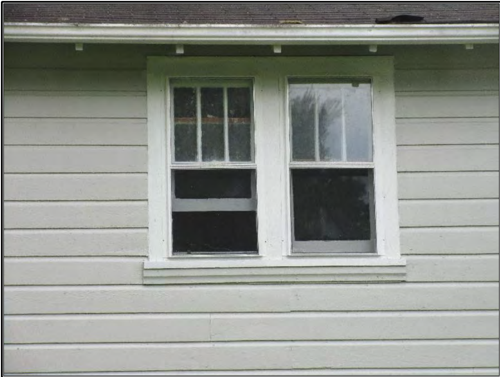
Figure 152. Detail of historic windows.
