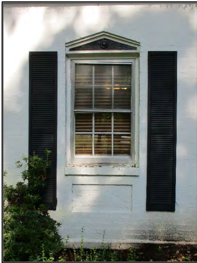
Figure 307. Detail of window with pediment on the façade.
