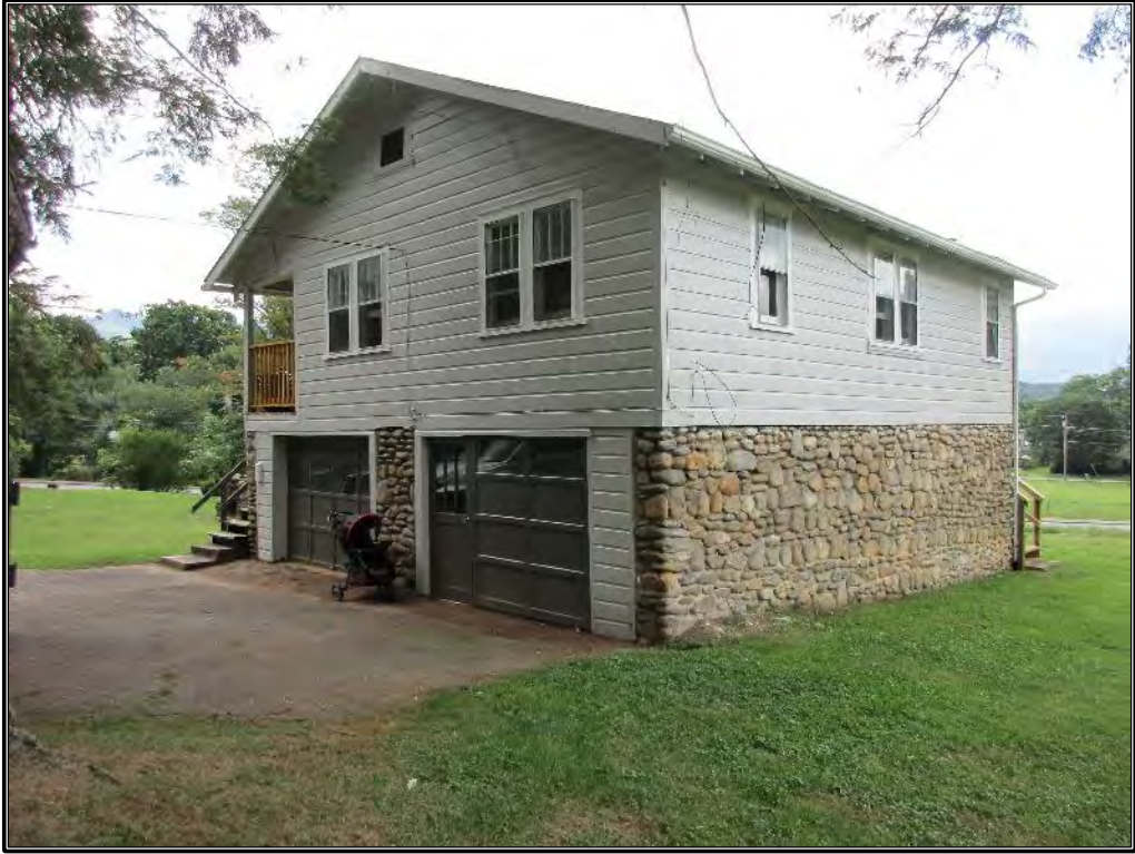
Figure 153. East and rear elevation of carriage house, looking west-southwest.
