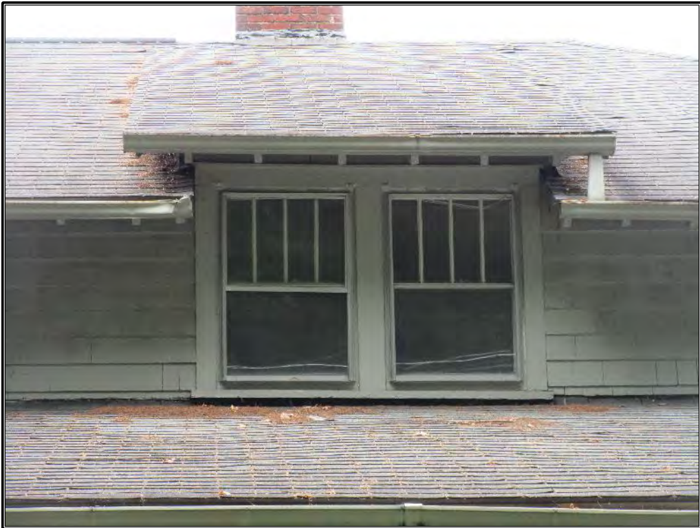
Figure 145. Detail of historic windows and wall dormer.
