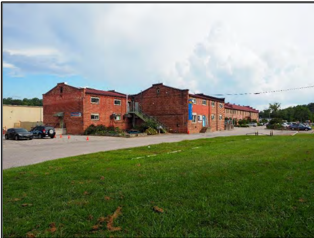
Figure 52. Overview of former industrial buildings along Lyman Street in Asheville showing regionally typical warehouse development, now a renovated arts district.
