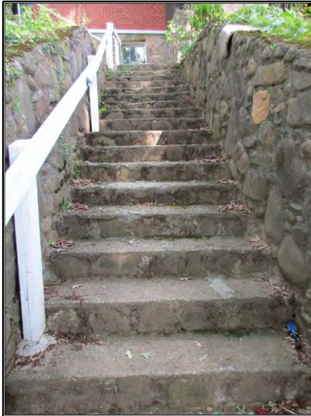
Figure 188. Stone and concrete stairs leading up the steeply sloping lot to the residence.
