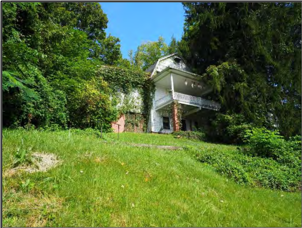
Figure 302. Rear view of carriage house (HW0751).
