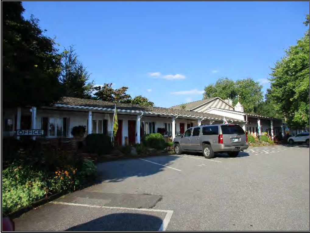
Figure 349. Overview of Building A, looking west-southwest.
