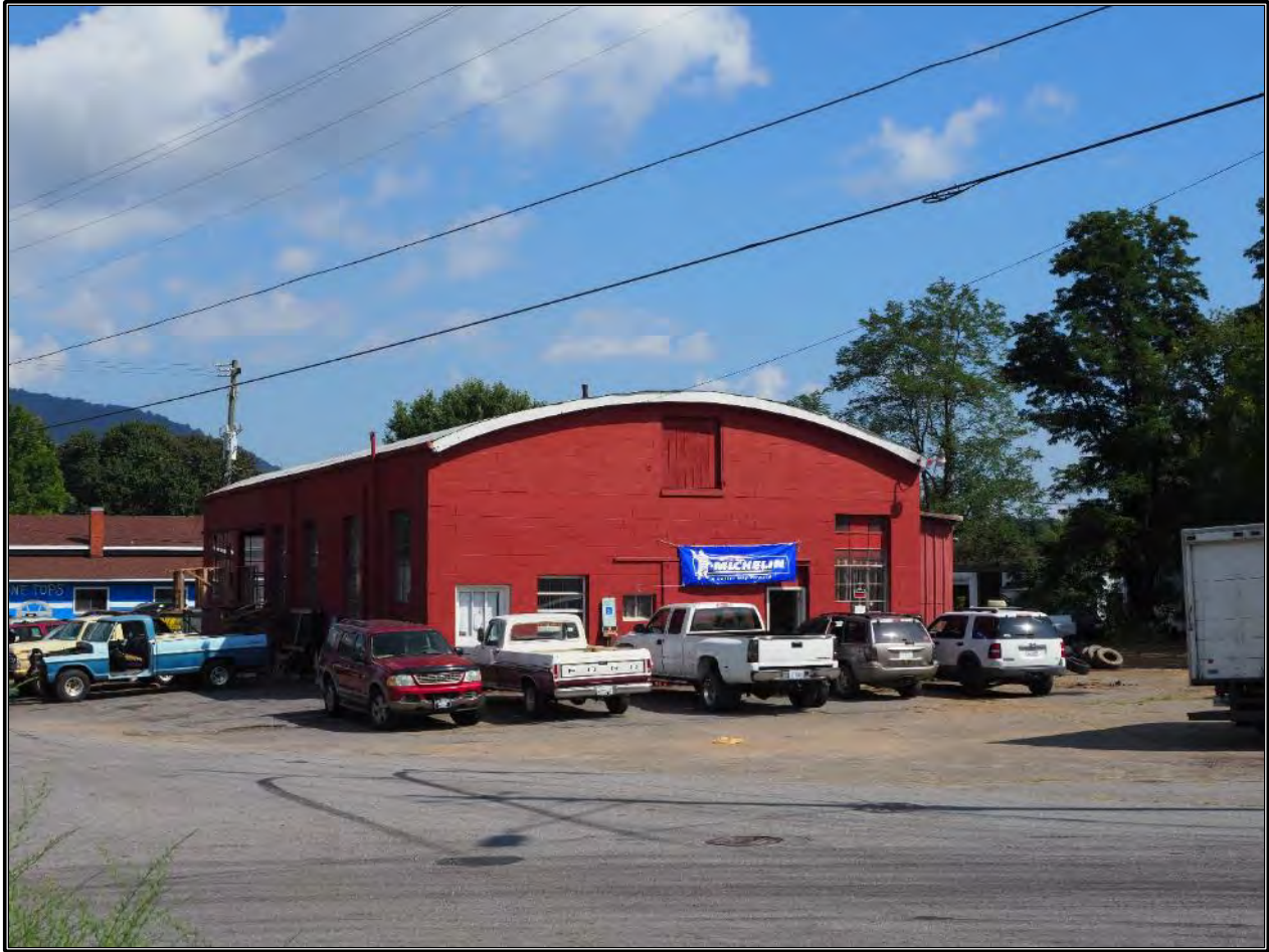
Figure 45. Façade and west elevation of repair shop, looking north-northeast.
