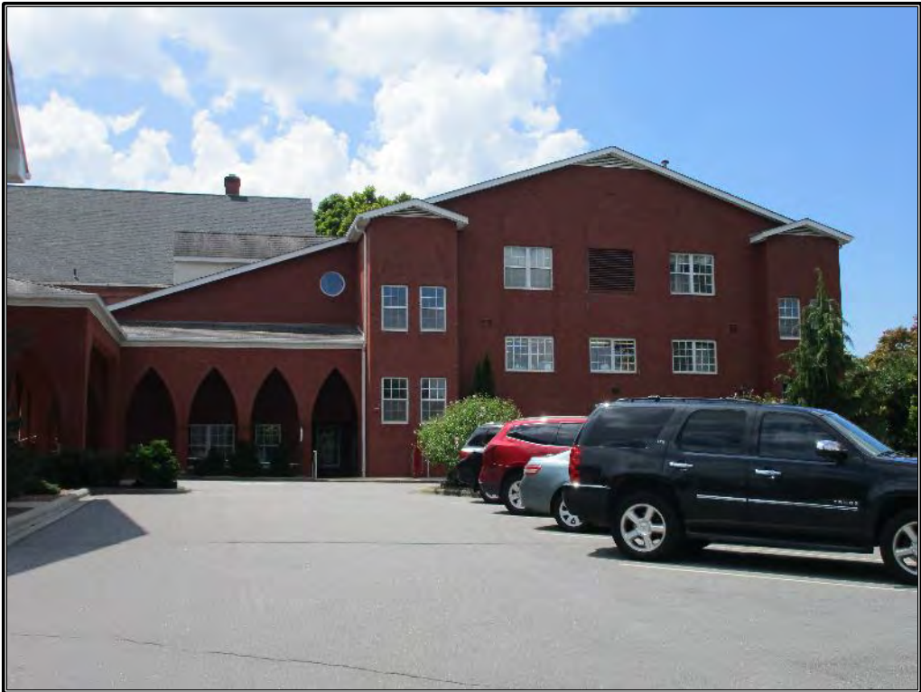
Figure 410. Northern elevation of the office annex.
