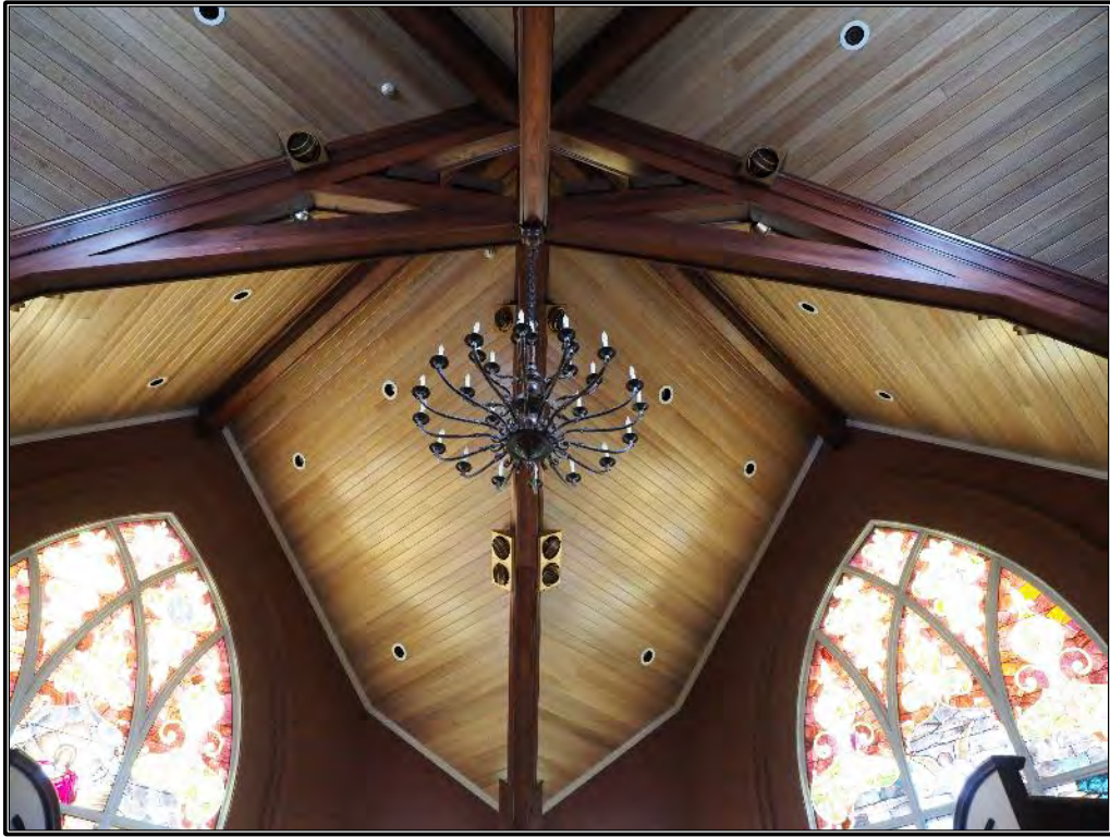
Figure 414. View of the new sanctuary ceiling.
