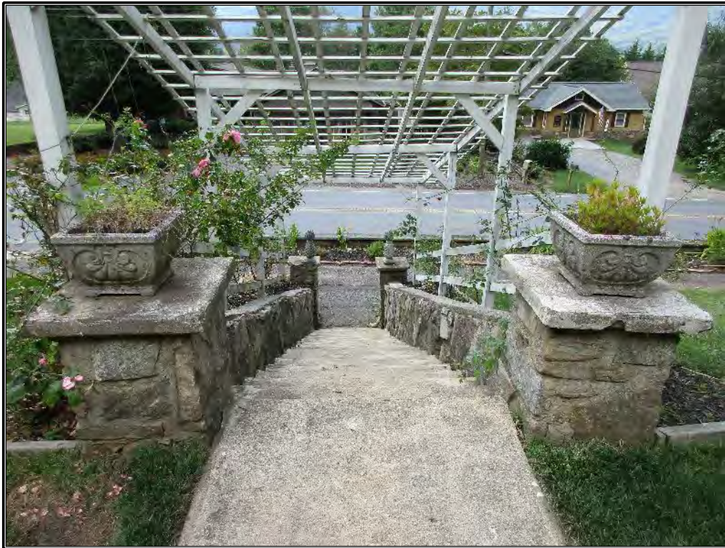
Figure 162. View of concrete steps, stone walls, and pergola.
