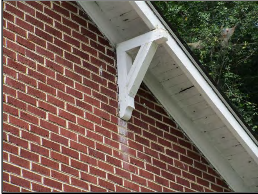
Figure 121. Detail of brackets and rafters.
