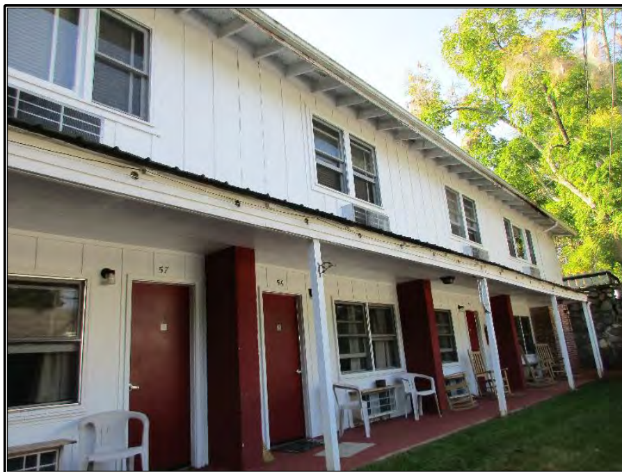
Figure 358. View the rear elevation of Building B.
