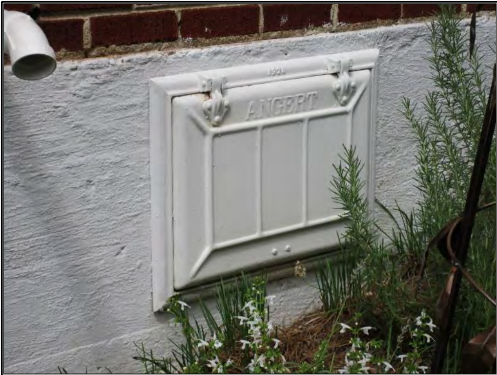
Figure 125. Detail of coal chute.
