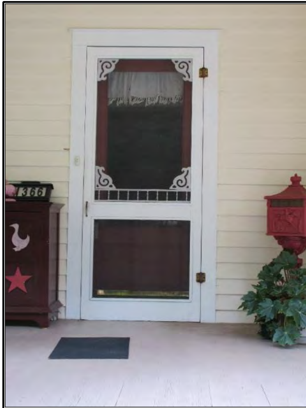
Figure 83. Detail of front entry.
