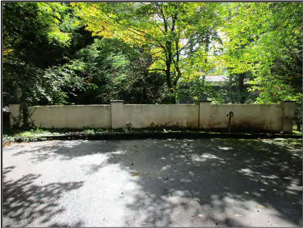
Figure 224. Stucco wall along Grimball Drive.
