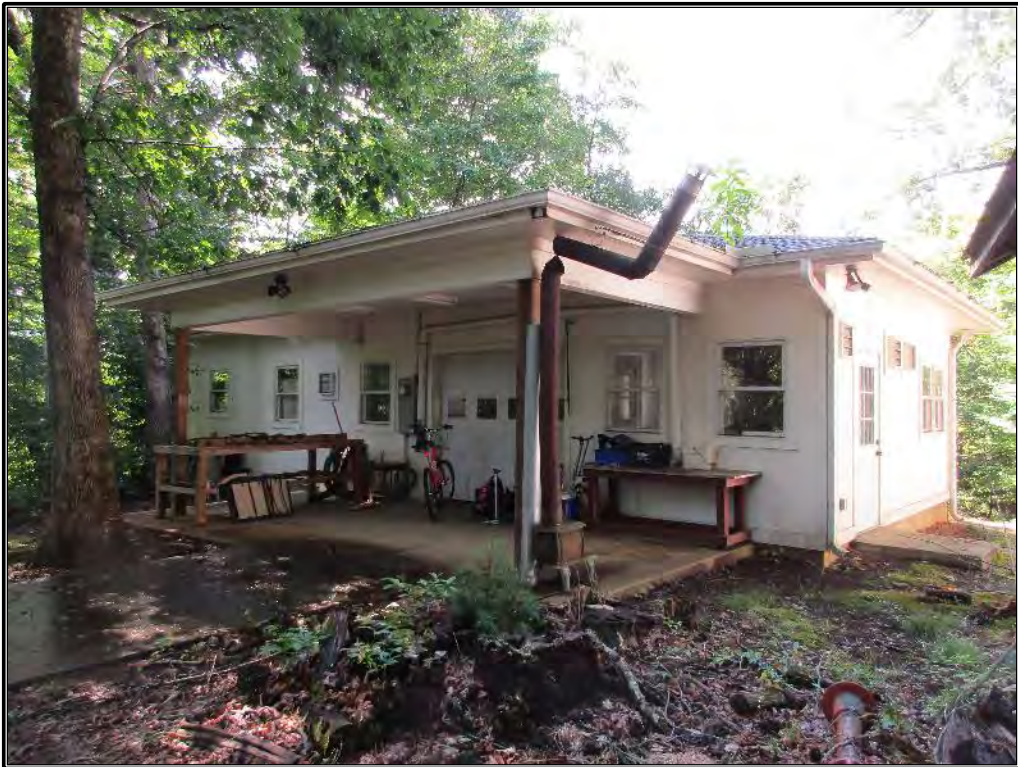
Figure 236. Rear elevation of the workshop.
