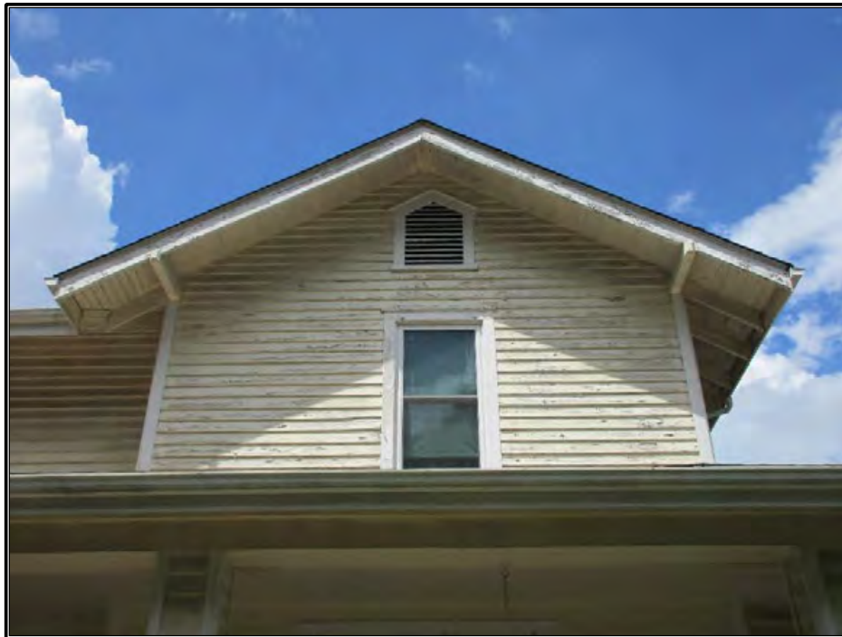
Figure 84. Detail of façade projection.
