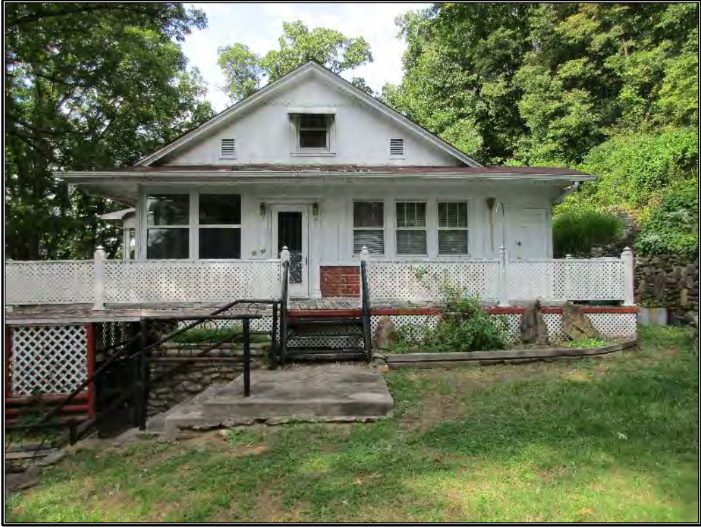
Figure 179. Southern elevation with concrete steps.
