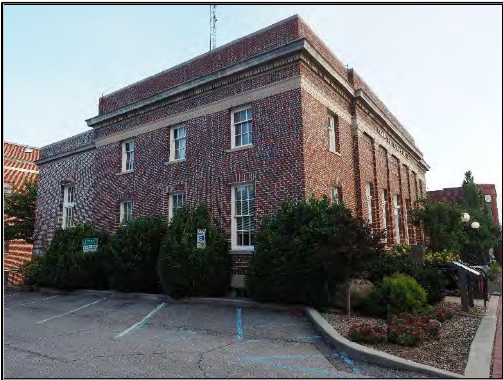
Figure 425. View of 16 South Main Street.
