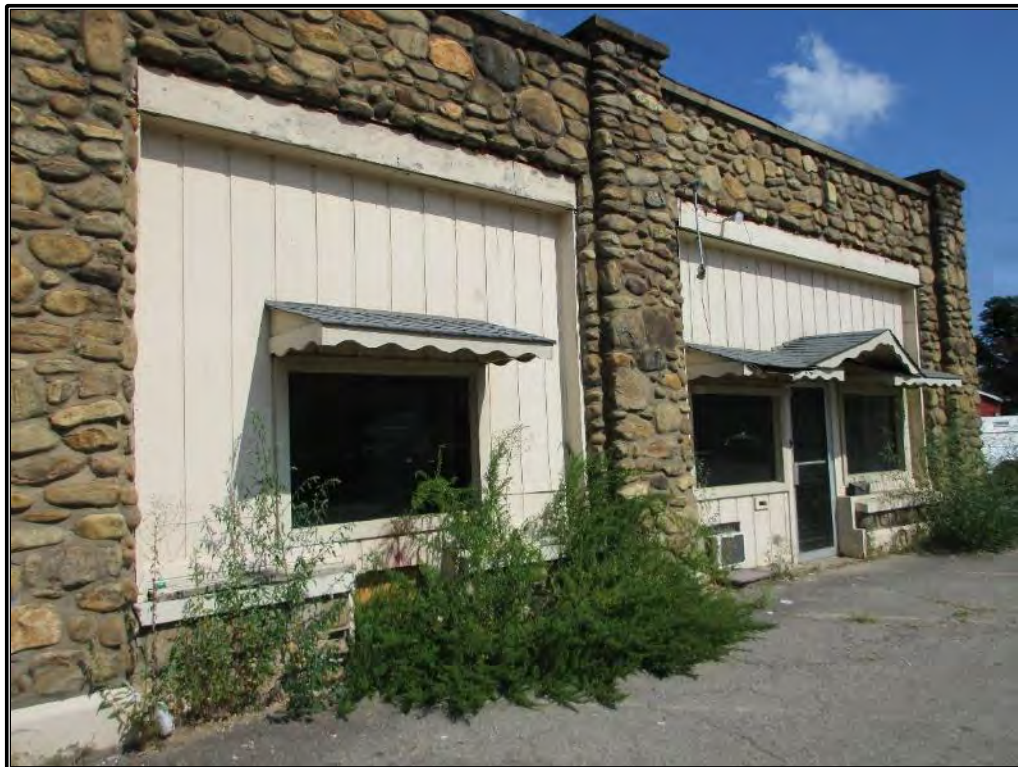
Figure 31. Detail of northeast façade storefront.
