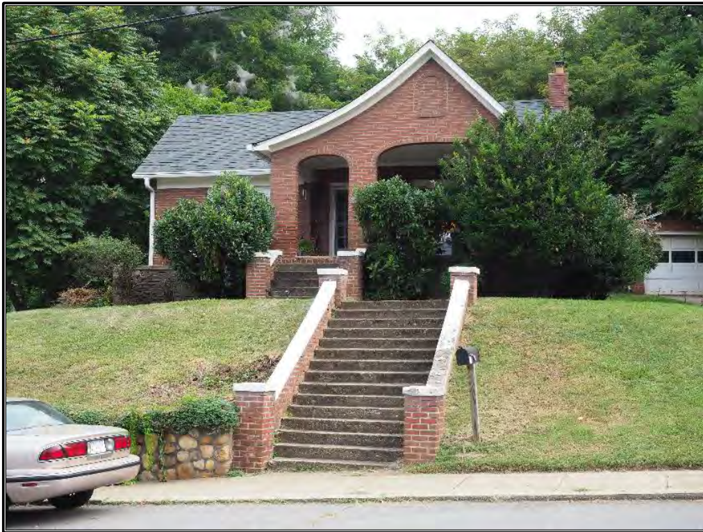
Figure 141. Residence at 75 Academy Street, Canton.
