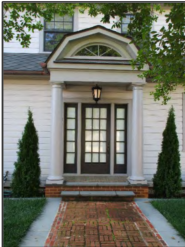
Figure 371. View of entry door and porch.
