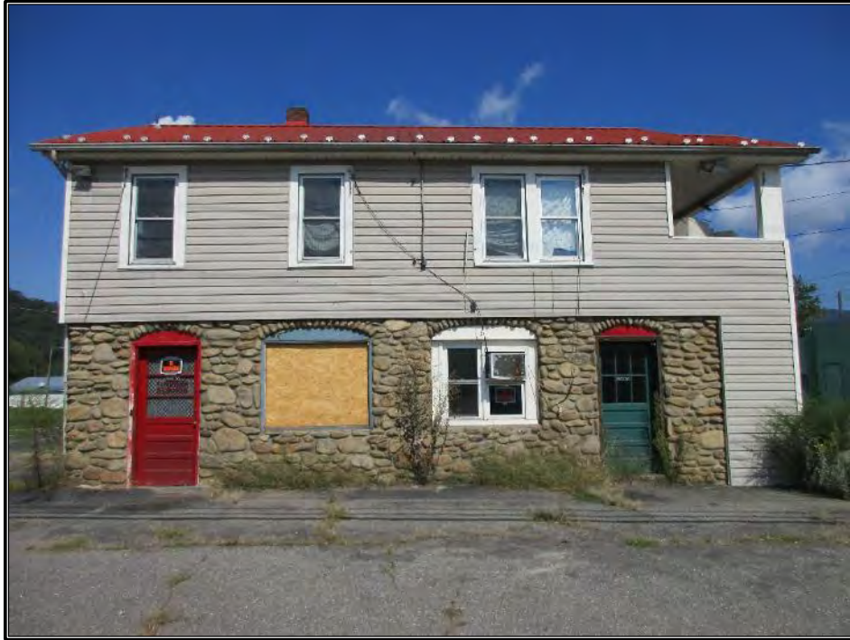
Figure 17. Façade of commercial building, looking northwest.
