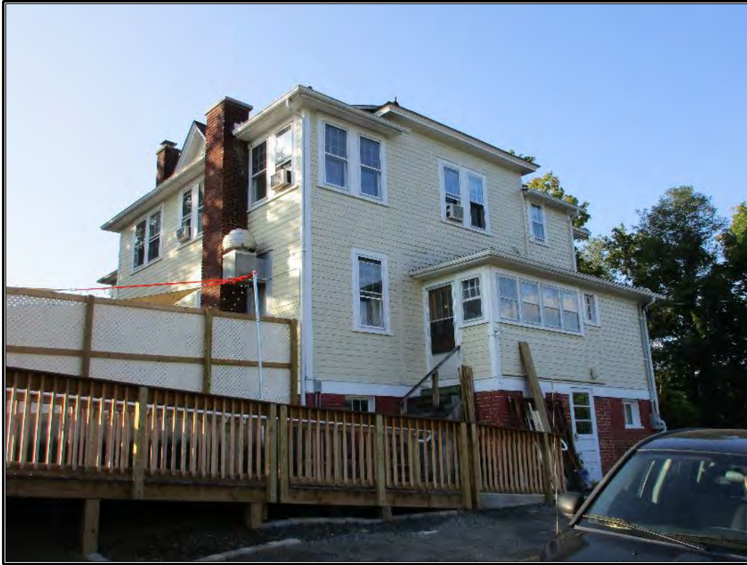
Figure 332. View of the rear elevation.
