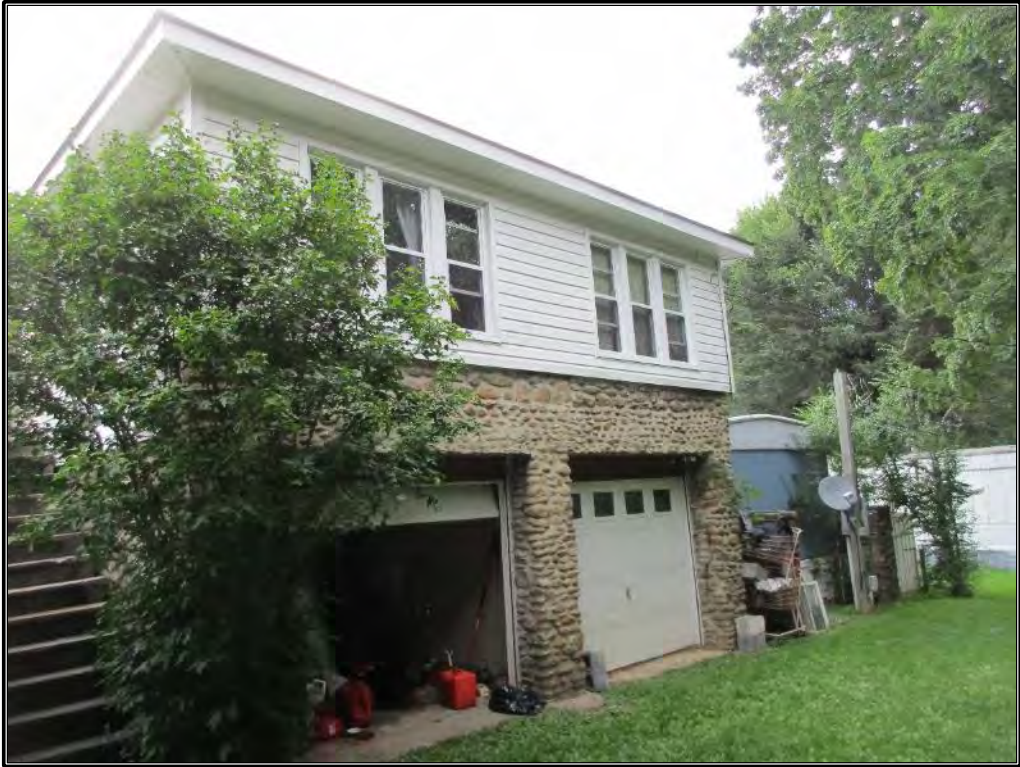
Figure 100. Southeast elevation of converted carriage house, looking east.
