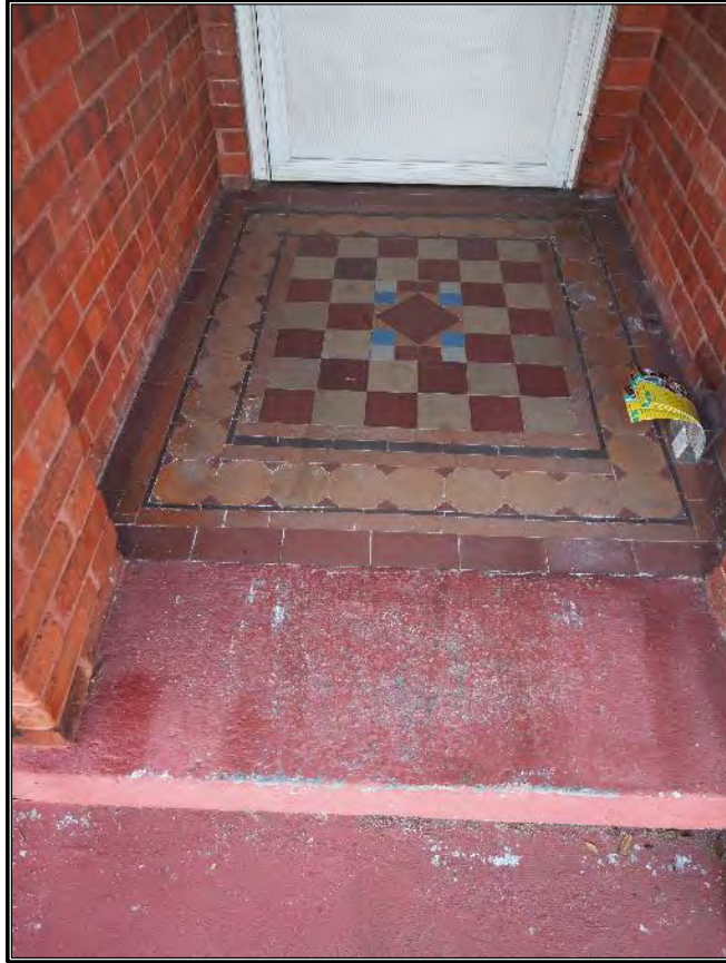
Figure 394. Detail of entry with painted brick.
