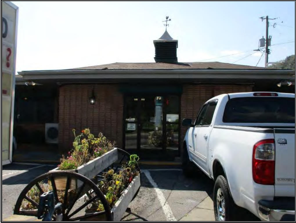
Figure 5. Detail of entry vestibule, looking south-southeast.
