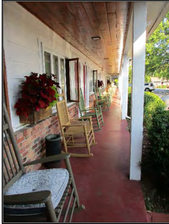
Figure 352. Overview of porch on Building A.
