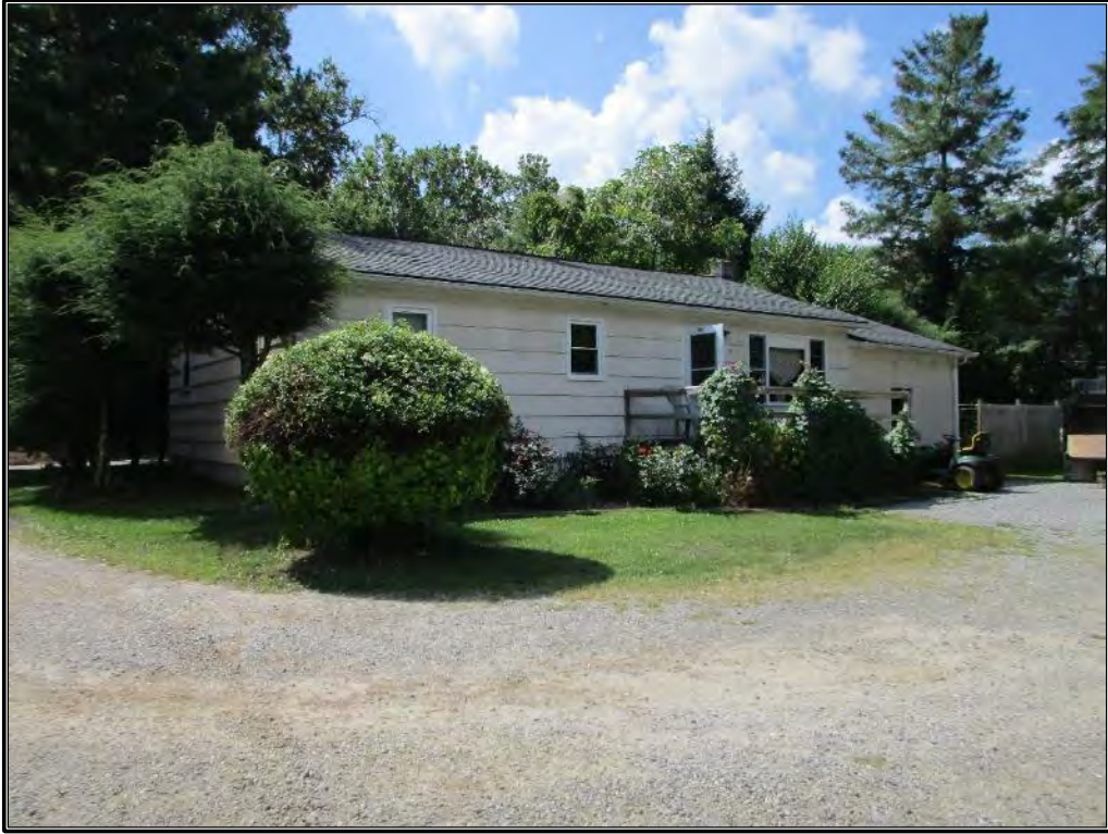
Figure 67. View of modern cottage (Cottage G), looking south.
