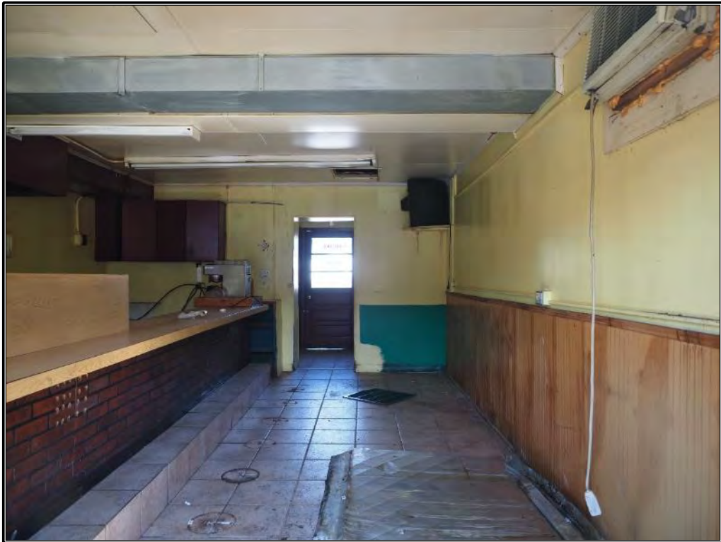
Figure 23. View of interior of commercial building from the front entry.
