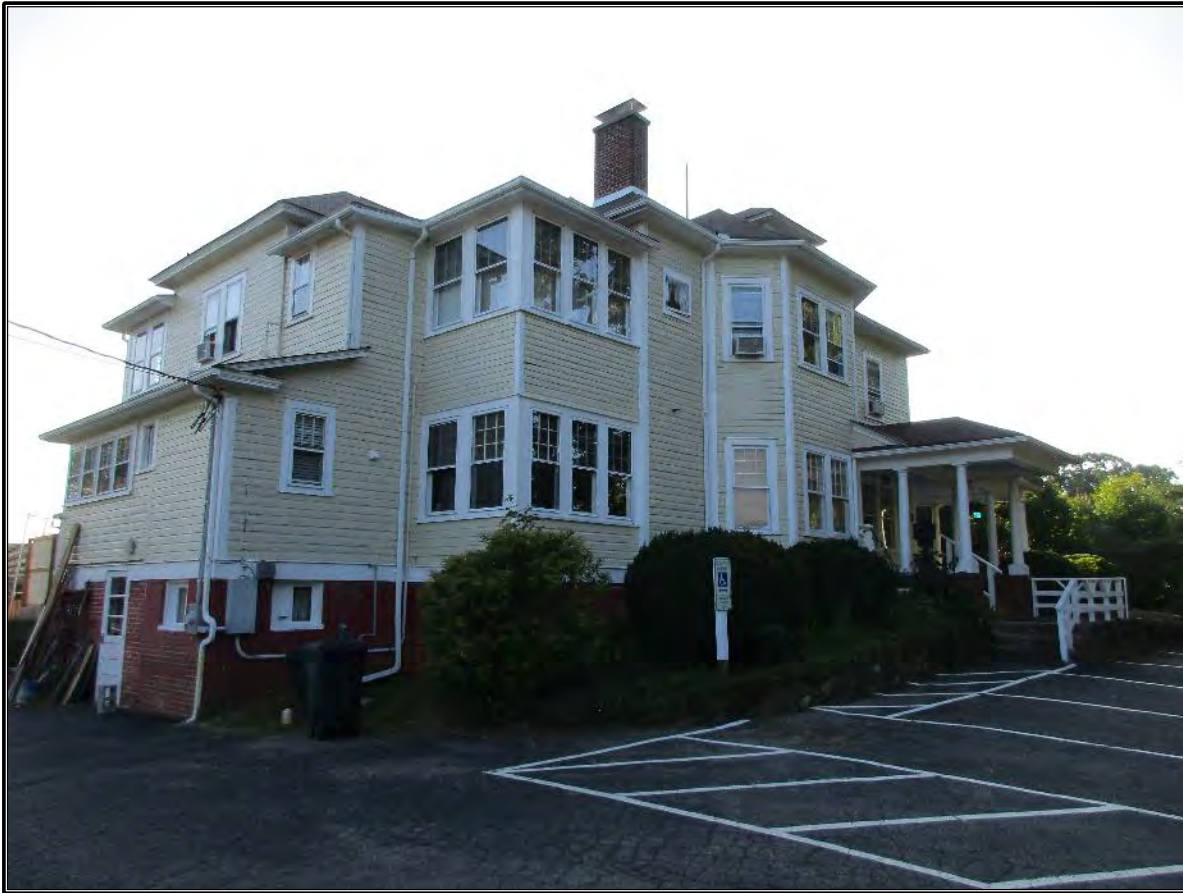
Figure 331. View of the southeastern (side) elevation.
