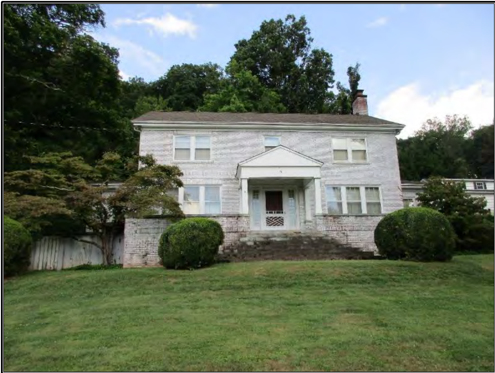
Figure 109. Façade of residence, looking north-northeast.
