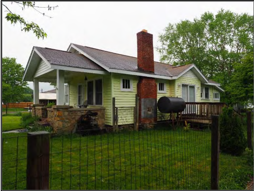
Figure 192. Residence at 10 Poplar Street, Waynesville.
