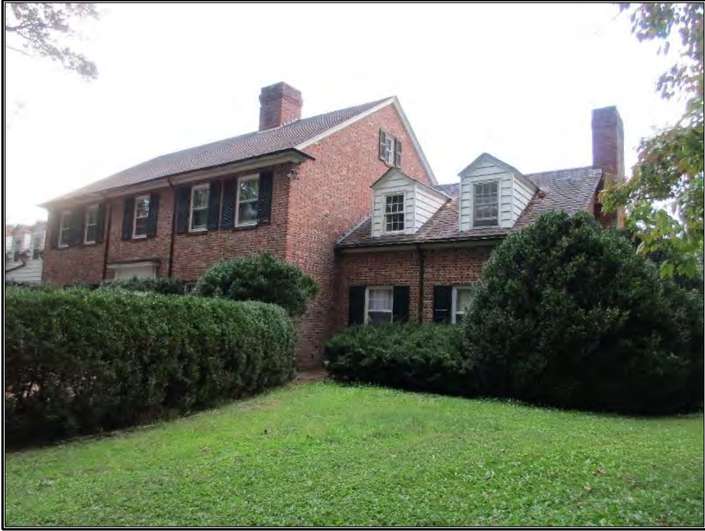
Figure 210. View of the west elevation of the southern wing.
