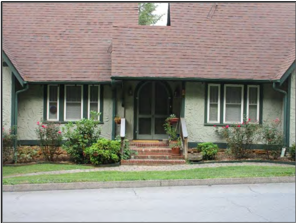
Figure 198. Detail of entry.
