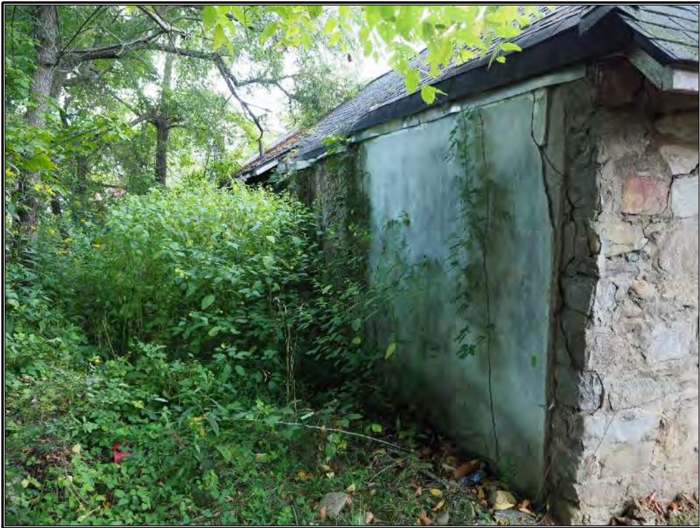
Figure 61. Rear elevation of linear building, looking north-northwest.
