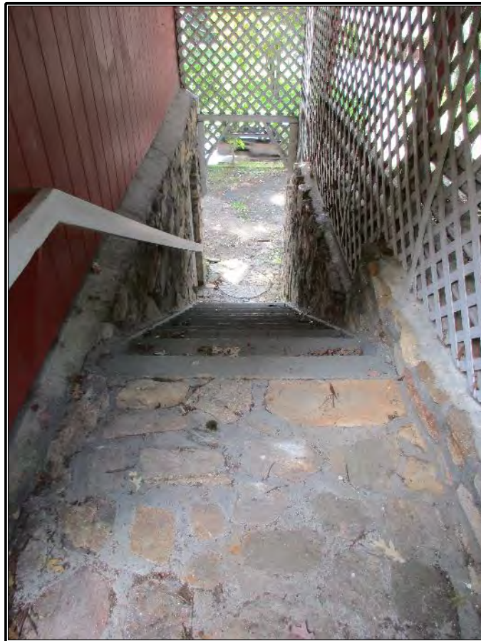
Figure 174. Concrete and stone stairs immediately next to the secondary residence.
