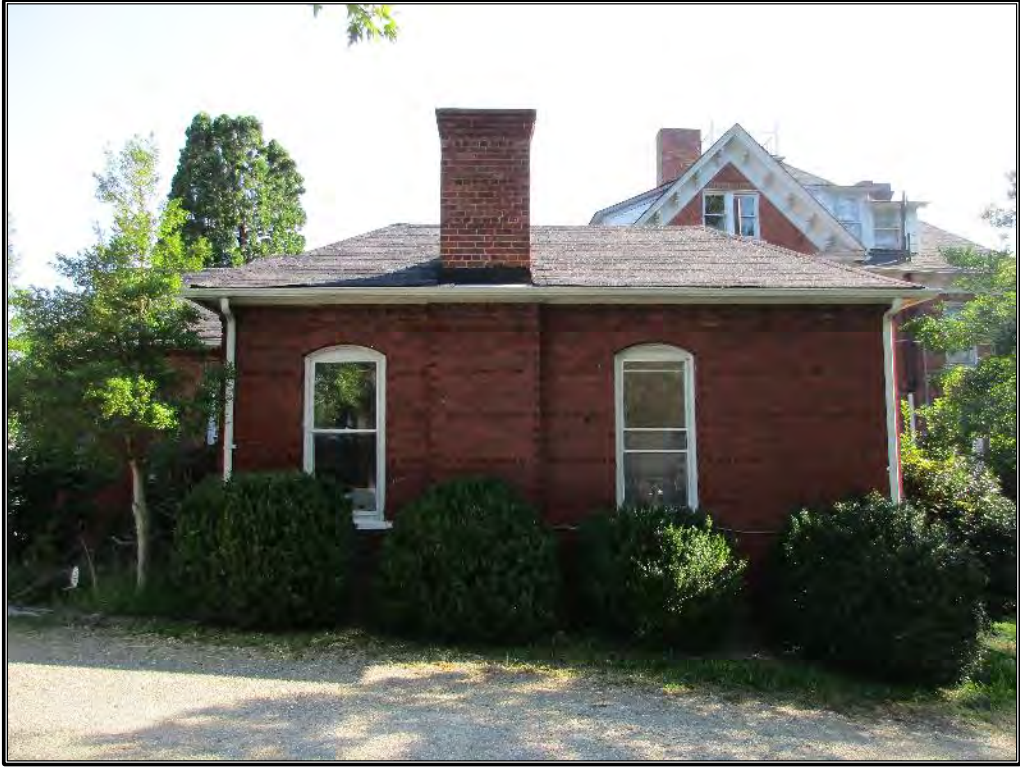
Figure 392. Southwest elevation of the office.
