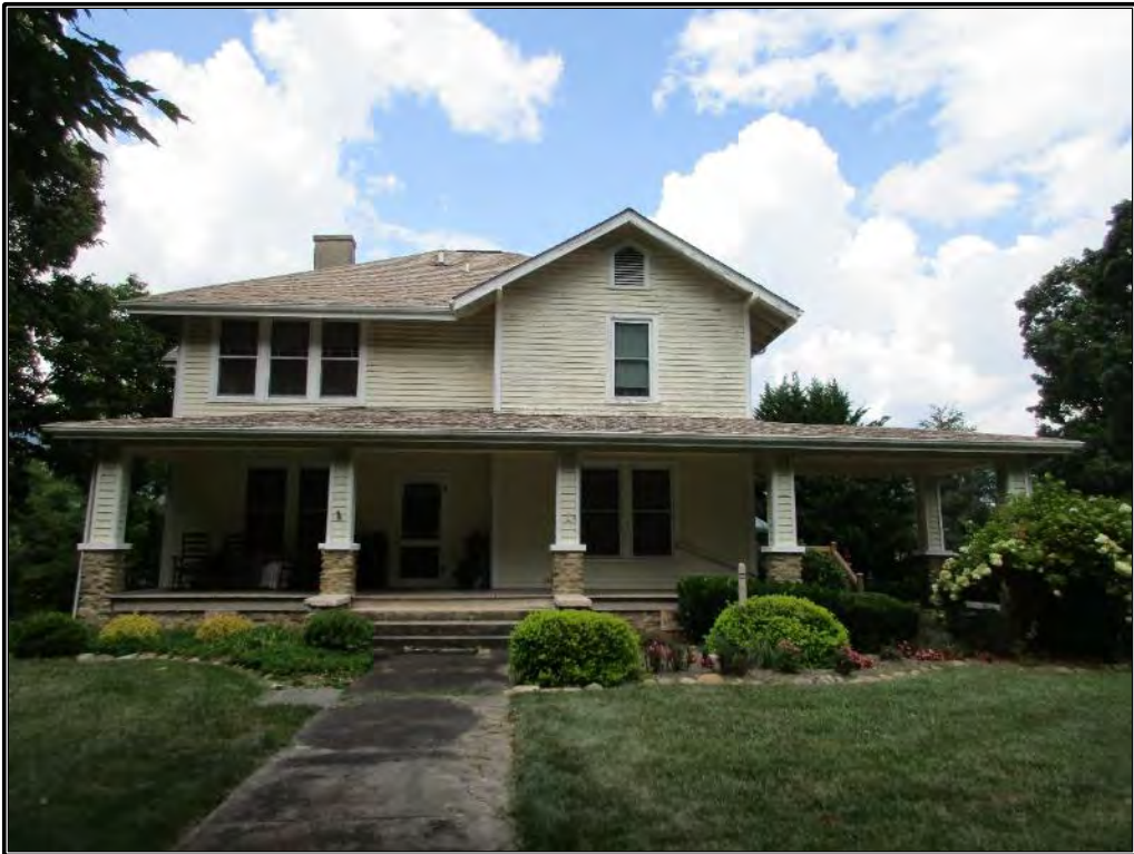
Figure 81. Façade of residence, looking north-northwest.
