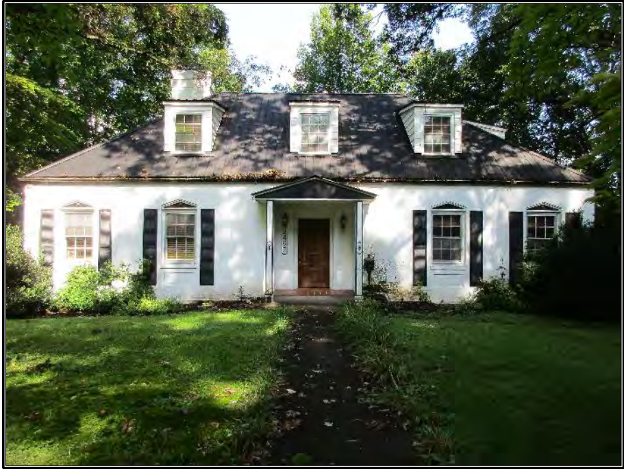
Figure 306. View of façade looking west.
