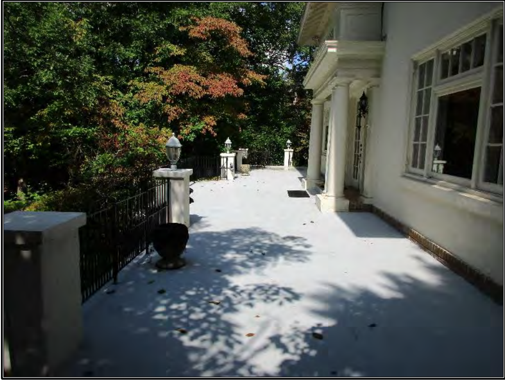
Figure 227. Detail of front porch and entrance.
