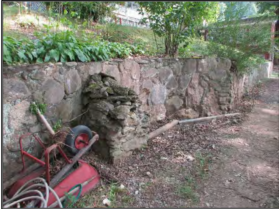
Figure 173. View of rock retaining walls along service road and stairs.
