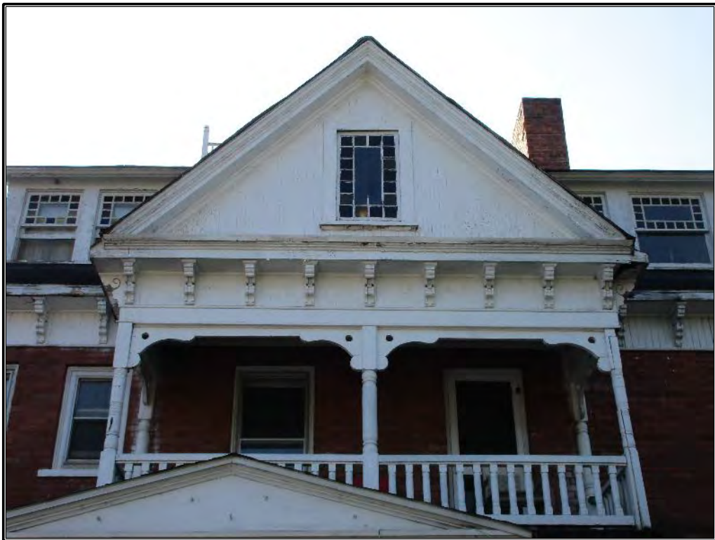
Figure 383. Detail view of the second-story porch on the façade.
