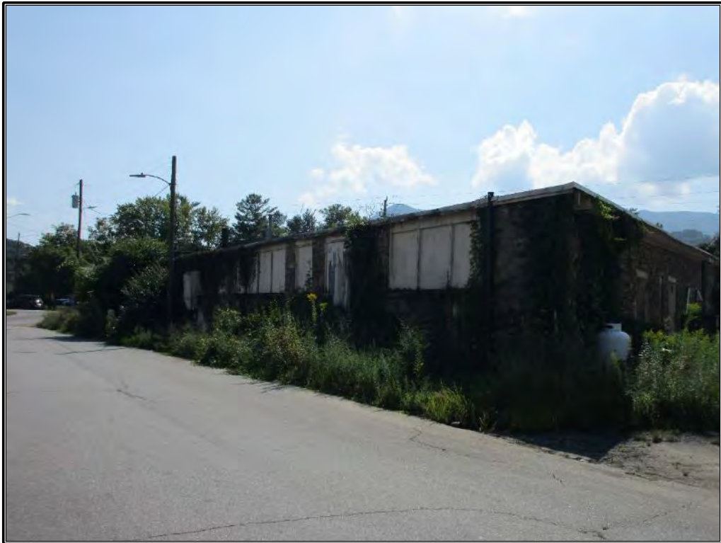
Figure 34. Rear elevation of commercial building, looking east-southeast.
