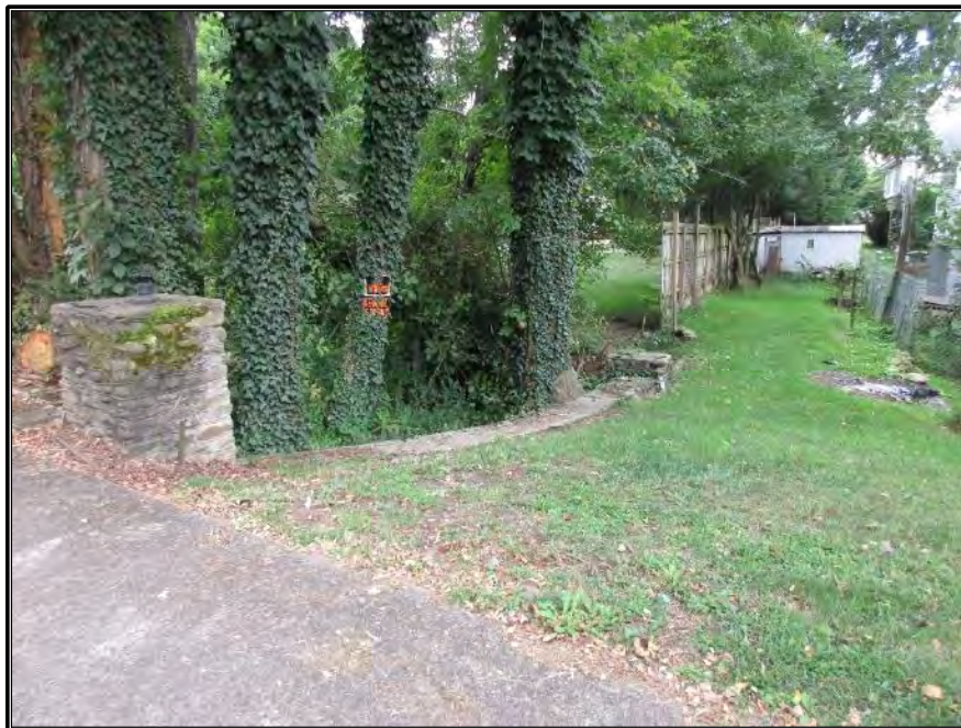
Figure 96. Overview of former driveway and gateposts, looking south-southwest.
