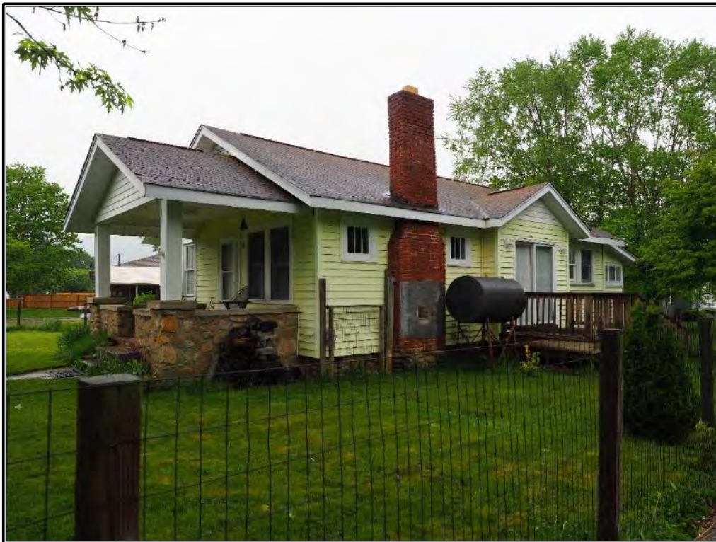
Figure 184. Residence at 10 Poplar Street, Waynesville.
