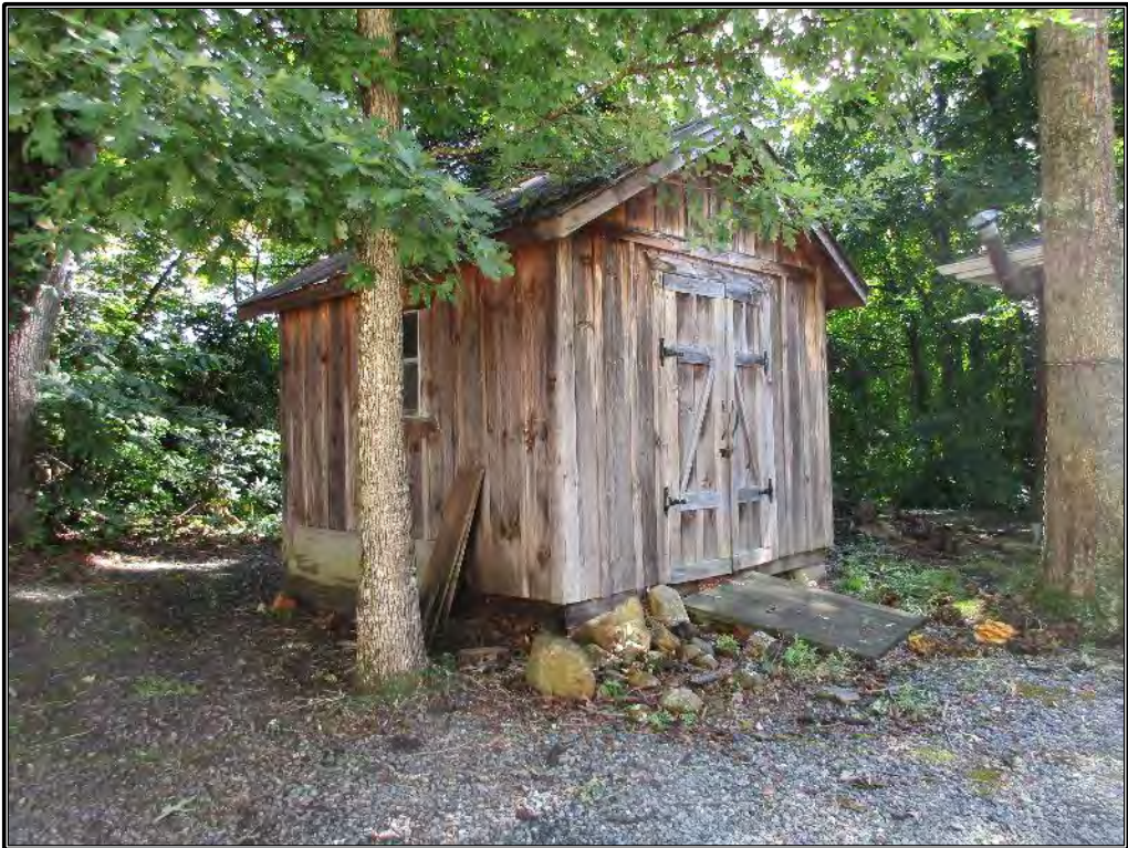
Figure 238. View of shed on the northern edge of the property.
