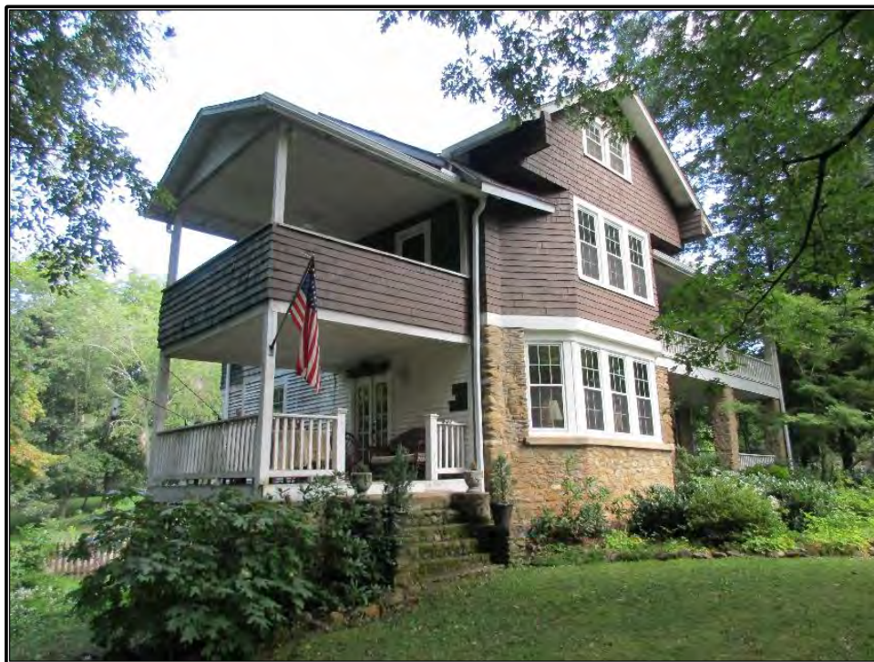
Figure 248. View of south corner with two-story porch.
