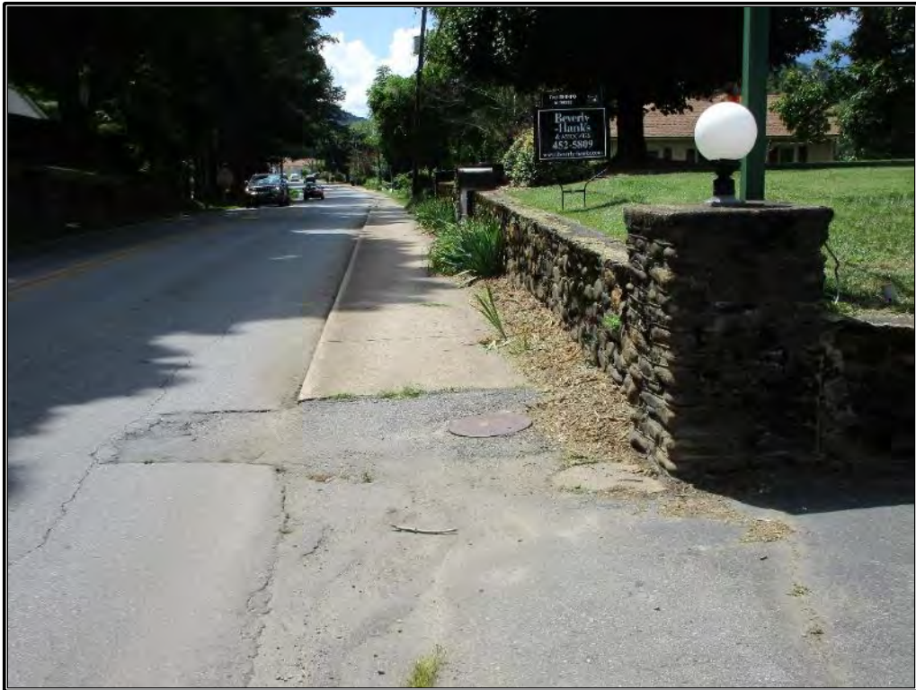
Figure 79. Overview of stone wall, looking west-southwest.
