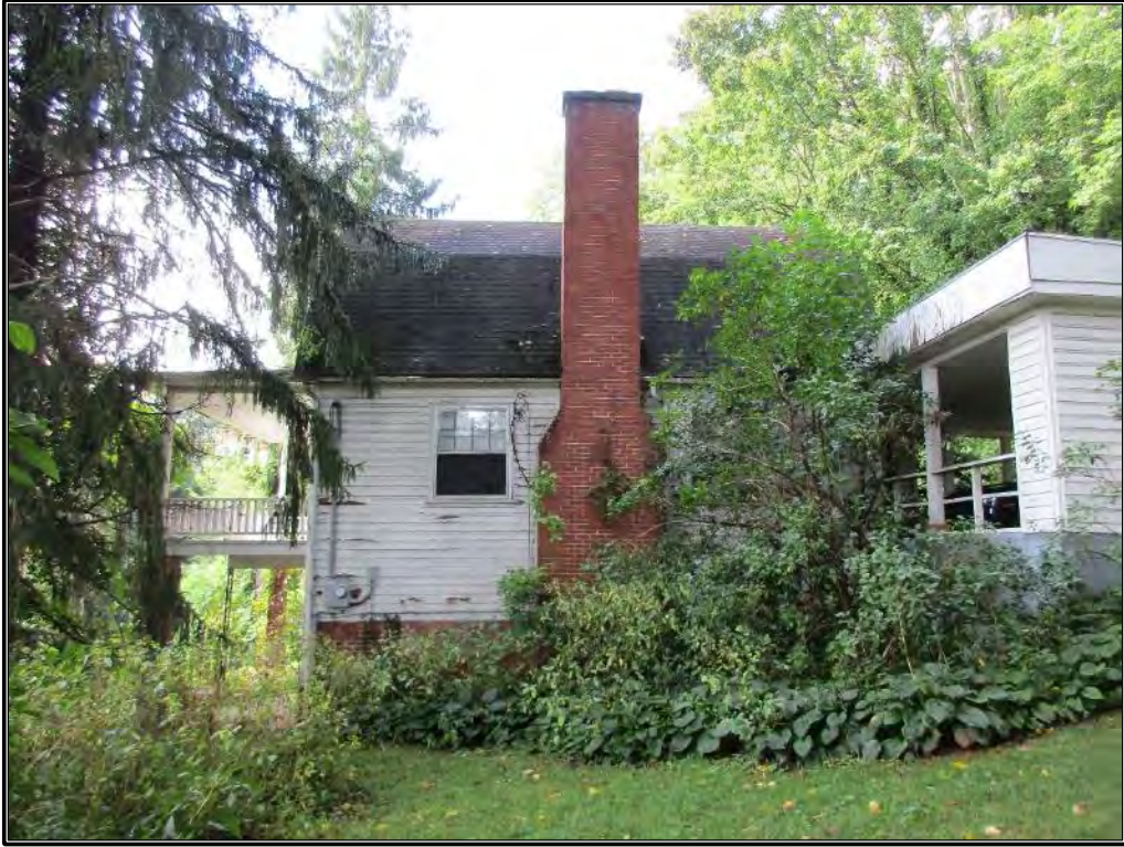
Figure 301. View of the northeast (side) elevation of the carriage house (HW0751).
