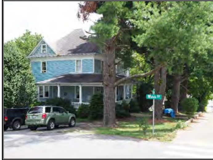
Figure 104. Residence at 101 East Street.
