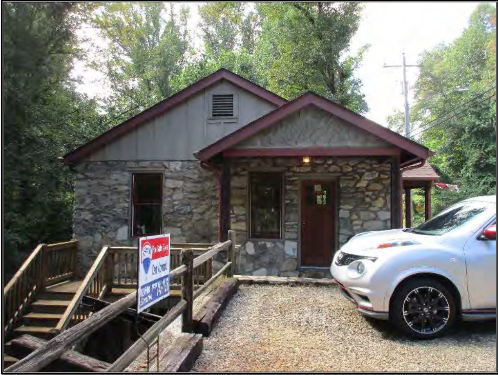
Figure 256. View of north elevation.
