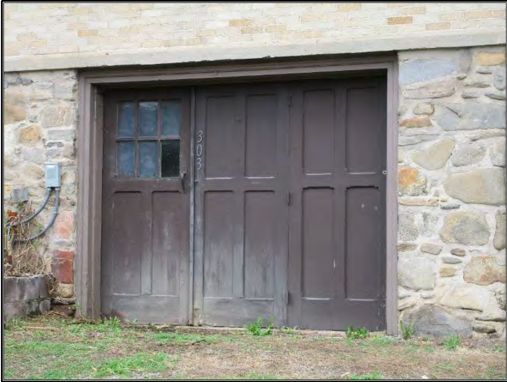
Figure 140. Detail of basement level garage.
