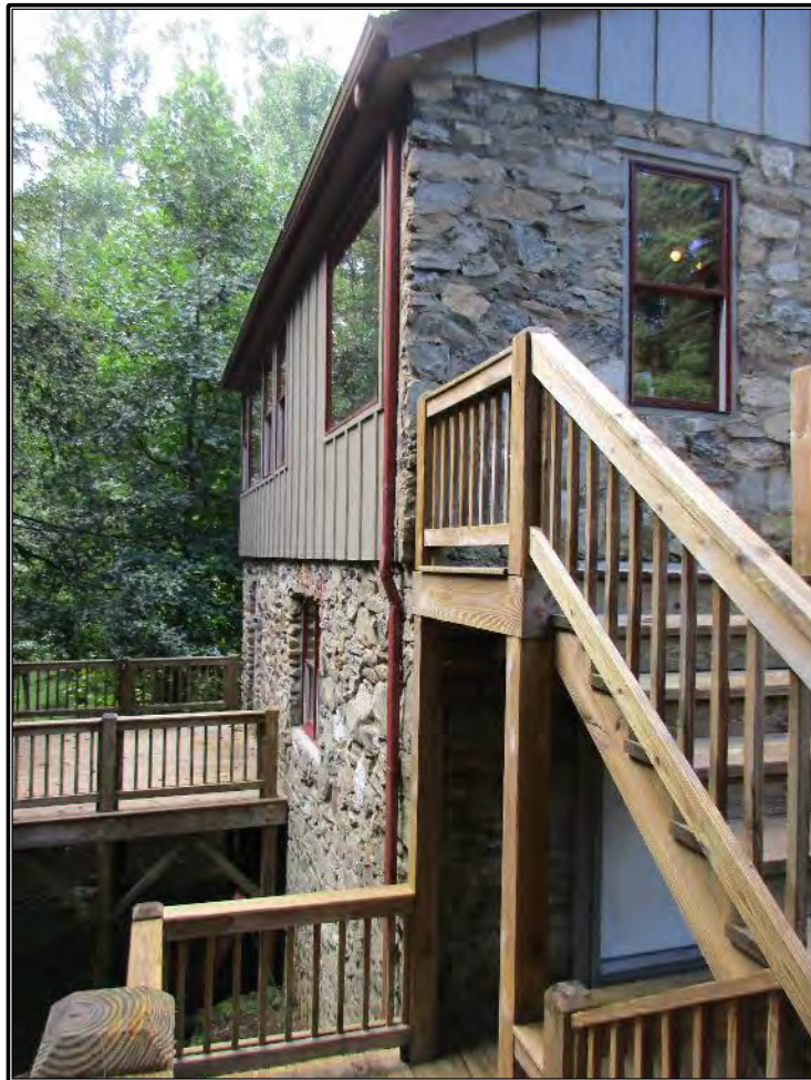
Figure 254. View of rear elevation.
