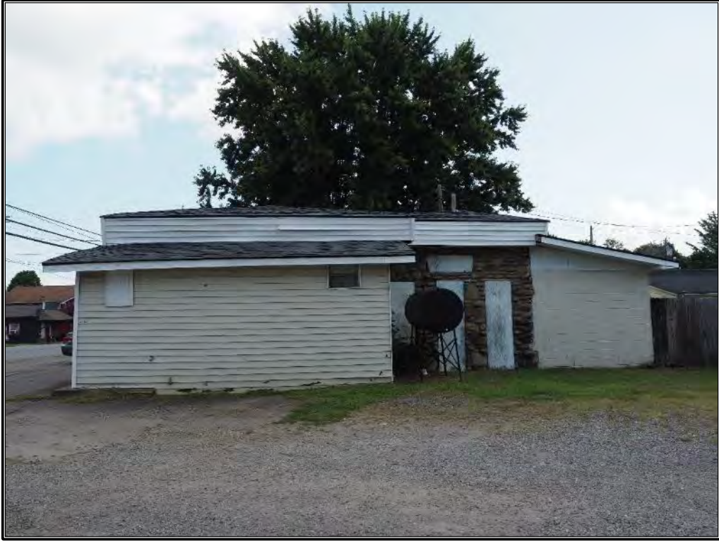
Figure 71. Southwest elevation of commercial building, looking north-northeast.
