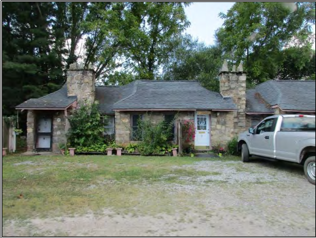
Figure 58. View of the second and third units, looking southwest.
