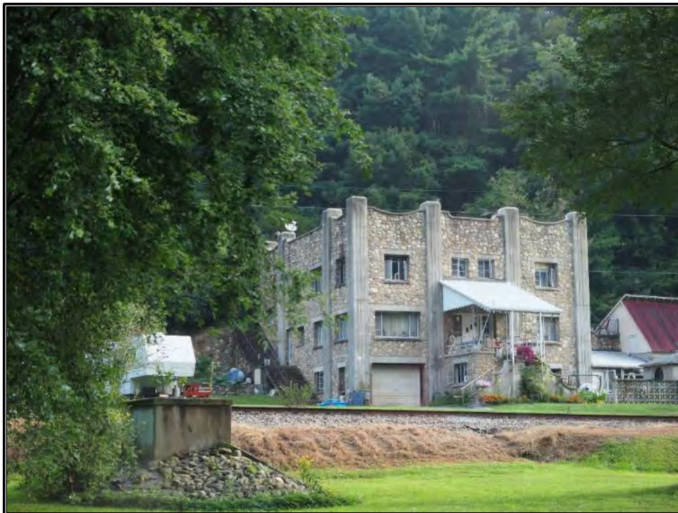
Figure 43. Rubble-rock masonry and cast-concrete commercial building along Asheville Highway east of Canton. This circa 1930–1950 building is among the largest and most intact examples encountered during the survey.
