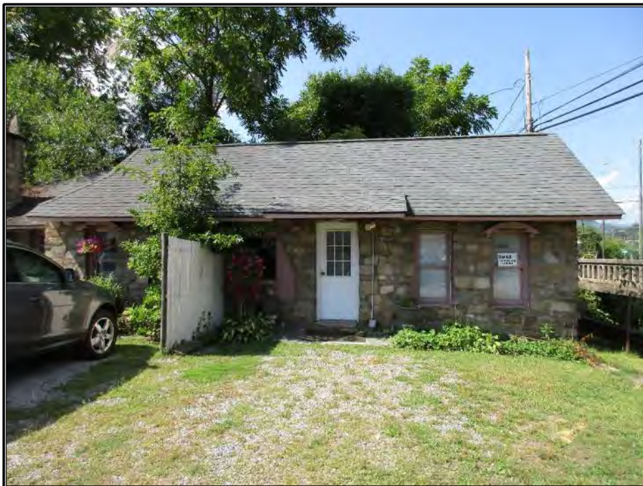
Figure 57. View of the first unit, looking southwest.
