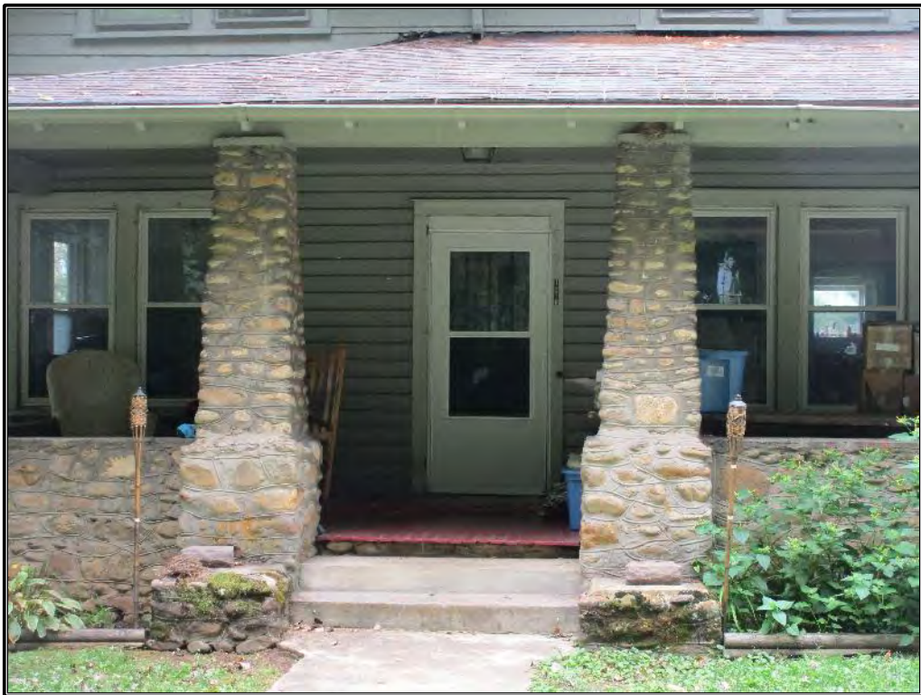
Figure 147. Detail of front entry and porch posts.
