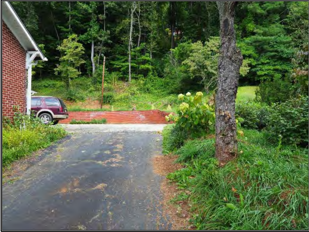
Figure 117. View of driveway and brick retaining wall, looking east.
