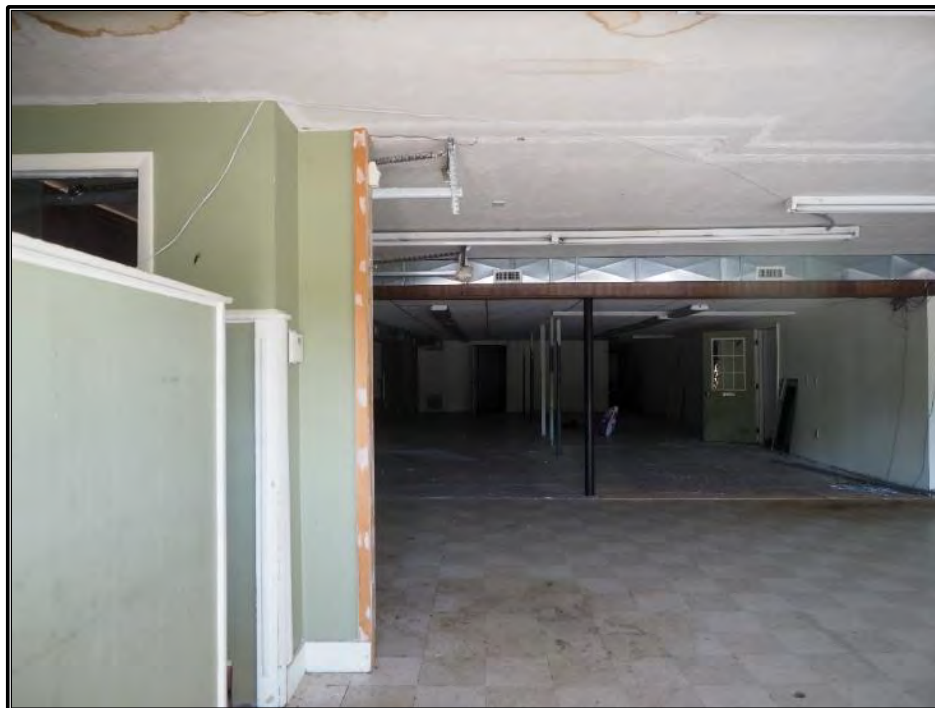
Figure 37. Interior view of northeast façade storefront.
