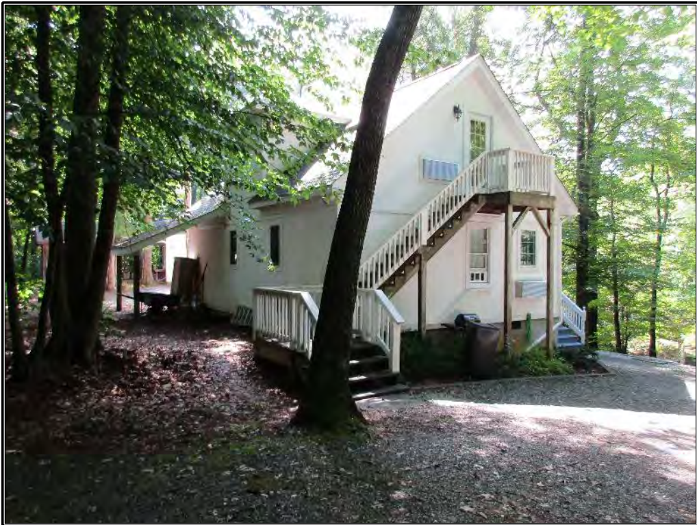
Figure 234. Secondary dwelling, view of northwest corner.
