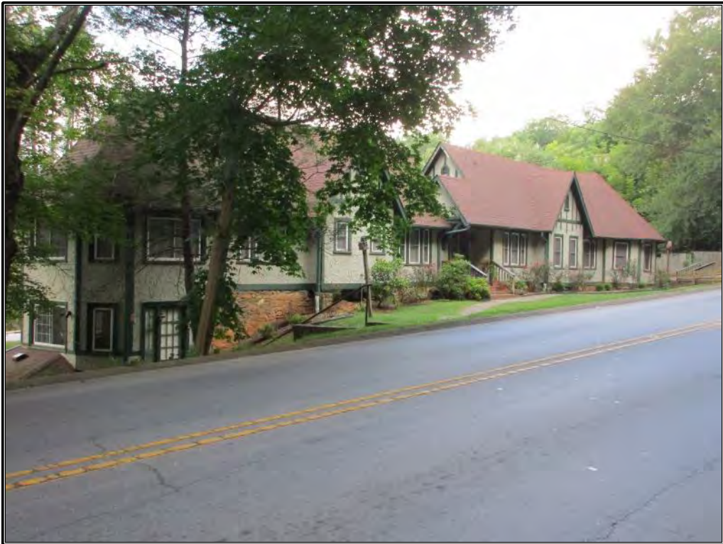
Figure 196. Southeast elevation with hyphen and entrances from sidewalk along South Main Street.
