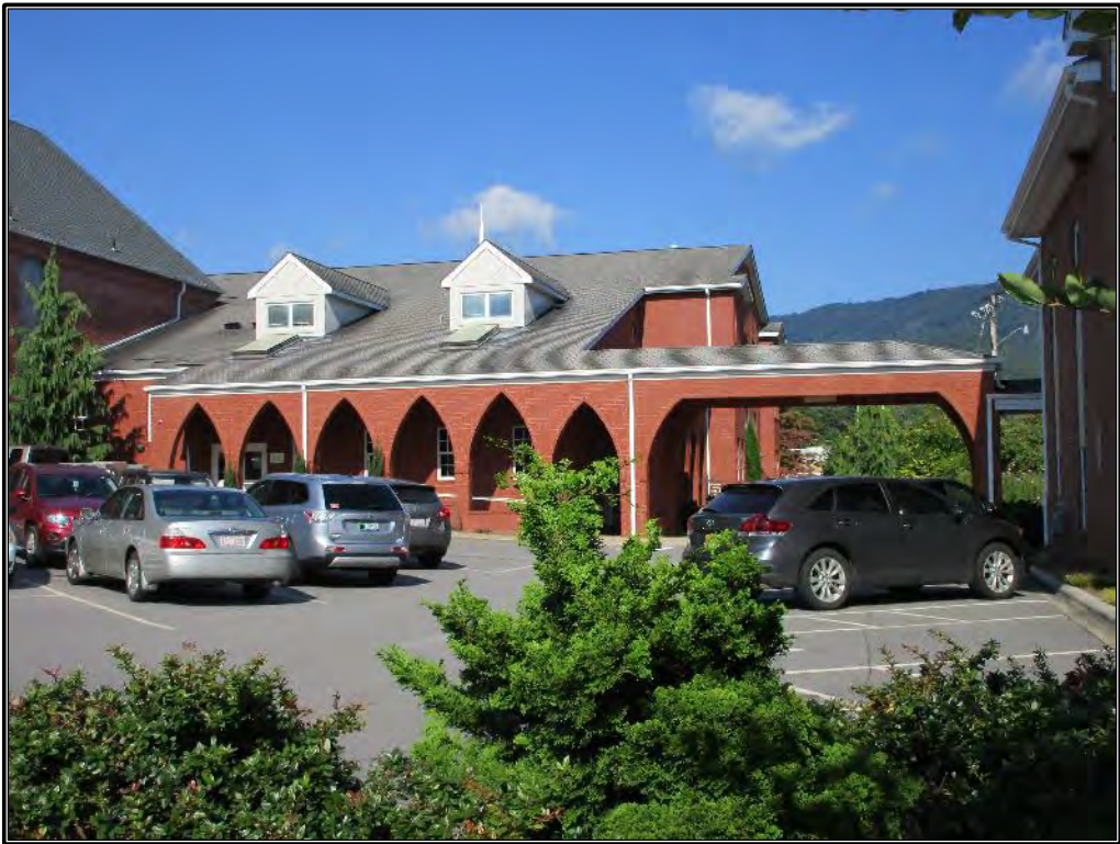
Figure 408. Eastern elevation of the office annex, connected to the northern elevation of the circa 1952 church sanctuary.
