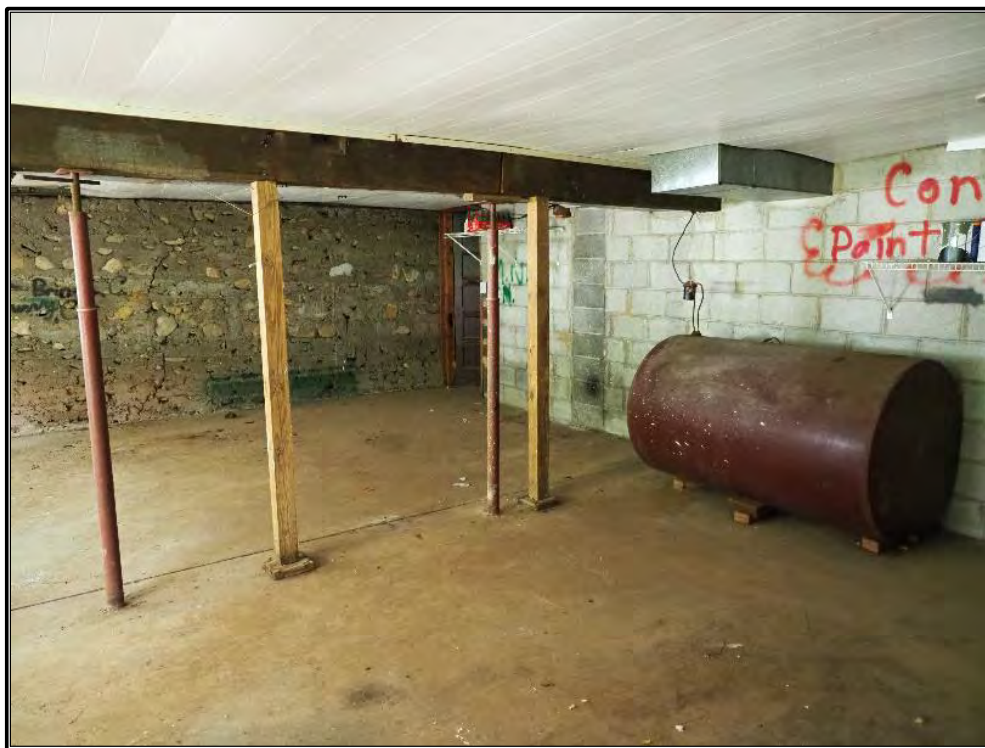
Figure 155. Interior of basement story of carriage house.
