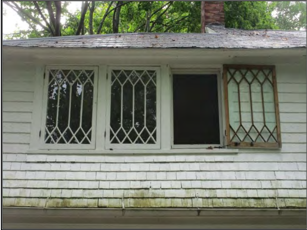
Figure 279. Detail of second-floor windows.
