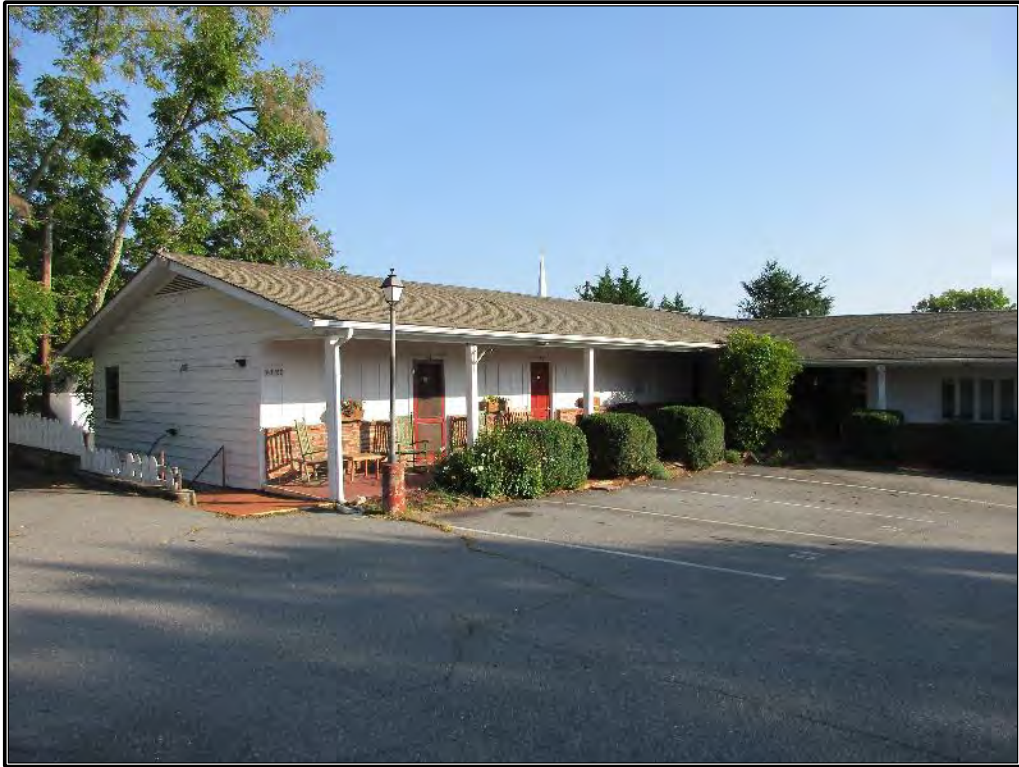
Figure 356. View of L-shape construction of Building B looking northwest.
