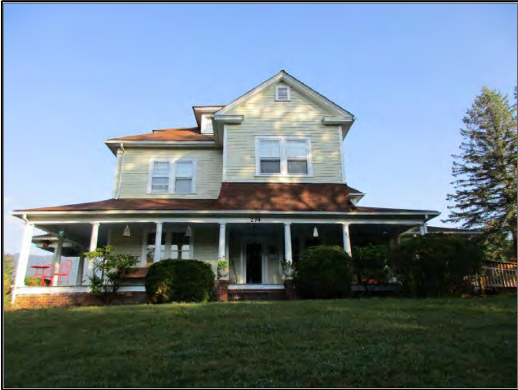
Figure 329. View of the façade looking northwest.
