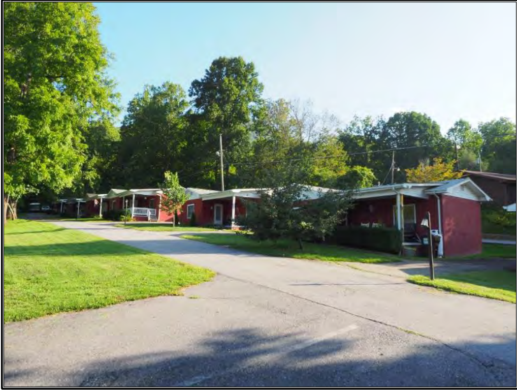
Figure 75. Detail of a row of individual guest houses at Leatherwood Cottages in Maggie Valley.
