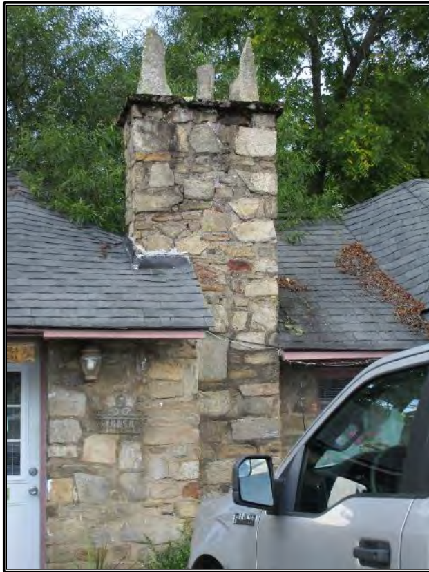
Figure 56. Detail of façade chimney.
