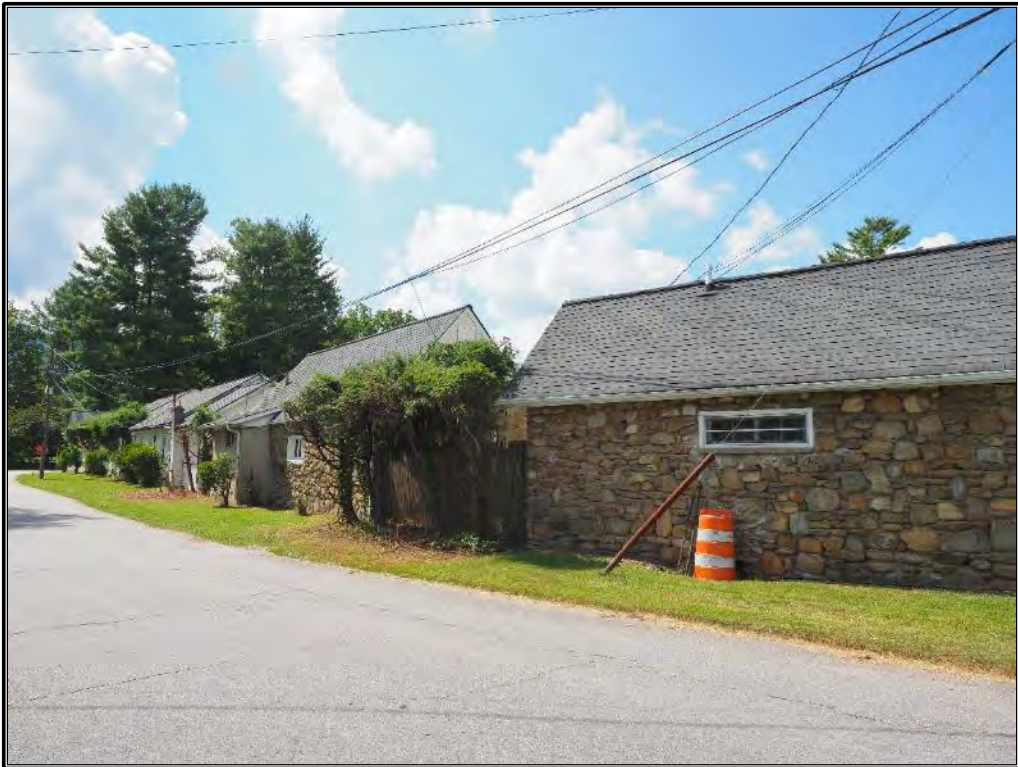
Figure 65. Rear view of northeast row of cottages (Cottages A-F), looking south-southeast.
