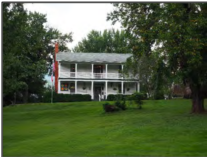
Figure 400. Façade view of the Shelton House (HW0003) on Pigeon Road, Waynesville.
