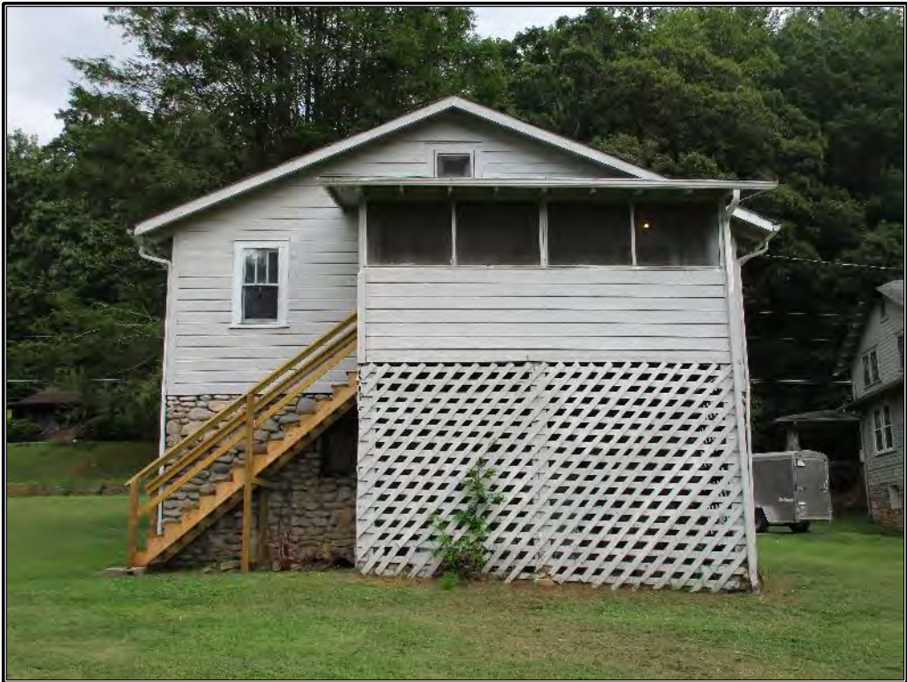
Figure 154. West elevation of carriage house, looking east-southeast.
