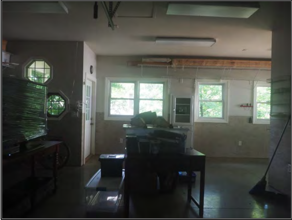
Figure 237. Large interior room of the workshop.
