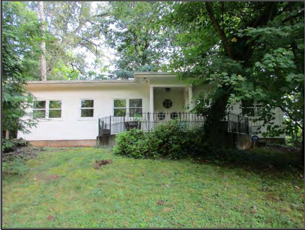
Figure 235. Workshop façade looking north.
