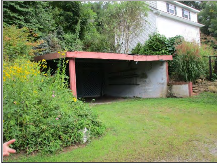
Figure 114. View of detached carport, looking southeast.
