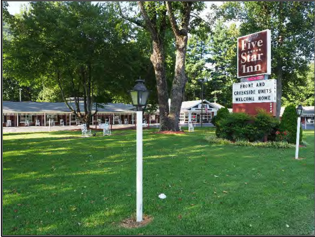
Figure 366. View of the Five Star Motel with sign.
