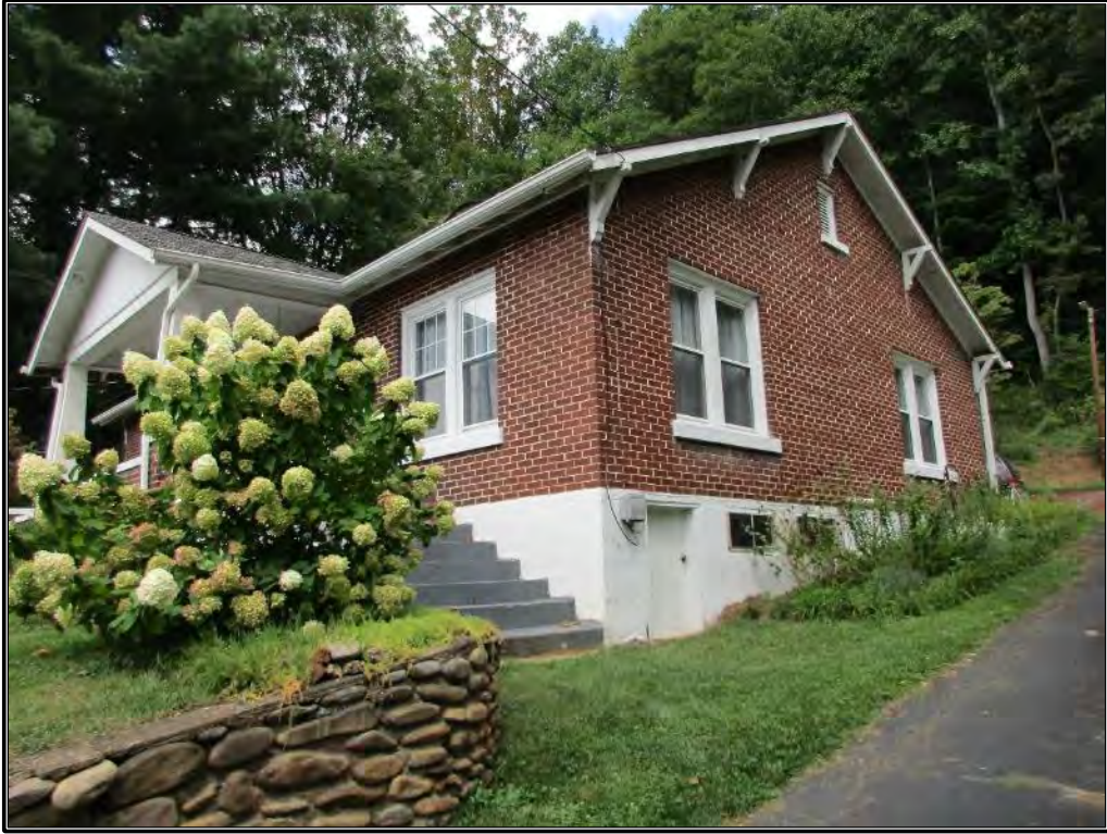
Figure 124. Façade and south elevation of residence, looking north-northeast.
