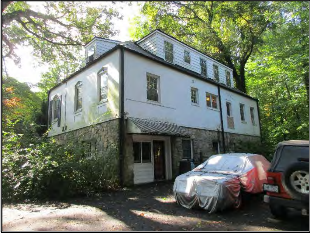
Figure 311. View of rear elevation.
