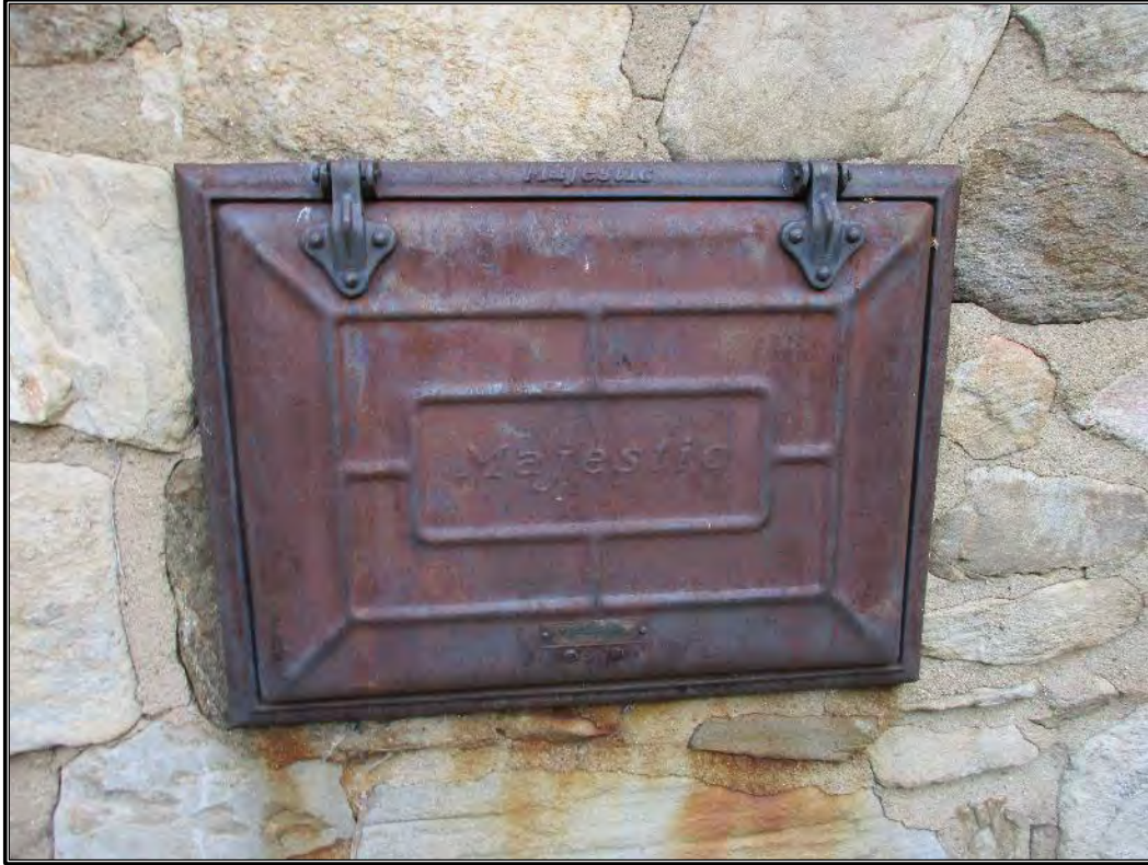
Figure 165. Coal chute on south elevation.
