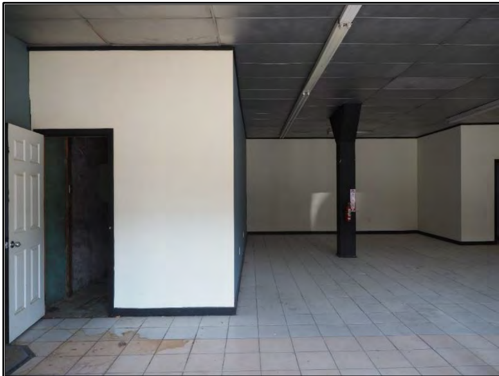
Figure 36. Interior view of center façade storefront.
