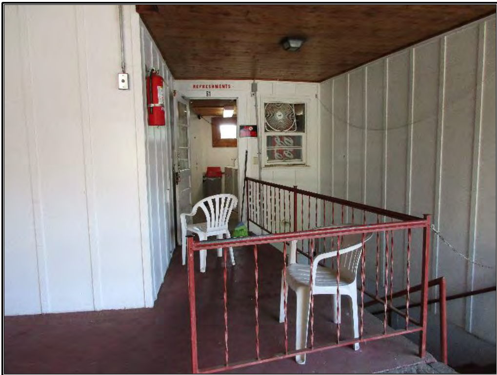
Figure 357. View of recessed laundry access.
