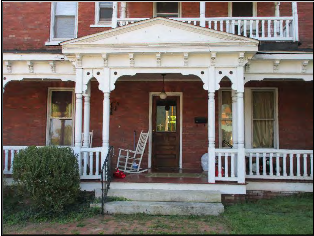
Figure 382. Detail view of front entry.
