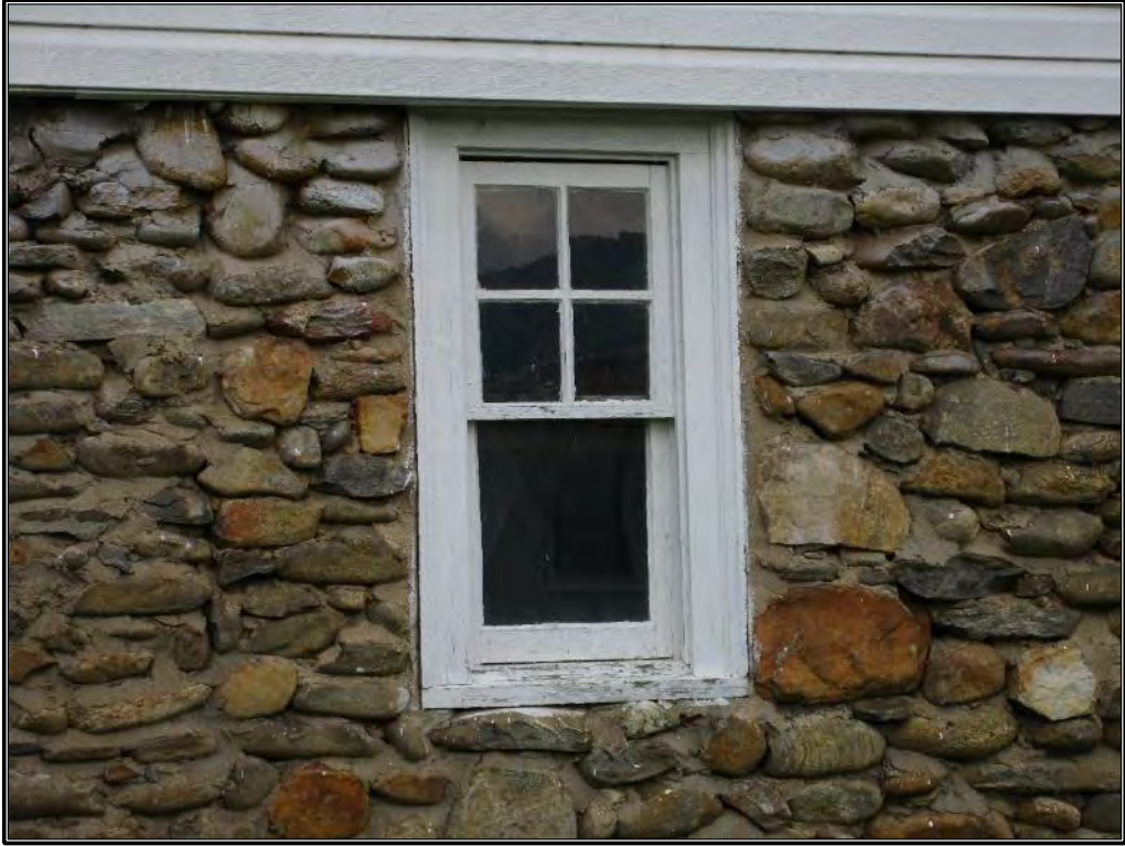
Figure 99. Detail of historic window.
