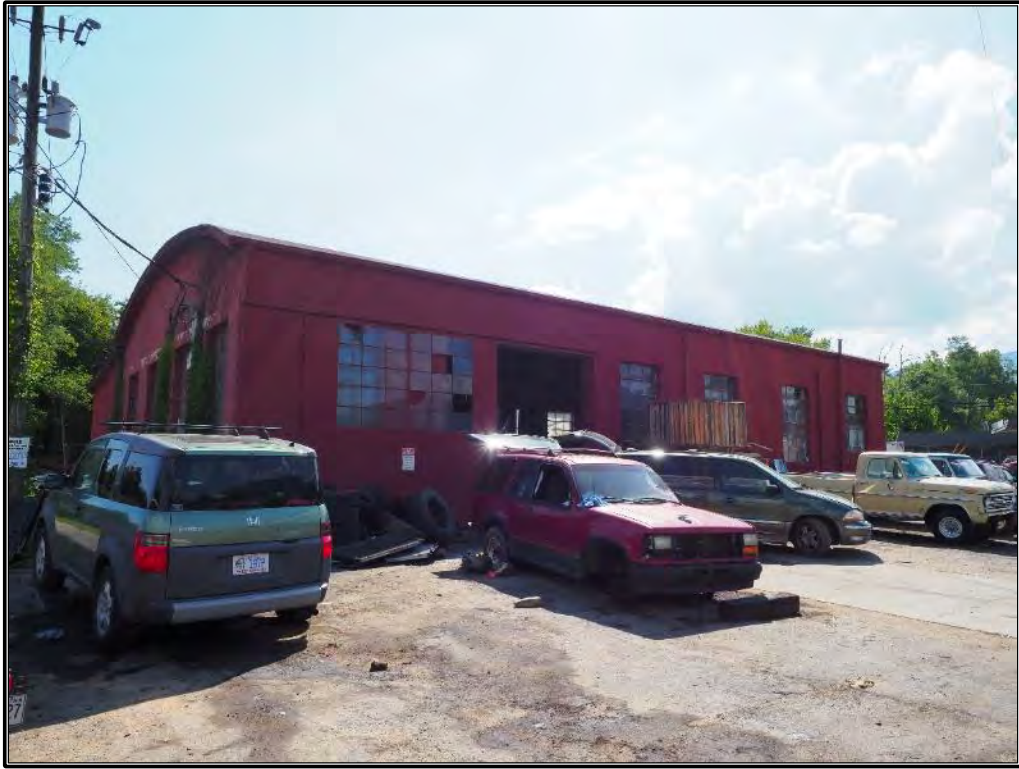
Figure 46. West and rear elevation of repair shop, looking east-southeast.
