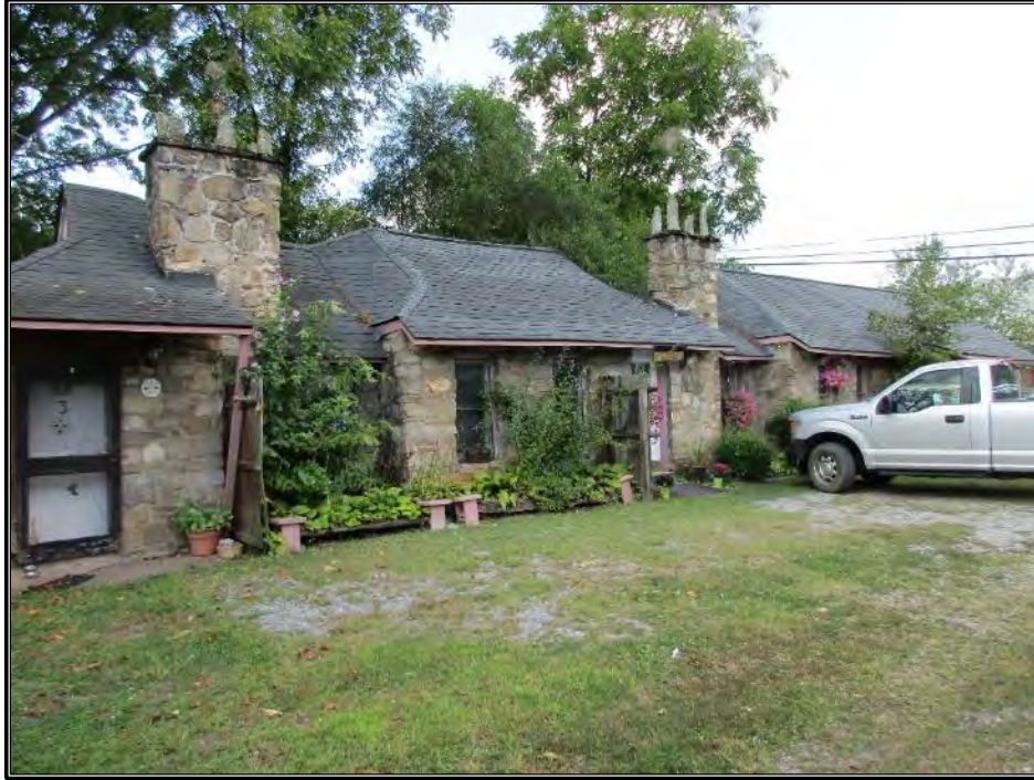
Figure 54. Façade of linear building, looking west.
