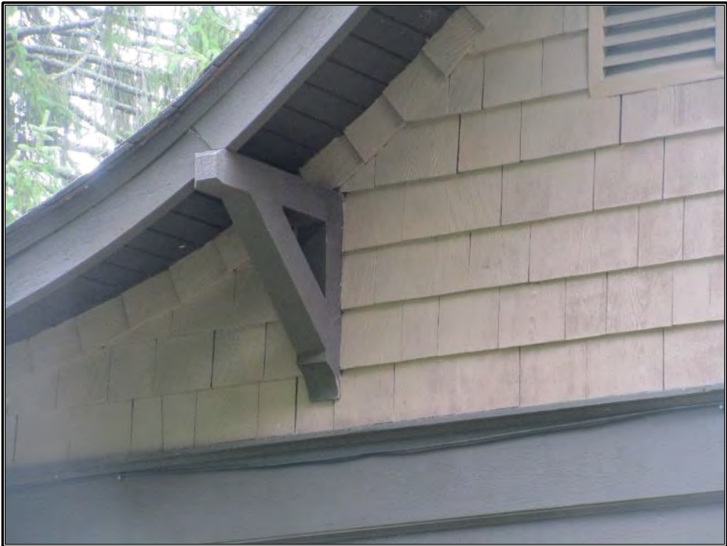
Figure 134. Detail of brackets and eaves.
