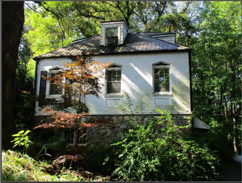
Figure 309. View of northeast (side) elevation.
