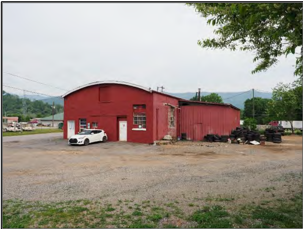
Figure 47. Façade and east elevation of repair shop, looking northwest.
