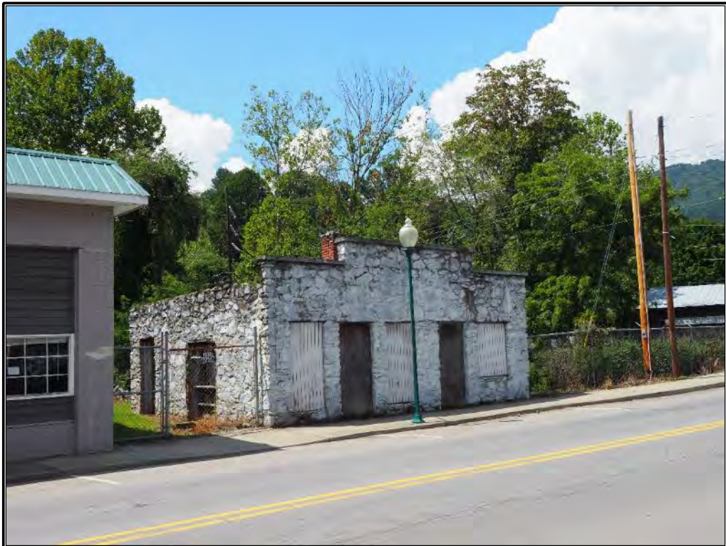
Figure 25. Rubble-rock masonry, circa 1940 commercial building in Frog Level, just west of the Waynesville Main Street Historic District (HW0161) on Depot Street adjacent to Richland Creek.
