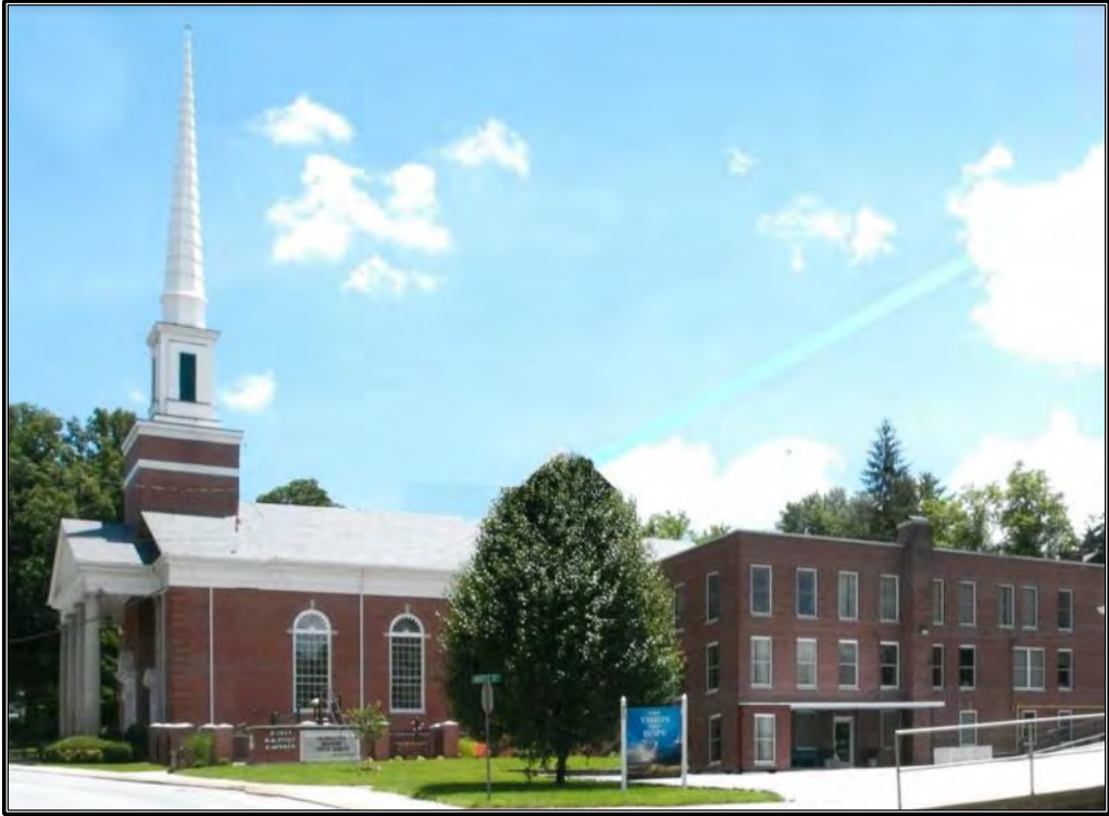
Figure 421. View of Canton First Baptist Church on Academy Street, Canton.
