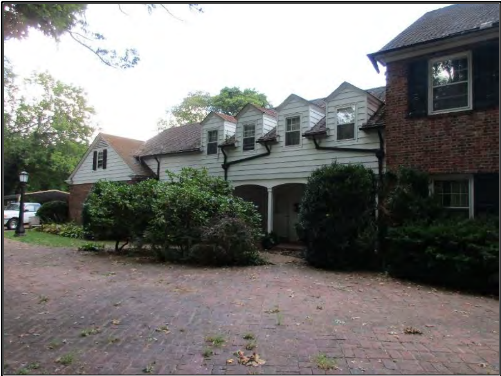
Figure 213. View of the west elevation of the northern wing.
