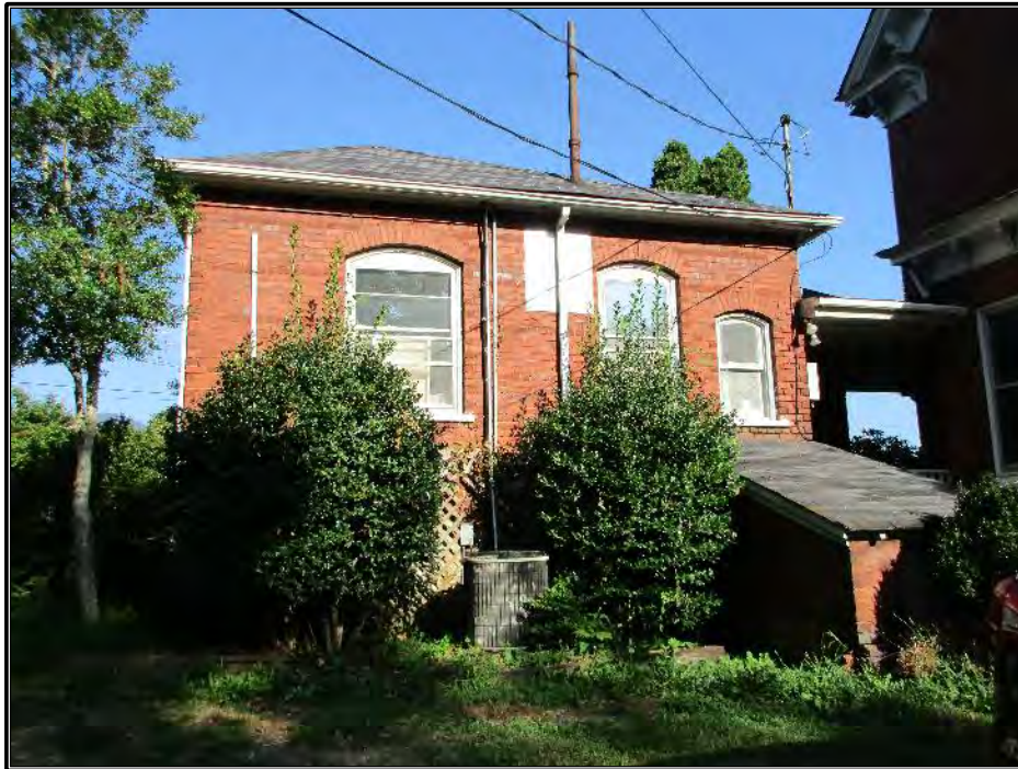
Figure 395. Rear elevation of the office.
