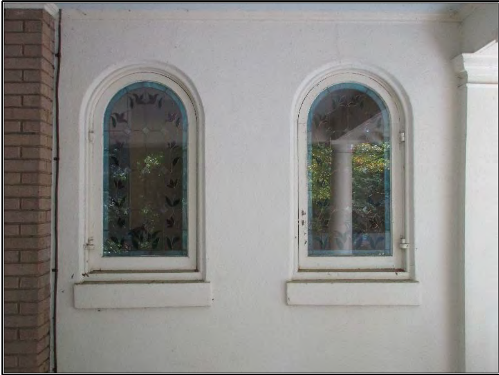
Figure 229. Detail of arched, stained glass windows.
