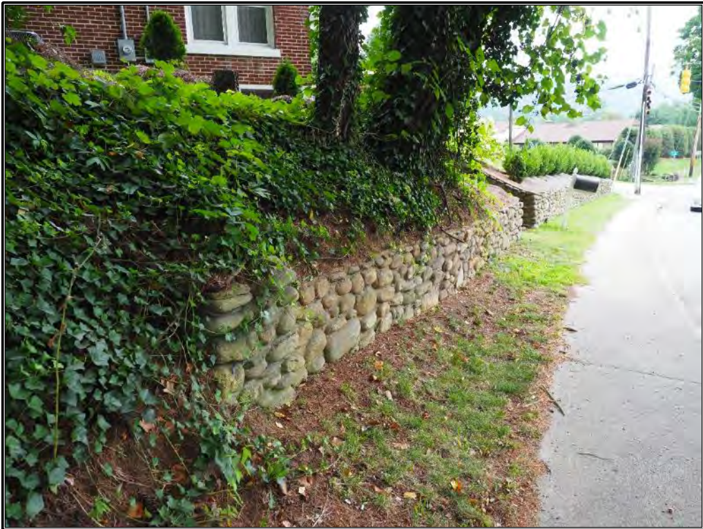
Figure 118. View of river rock retaining wall and steps, looking south-southwest.
