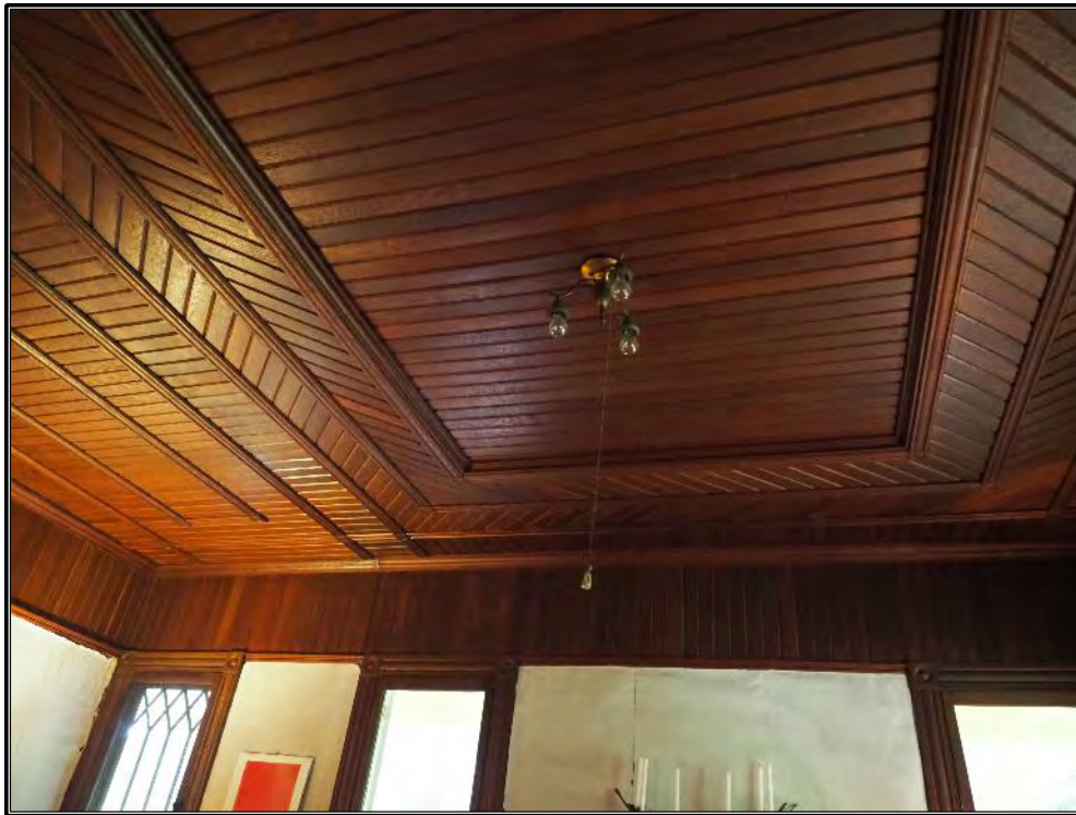
Figure 288. Detail of the living room ceiling.
