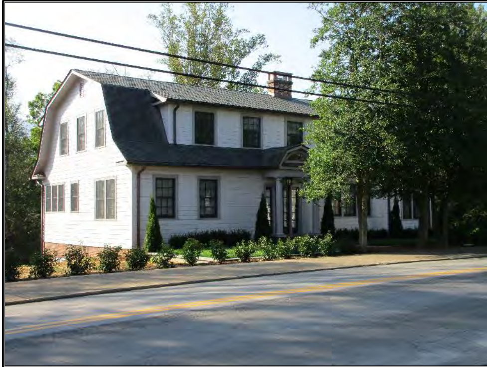
Figure 370. Façade view of the residence, looking south.
