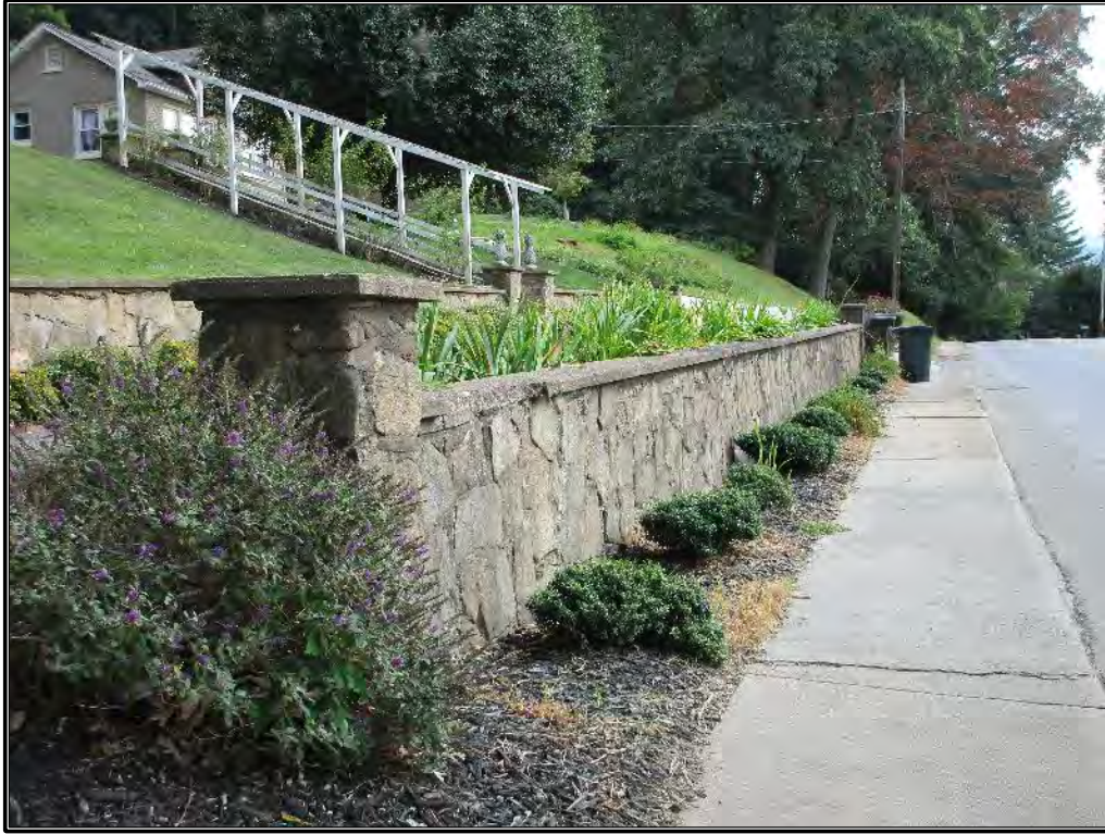
Figure 161. Stone walls along service drive.
