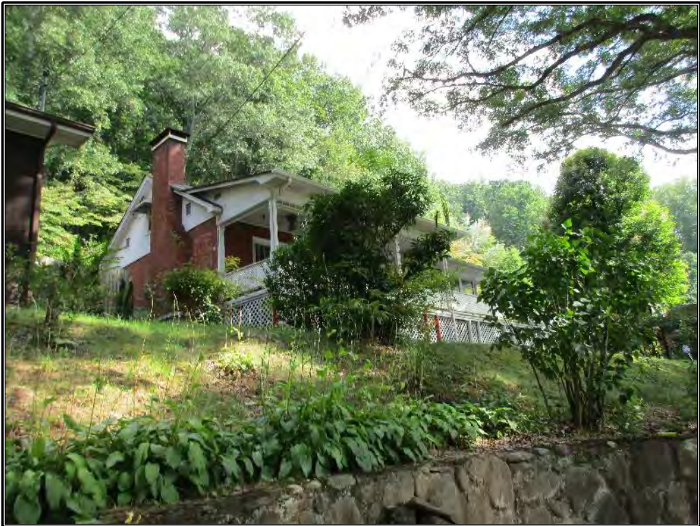
Figure 180. Northern elevation showing steeply sloping lot.
