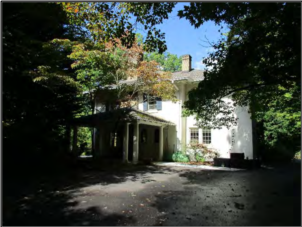
Figure 228. Northeast side elevation with hip-roof porch.
