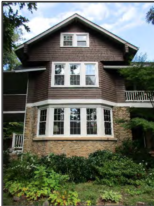
Figure 247. Detail of façade projection.
