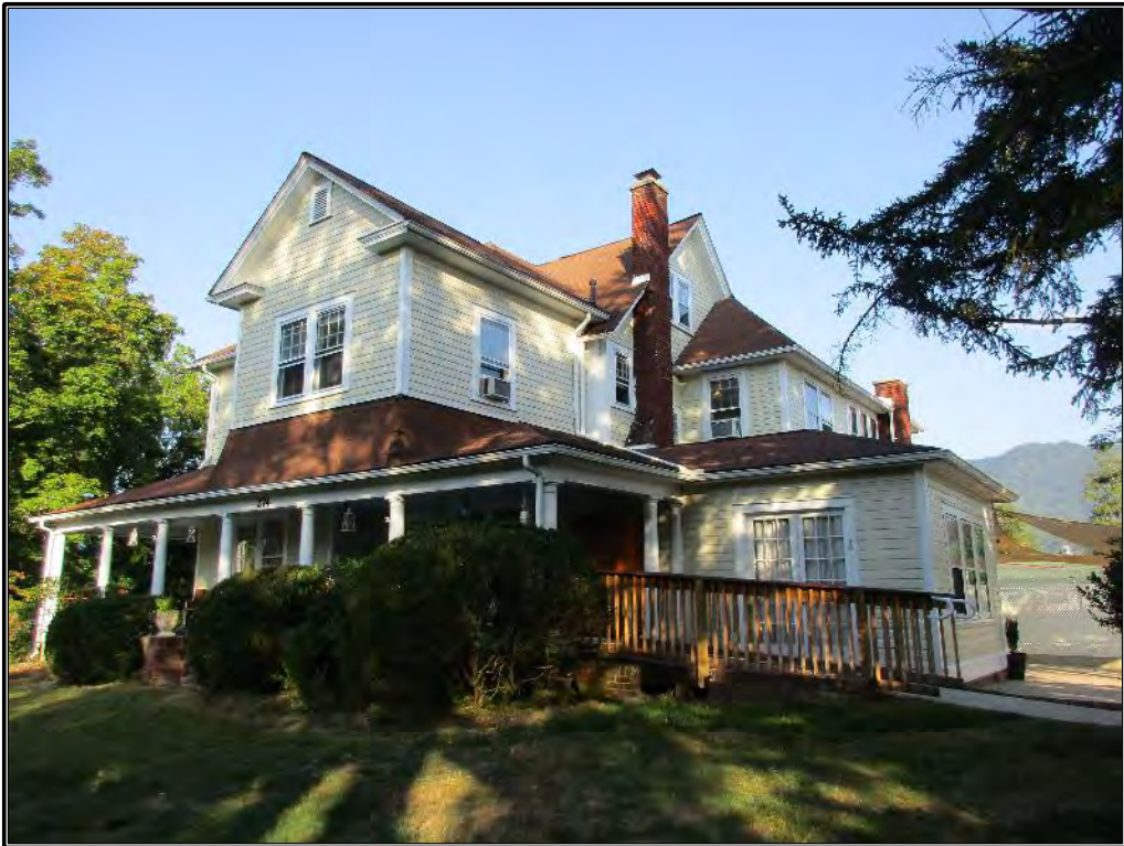
Figure 330. View of the northeastern (side) elevation with chimney.
