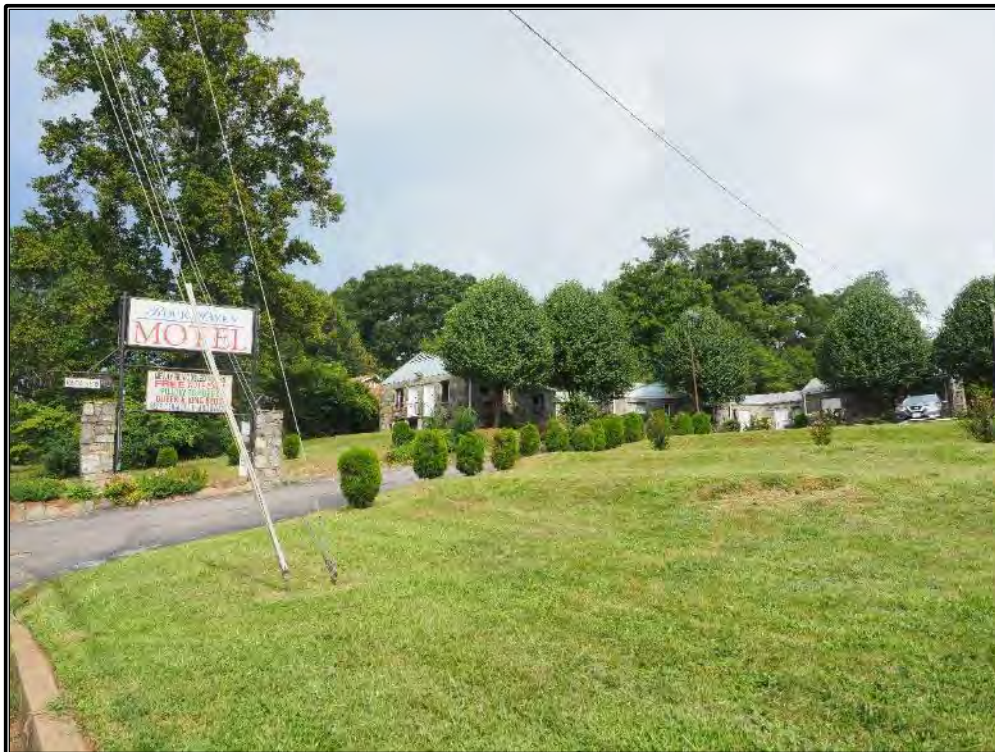
Figure 74. The Rock Haven Motel located in West Asheville on Patton Road featuring stone veneer and linear buildings with multiple guest rooms.
