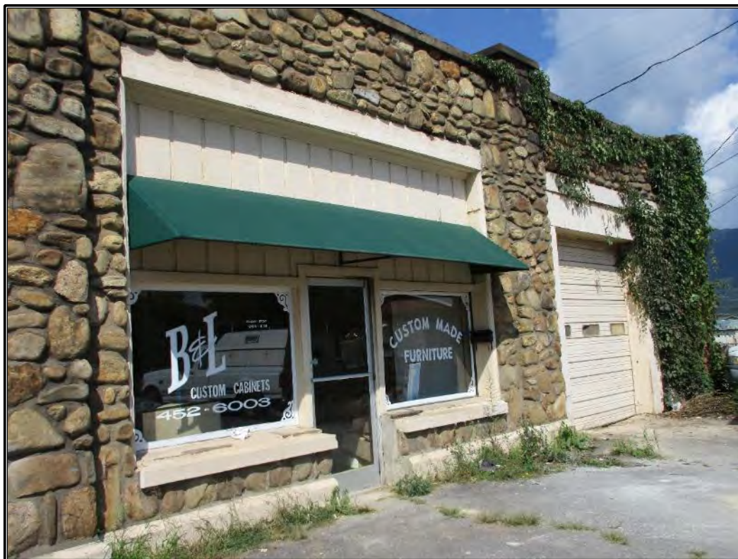
Figure 32. Detail of storefront along the northeast elevation.
