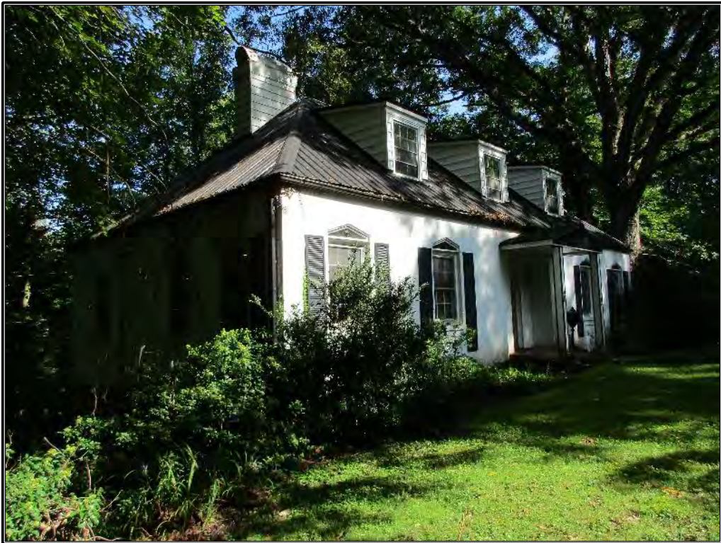
Figure 310. View of the building's southern corner.
