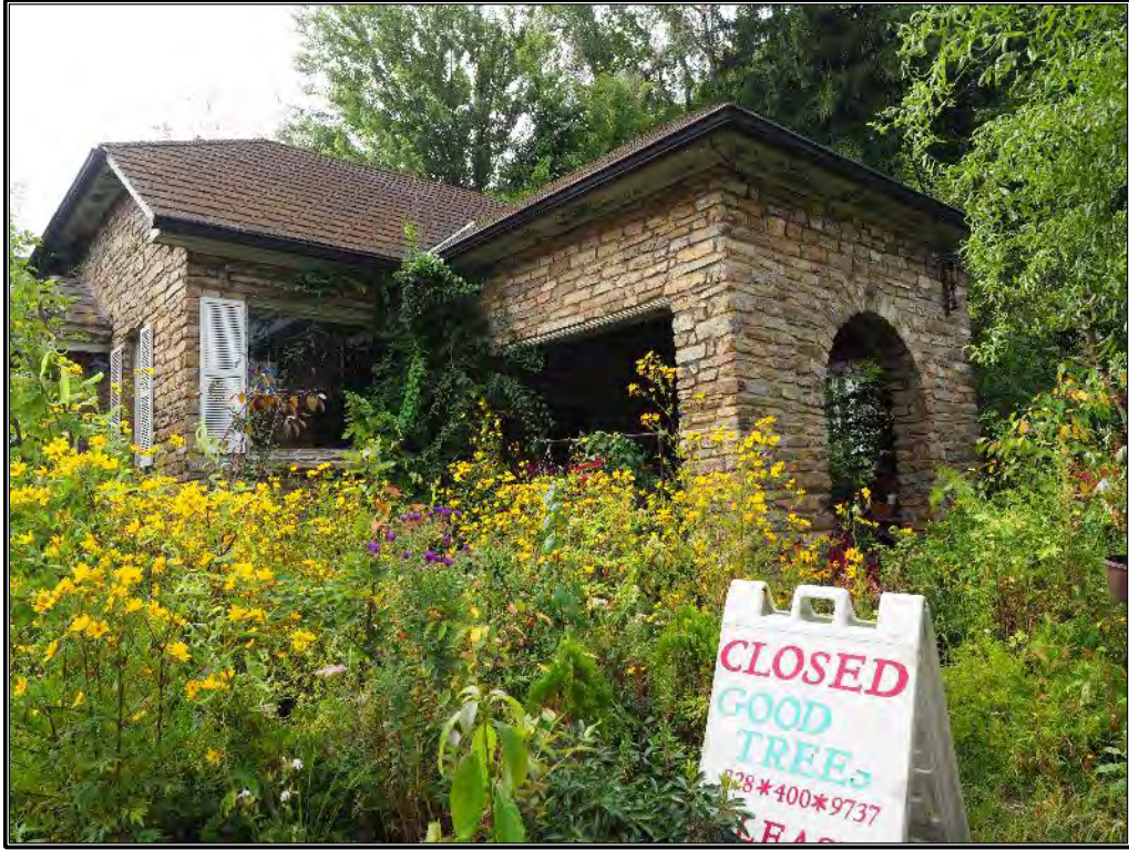
Figure 260. Residence converted to a retail space, Good Trees Garden Center at 44 Academy Street, Canton.
