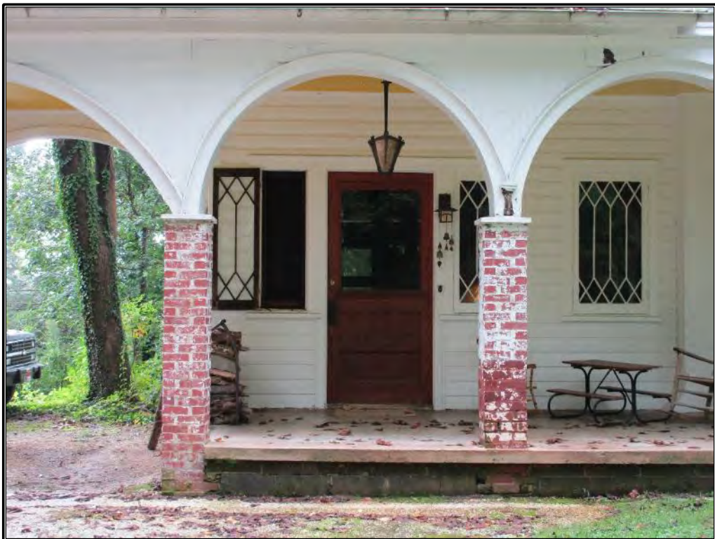
Figure 280. Detail of the arcade with the porte cochère to the left and the concrete porch with foyer entry to the center and right.
