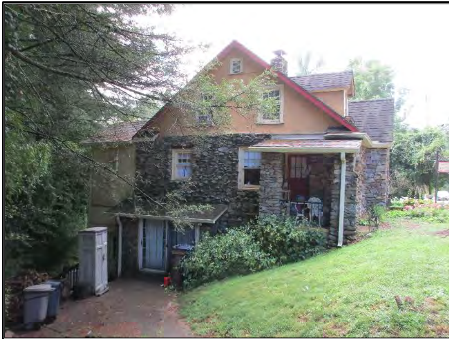
Figure 267. View of northern elevation.
