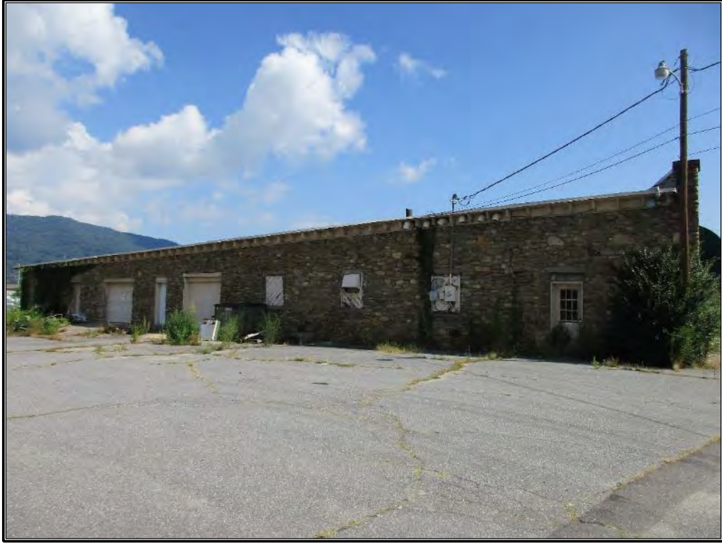
Figure 33. Southwest elevation of commercial building, looking north-northeast.
