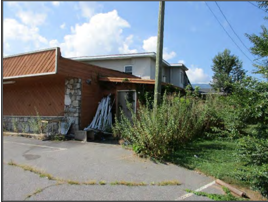
Figure 40. Northeast and rear elevation of secondary commercial building, looking south.
