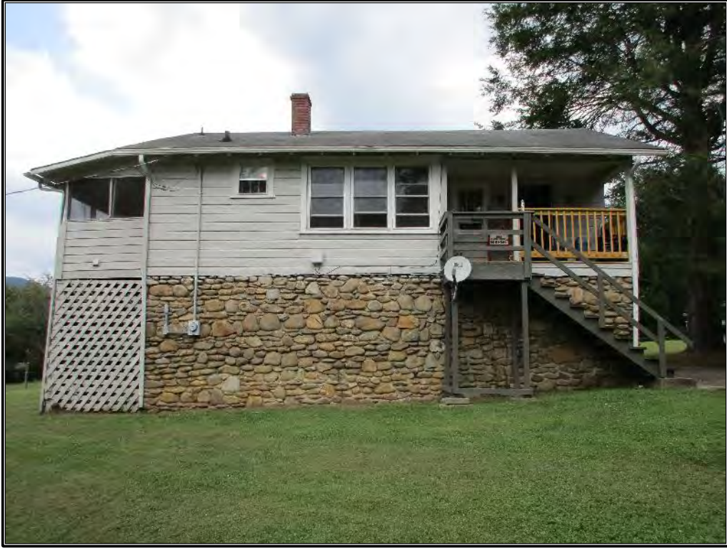
Figure 151. Façade of carriage house, looking north-northeast.
