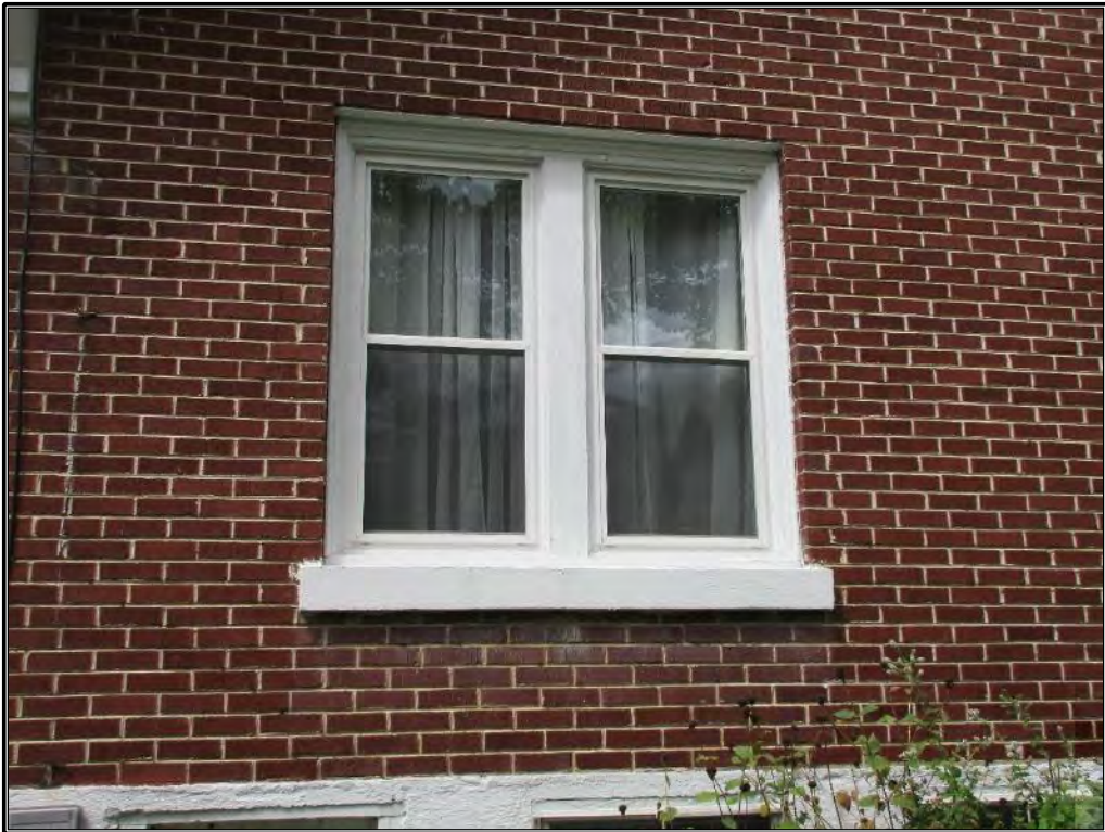
Figure 120. Detail of windows.
