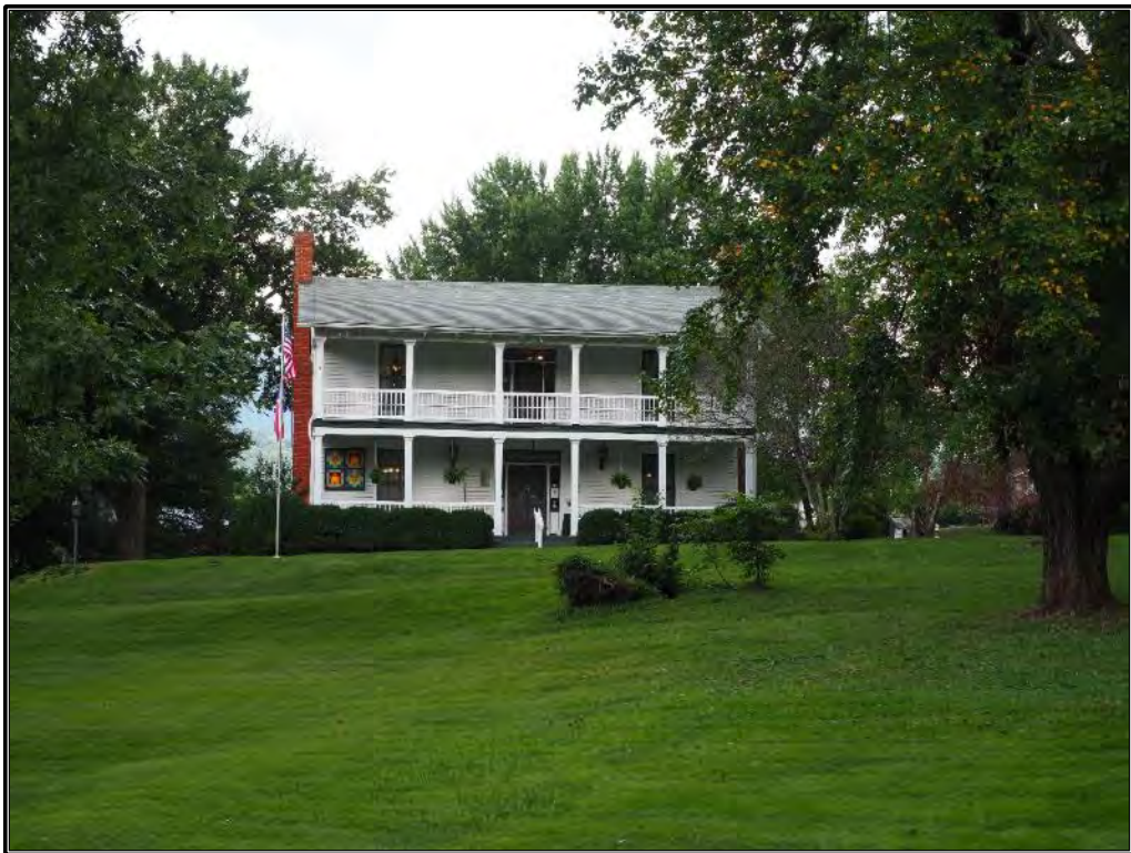
Figure 343. Façade view of the Shelton House (HW0003) on Pigeon Road, Waynesville.
