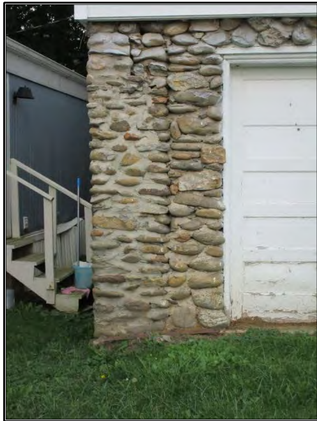
Figure 98. Detail of infilled pier foundation.
