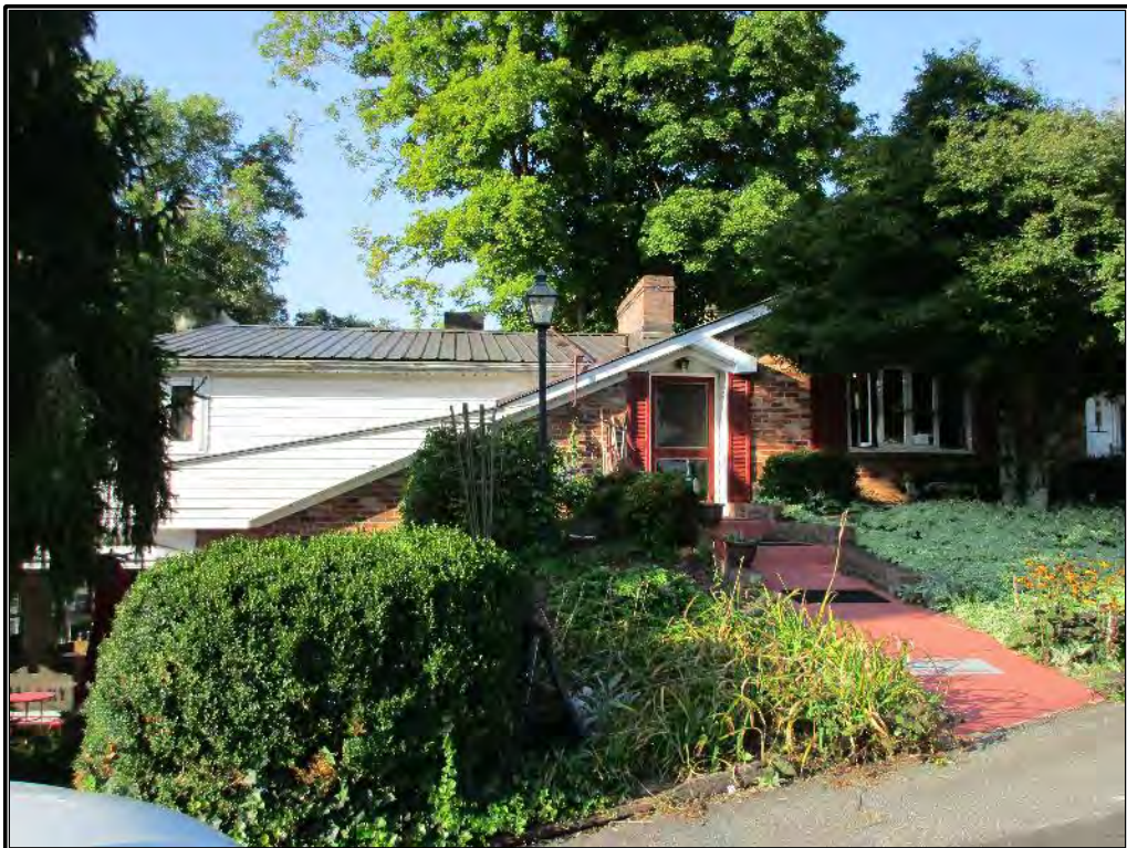
Figure 348. Walkway and entrance to the private innkeeper's quarters in Building A.
