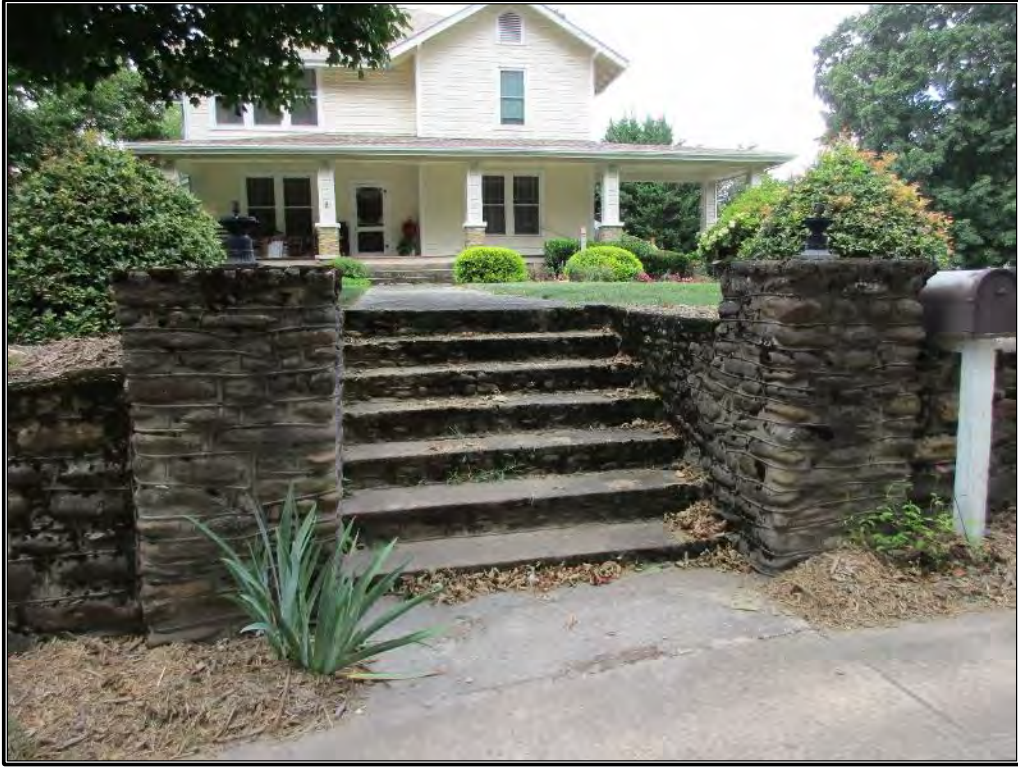
Figure 80. View of stone steps and gateposts and front walkway, looking north-northwest.
