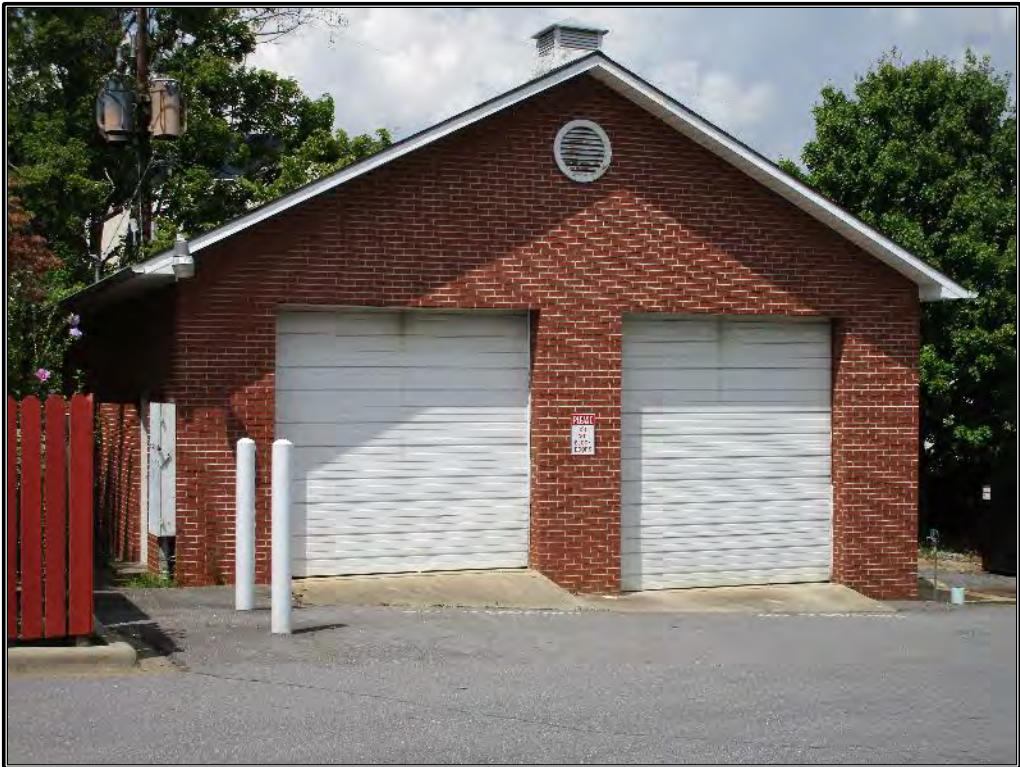
Figure 420. Eastern elevation of the garage.
